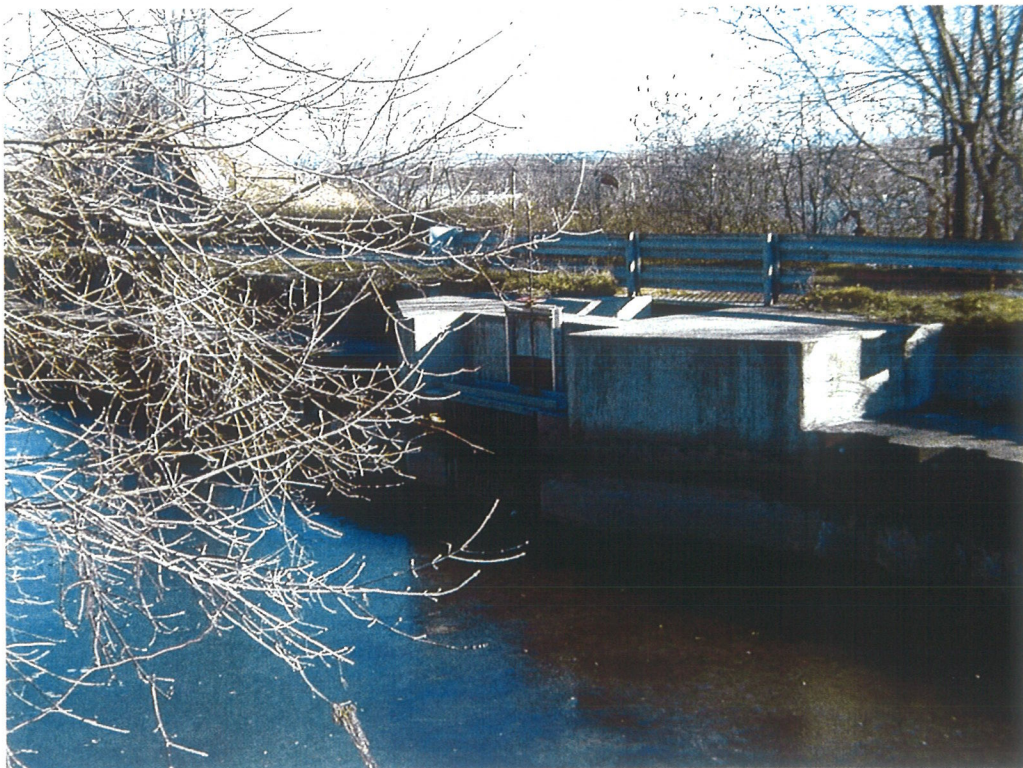
24. Gate from canal to Weir Brook (looking southeast).
