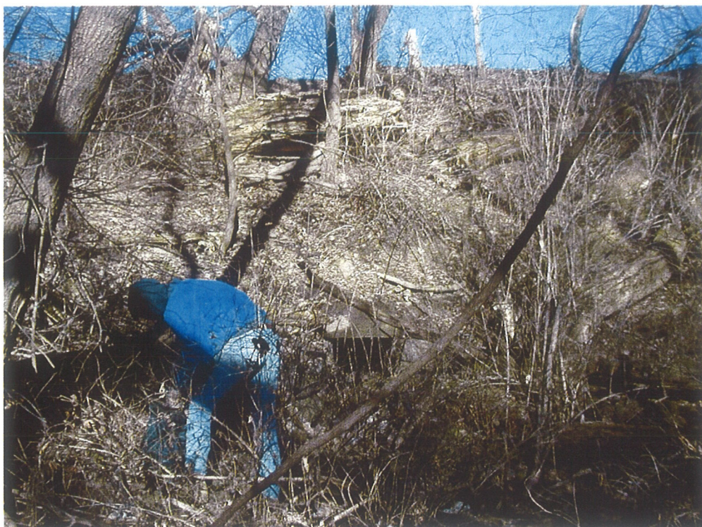
3. Stone culvert under canal by Northeast Lot (looking north).
