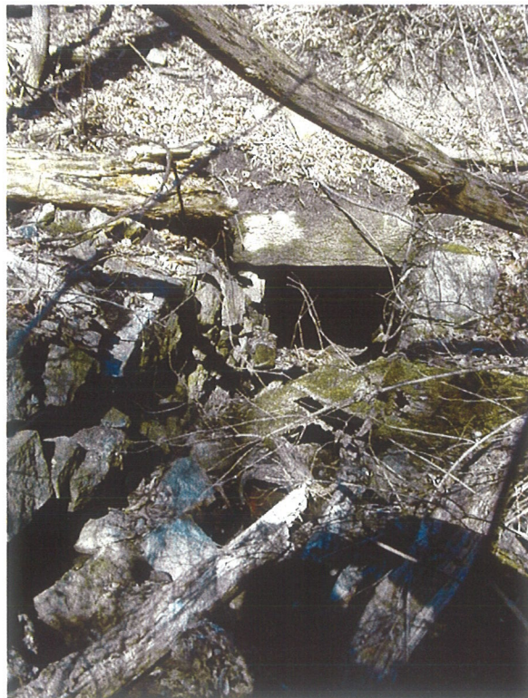
2. Stone culvert under canal by Northeast Lot (looking north).
