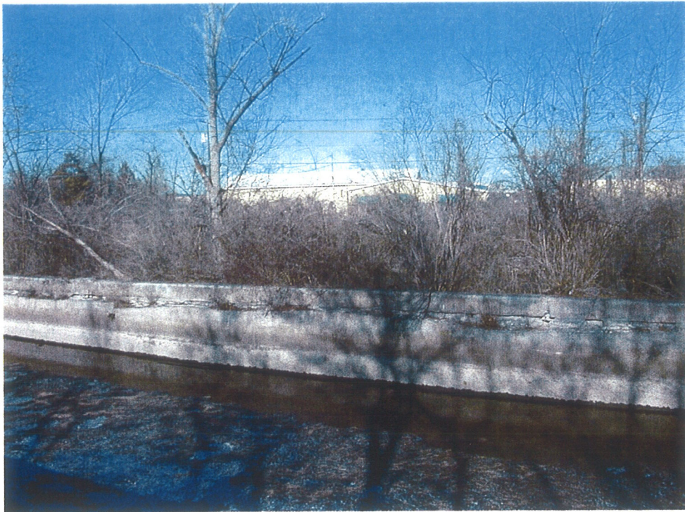
13. North wall of canal adjacent to Sliver Quarry (looking northwest).
