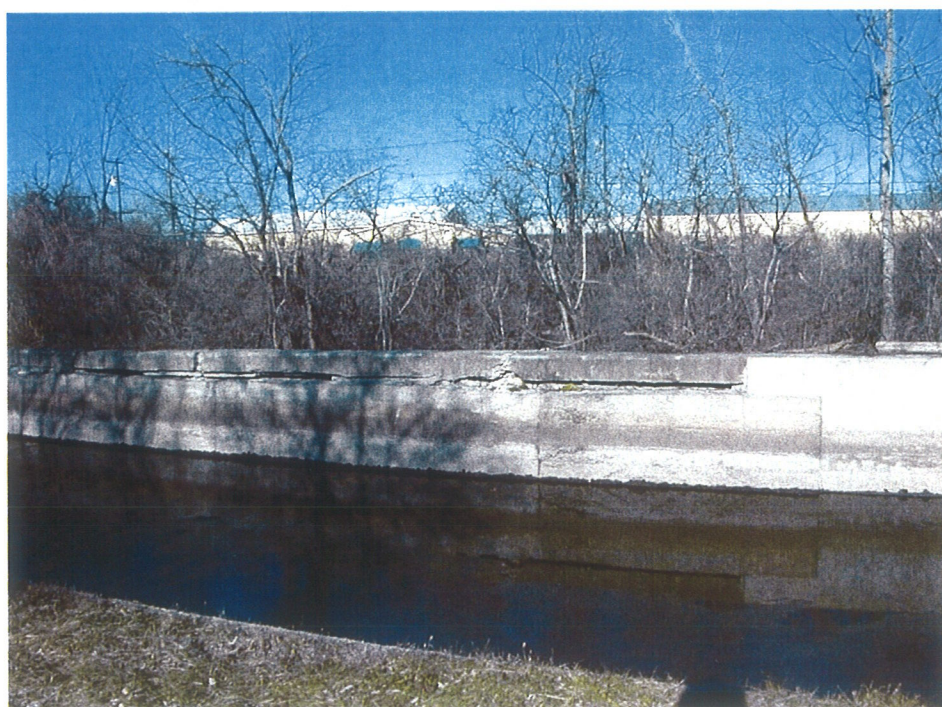
12. North wall of canal adjacent to Sliver Quarry (looking northwest).
