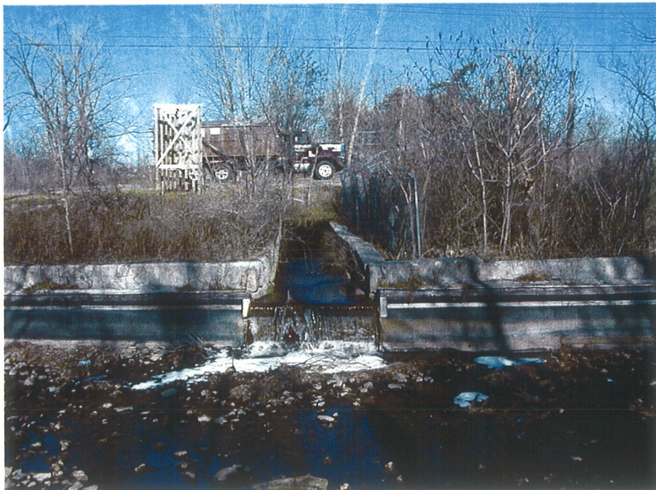
16. Sluice for stream entering canal from north (looking north). Sluice is directly west of Sliver Quarry.
