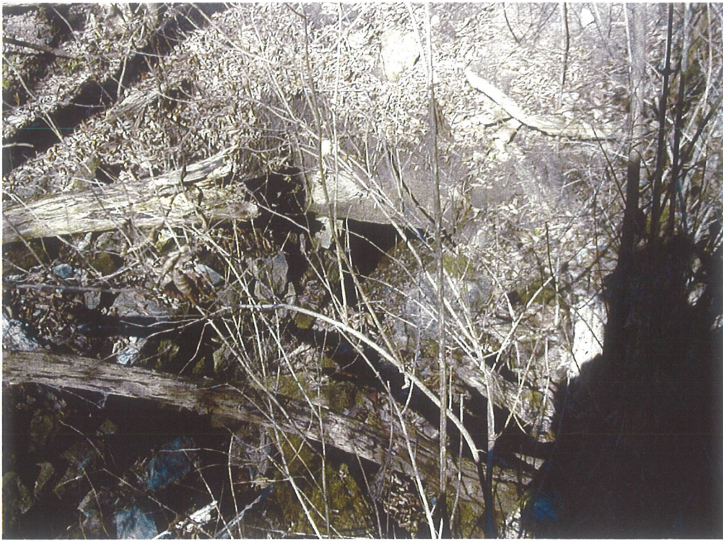
1. Stone culvert under canal by Northeast Lot (looking northeast).
