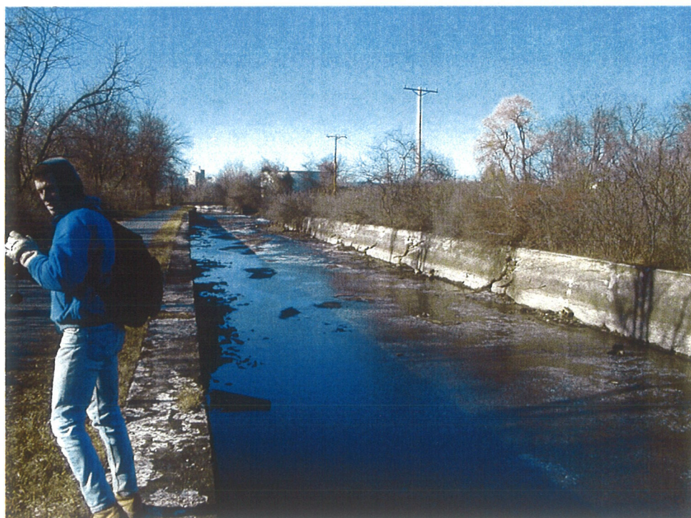
4. Canal east of Pretreatment Plant and north of Northeast Lot (looking west).
