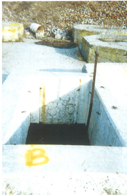
A6. Sump in concrete pad located directly west of former Building 53, designated as "Sump B".
