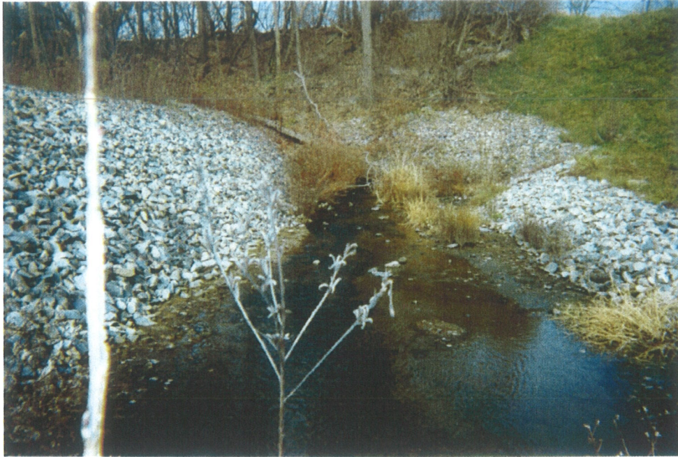
A1. Stream feeding Cement Company Pond (looking north) on 11/18/99, prior to opening of gate from canal to Weir Brook.
