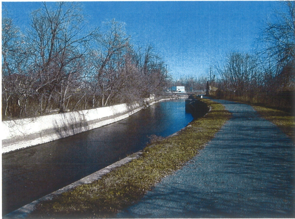
10. View of canal looking east from approximately 200 feet west of Weir Brook inlet gate. Gate structure is visible.
