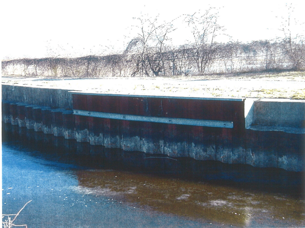
25. Repair to south wall of canal with tie-backs east of Weir Brook gate (looking southeast).
