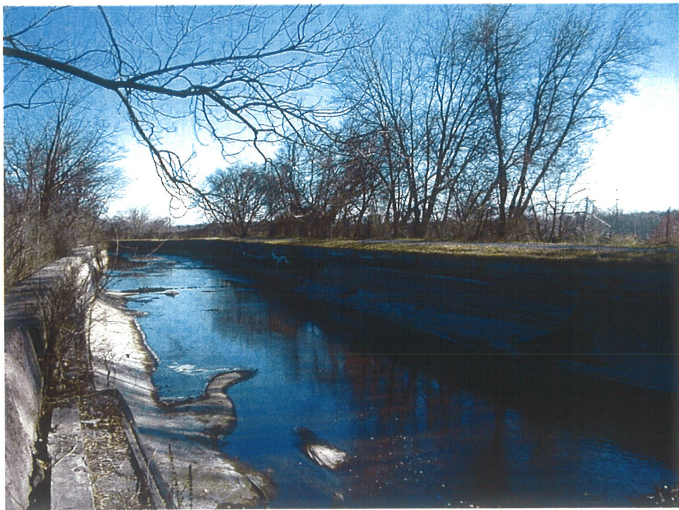
18. View of canal to east from canal wall near west end of Sliver Quarry (near sluice).
