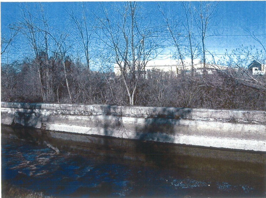
14. North wall of canal adjacent to Sliver Quarry (looking northwest).
