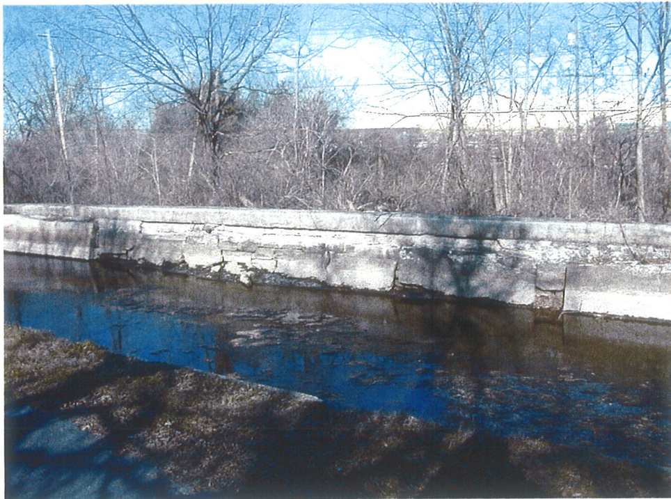
15. North wall of canal adjacent to Sliver Quarry (looking northwest).
