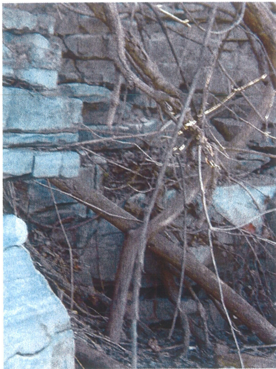
23. Rock cove in south wall of Sliver Quarry by flow outlet area.
