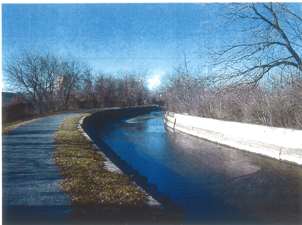
11. View of canal looking west from approximately 200 feet west of Weir Brook inlet gate.
