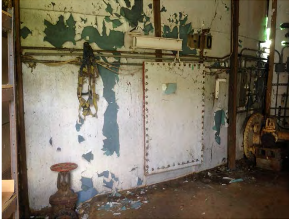
Photo 3 Tank-110 access port and drain valve in PTP building
