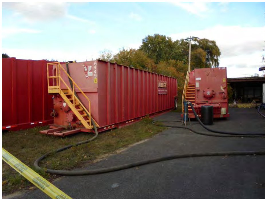
Photo 21 On-site frac tanks for water storage
