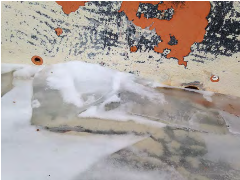
Photo 33 Holes drilled in AST walls on NW side
