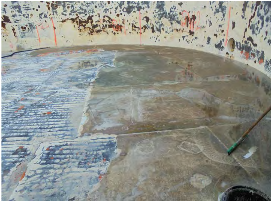
Photo 10 Tank-110 floor (left side of photo after initial clean, right side not cleaned)
