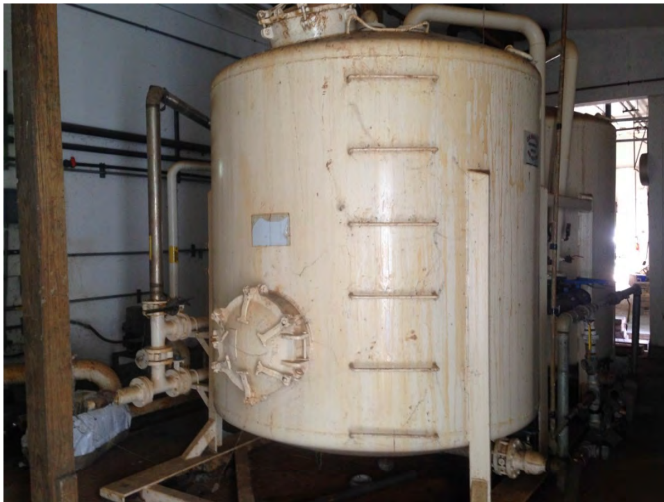
Photo 4 Skid mounted sand vessels in PTP
