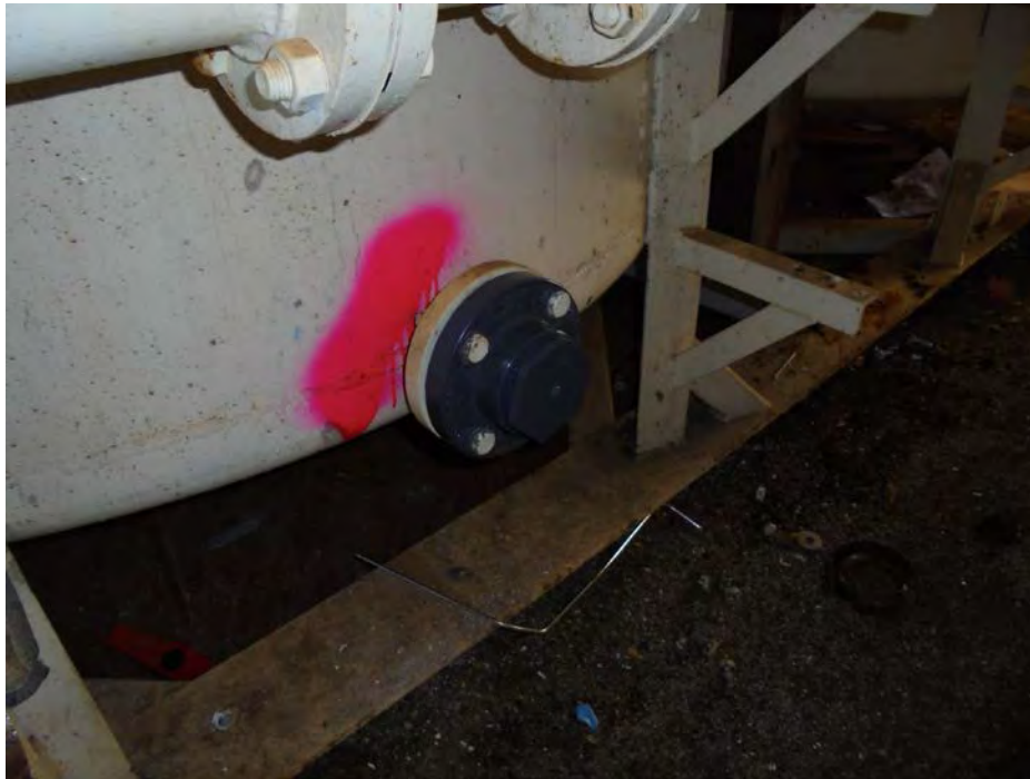
Photo 18 Blanked outlet on south side vessels
