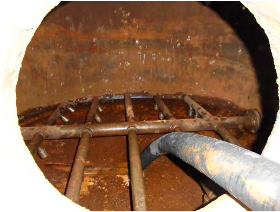
Photo 16 Vessel interior prior to cleaning
