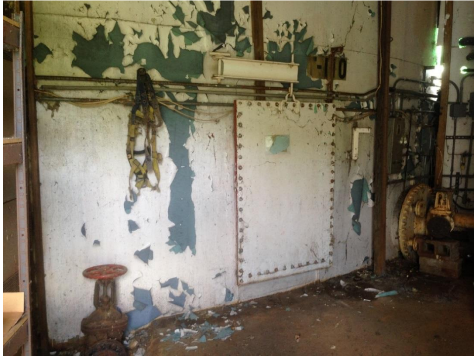
Photo 3: 500,000.gallon AST access port and drain valve in PTP building.
