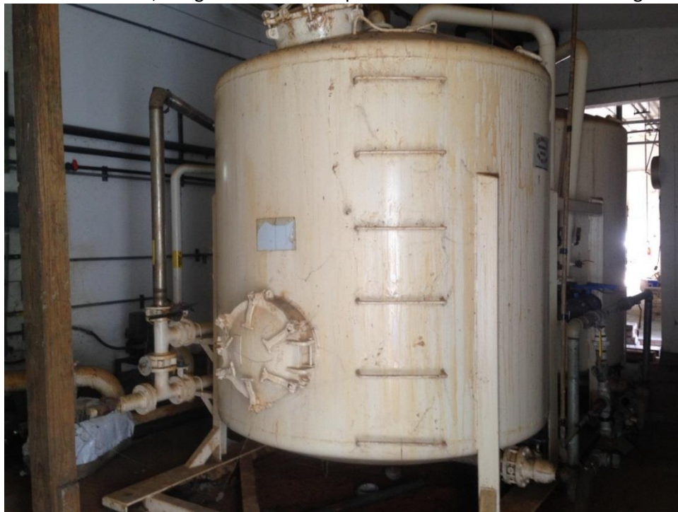
Photo 4: Skid mounted sand vessels in PTP.
