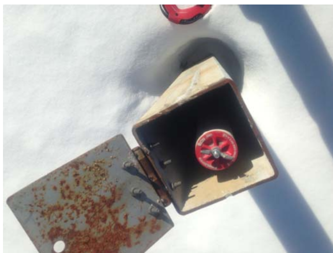
Typical down well view (at MW-7)
