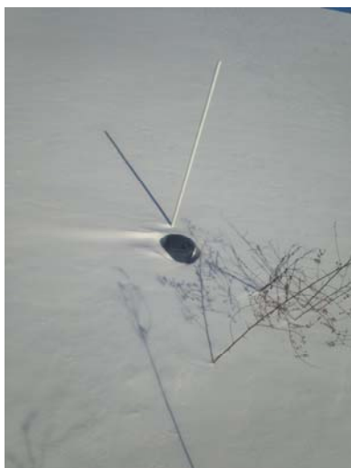
W-4 to leachate system pipe cleanout
