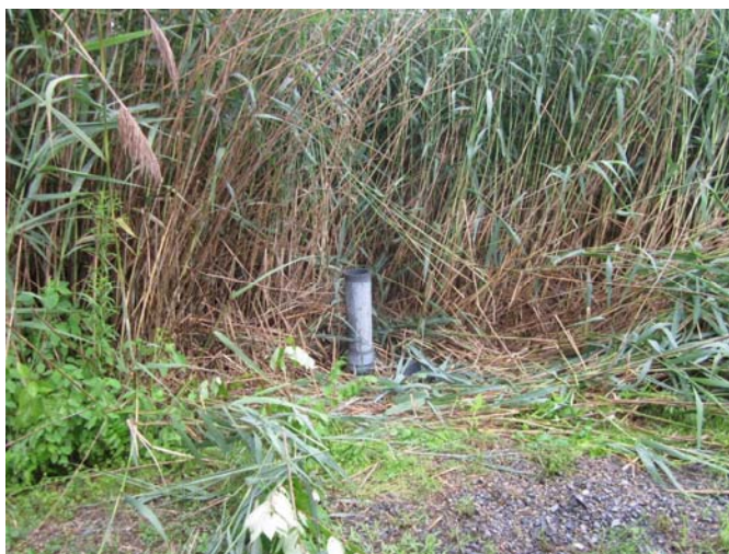
Typical CWTS cell cleanout
