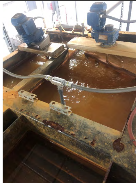
Top view of IPC Flocculant chamber.
