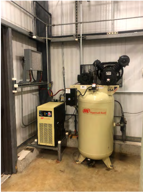
View of current Air Compressor setup.
