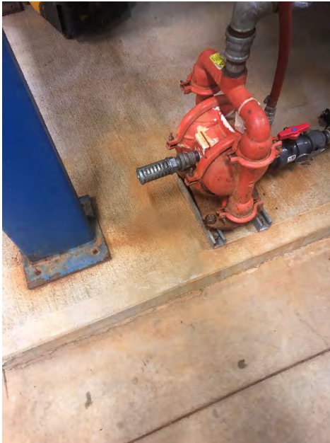
View of Inclined Plate Clarifier transfer pump.
