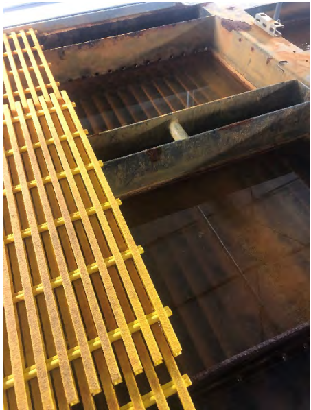
Partial top view of Inclined Plane Clarifier prior to washdown.
