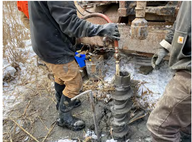
Parratt-Wolff abandoning SB-12C with grout/bentonite mix.
