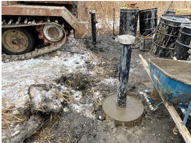
Poured concrete pad for MW-12B.
