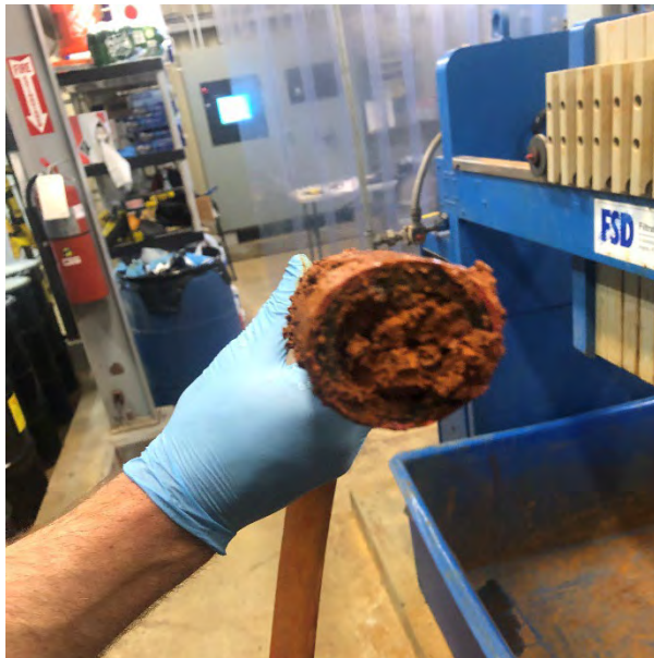
View of EW-4 transfer piping clogged with sludge.
