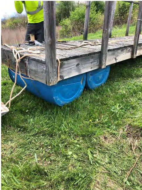
View of Polishing Pond dock following replacement of drums.
