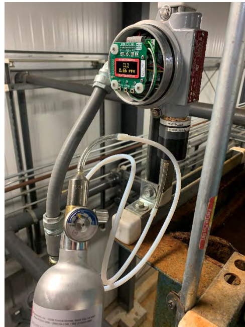
View of chlorine sensor calibration.
