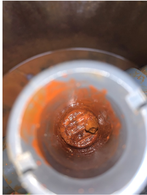
View of scaling within EW-3 flowmeter piping tee.
