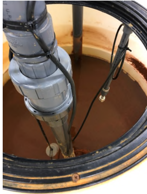
View inside of clarifier catch tank.
