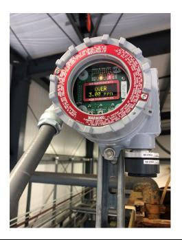
View of chlorine sensor located within Treatment System building.
