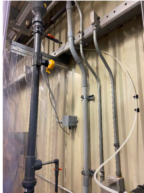
View of bleach pump transfer tubing.
