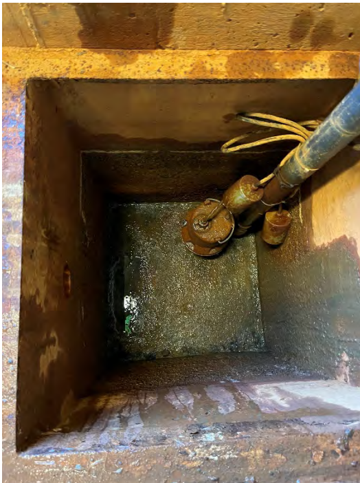
View of Old Sump after cleaning.
