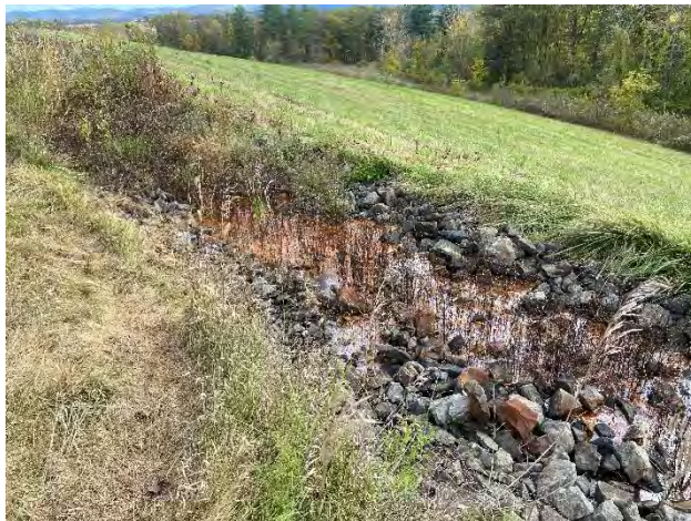
View of ponding water in Southern mid-cap swale.
