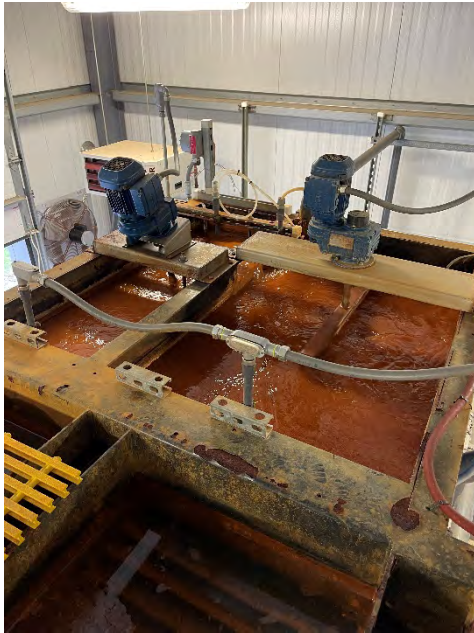
View of Inclined Plate Clarifier (IPC) mixing chambers.
