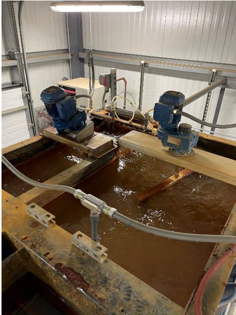
View of influent IPC mixing chambers.
