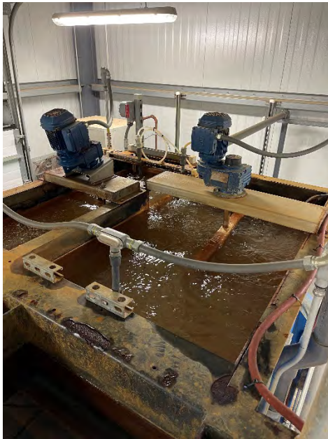
View of IPC mixing chambers.
