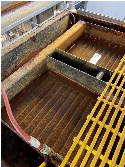
View of IPC plates before cleaning.
