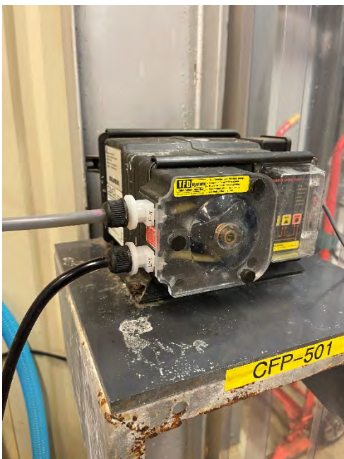
View of Sodium Permanganate pump.
