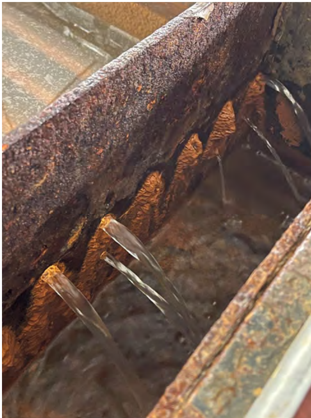
View of sludge build-up on IPC prior to spray down.
