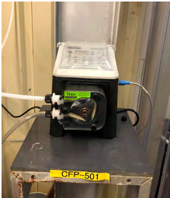
View of newly installed sodium permanganate pump.
