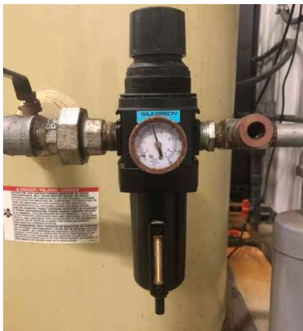
View of air compressor regulator after repair.
