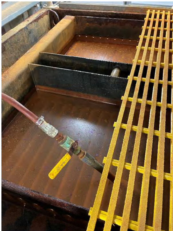
View of IPC plates prior to cleaning.
