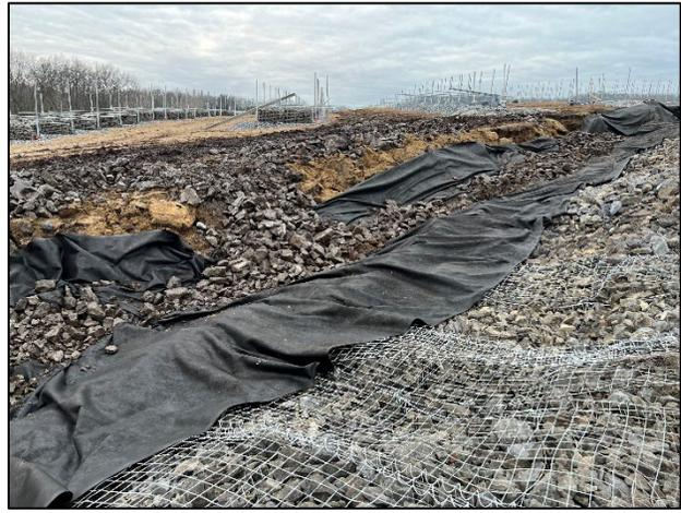
10. Placement of rip-rap stone onto geotextile within temporary swale.
