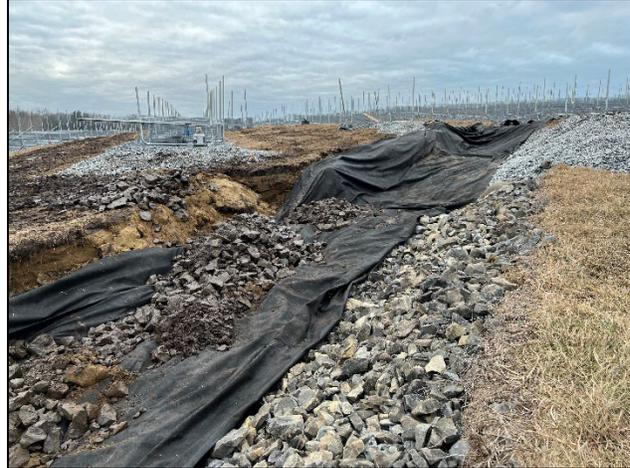
12. Placement of rip-rap stone into temporary swale.
