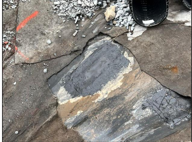
6. Temporary repairs made to HDPE geomembrane liner.
