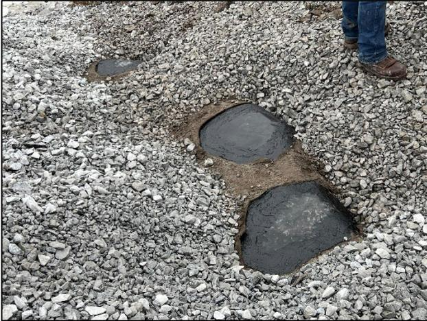
7. Temporary repairs made to HDPE geomembrane liner.
