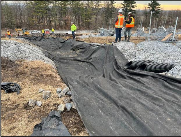
9. Geotextile fabric placed in down-chute swale.
