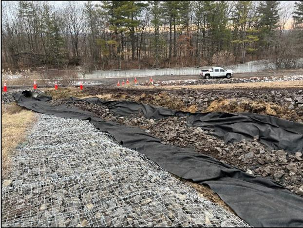
11. Placement of rip-rap stone into temporary swale.
