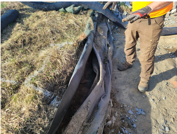
Swale with Dummy Layer
