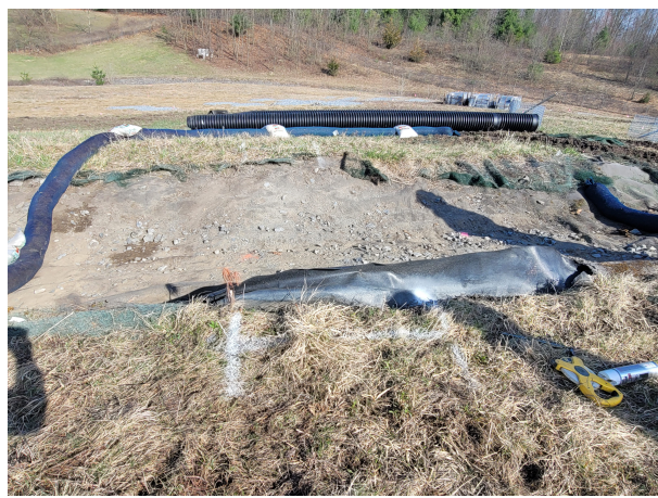
Silt Sock Install
