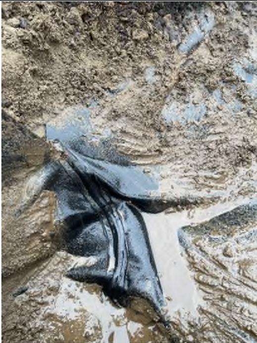
13. Fusion weld of swale liner near Test Pit #2.
