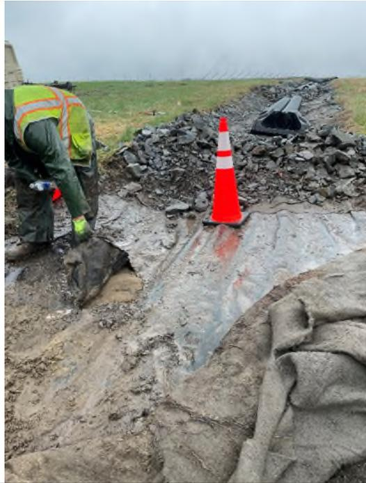
12. Damaged swale Liner at sediment upwelling area - Test Pit #2 Area looking southwest.
