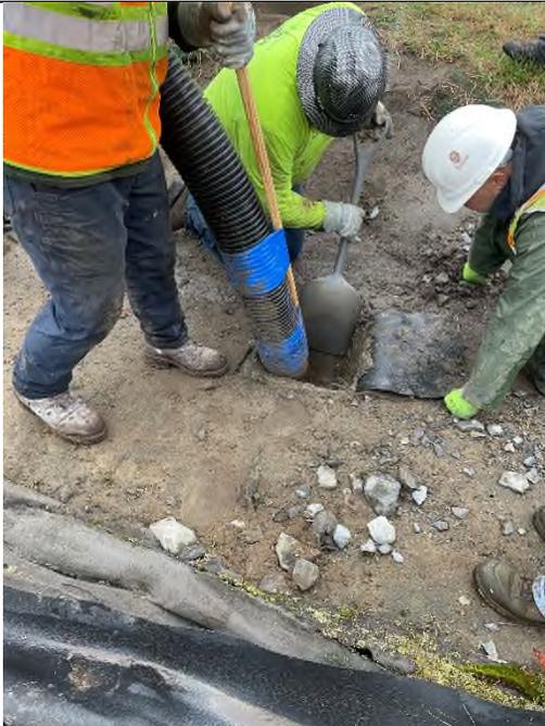
Crew working to expose cap liner in center of swale through access hole cut in liner at Test Pit #1B.
