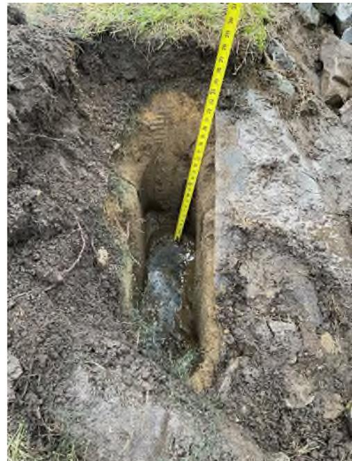
6. Cap Liner found at 18" at edge of swale – Test Pit #2A.
