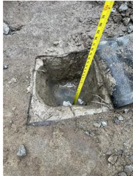
Landfill Cap Liner found at 14" below swale liner at Test Pit #1B.
