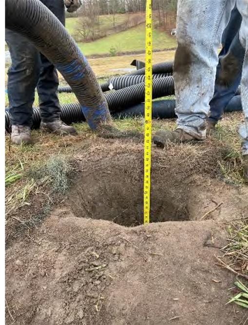
16. Landfill Cap Liner Found at 38" below edge of swale – Test Pit #1A.
