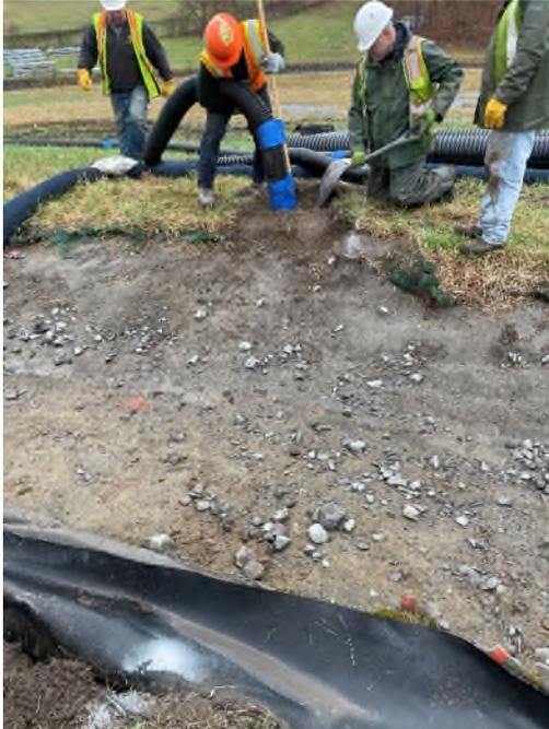
15. Crew working to expose cap liner at Test Pit #1A. Facing northwest.
