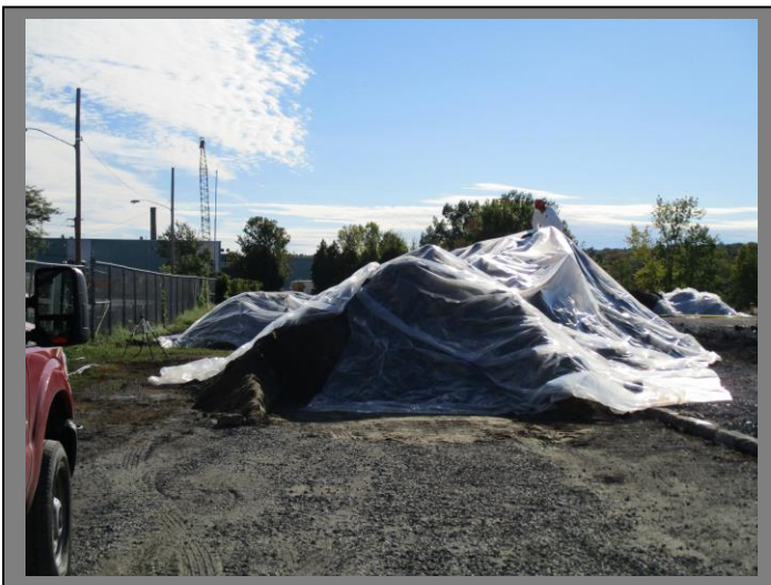
Example of covered stockpiles during deconstruction.
