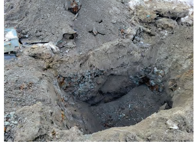
Photo 70: Completed excavation at the TP-118 location, facing south.
