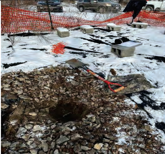
Photo 51: Excavation with handheld equipment at the TP-113 location, facing west.
