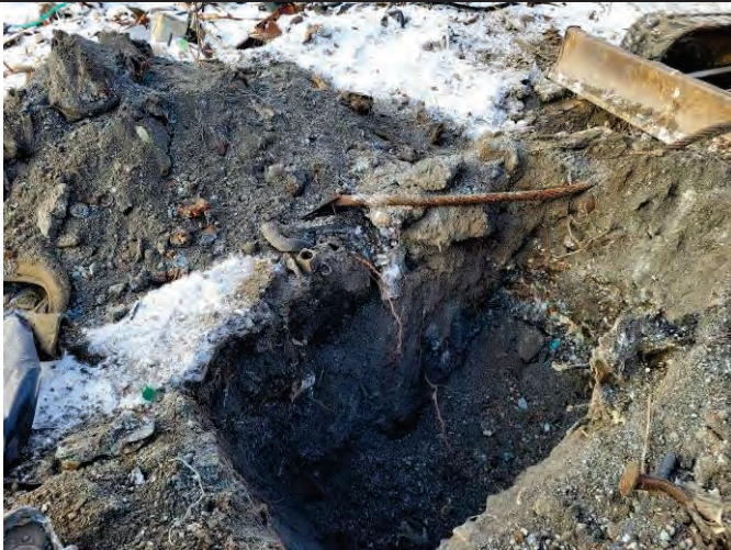
Photo 83: The completed excavation at the TP-123 location, facing southeast.
