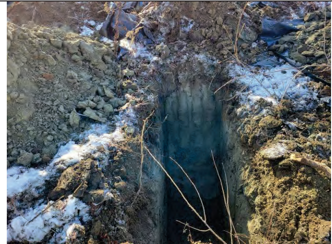
Photo 72: Sidewall at the TP-119 location, facing south.
