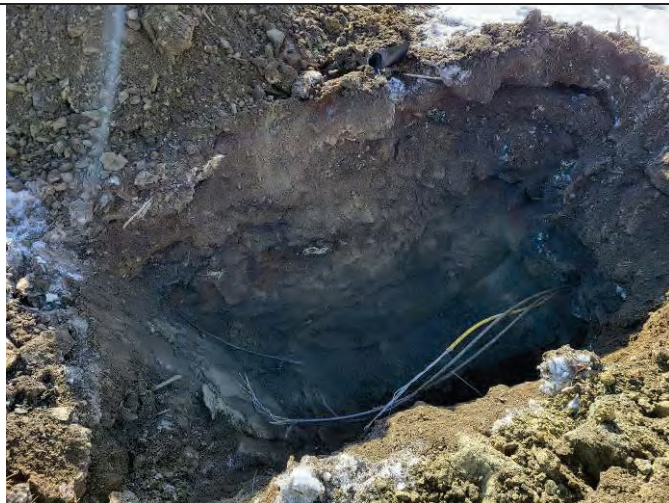
Photo 75: The completed excavation/sidewalls from the TP-120 location, facing southwest.
