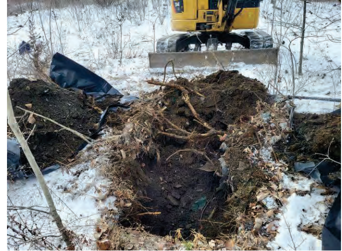
Photo 14: TP-103 excavation/test pit, facing south.
