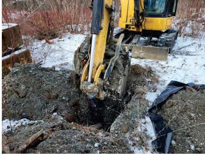
Photo 49: Excavation activities at the TP-112 excavation location, facing west.
