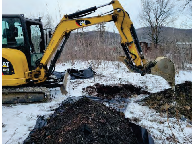
Photo 1: Excavation activities at the TP-101 location, facing west.
