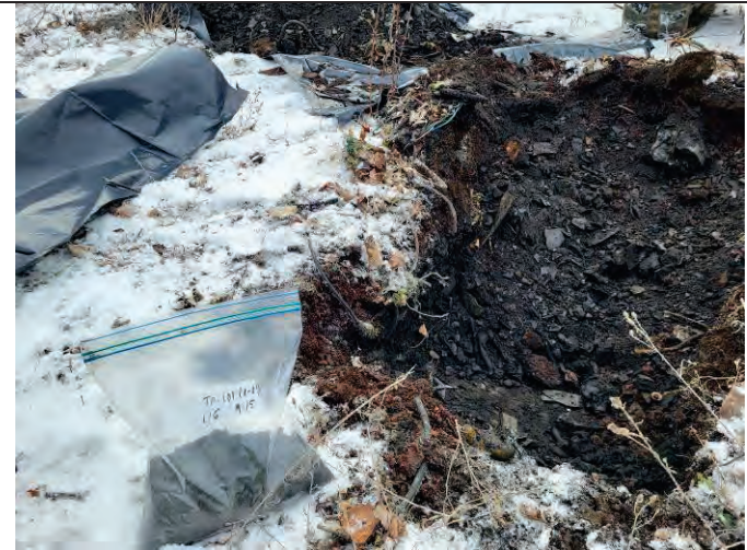
Photo 4: Sidewall of TP-101, facing north.
