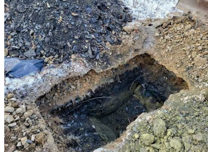
Photo 34: The completed TP-108 test pit excavation, facing west.
