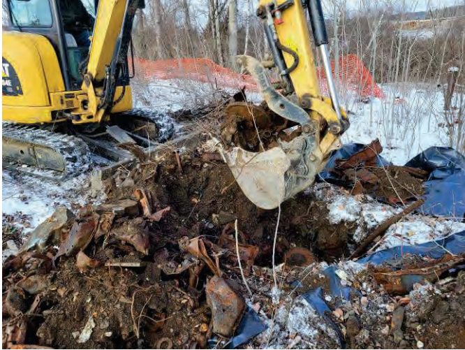
Photo 45: Excavation activities from the TP-111 location, facing north.
