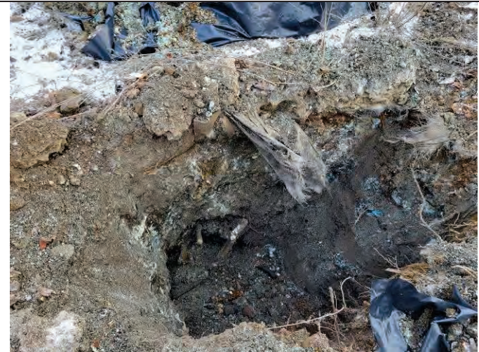
Photo 48: Sidewalls at the TP-112 test pit location, facing northwest.
