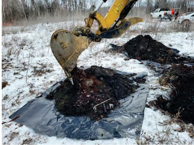
Photo 5: Excavation activities at the TP-101 location using a mini-CAT excavator, facing southwest.
