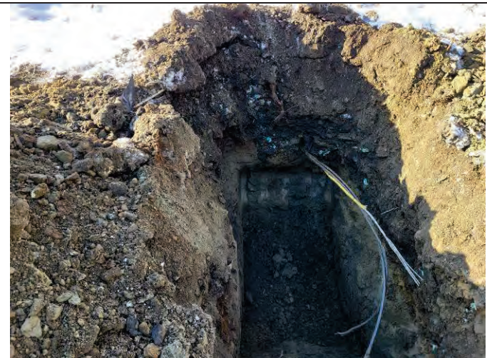
Photo 76: The sidewall at the TP-120 location, facing west.
