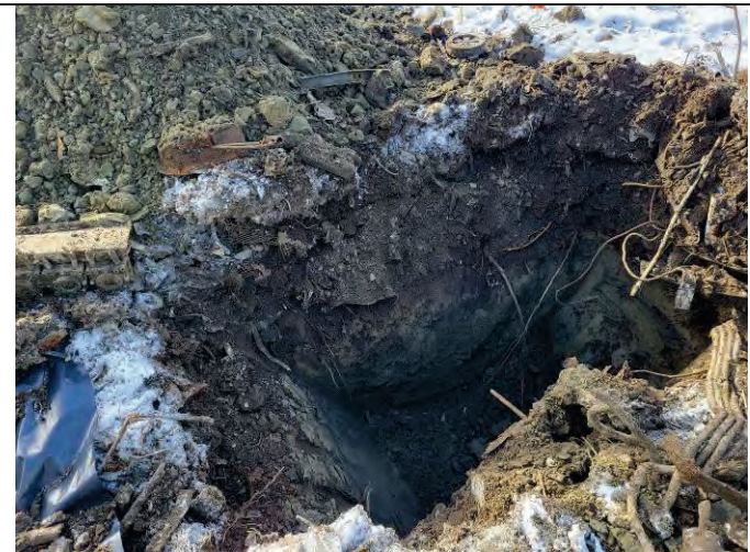
Photo 64: Sidewall at the TP-117 location, facing east.
