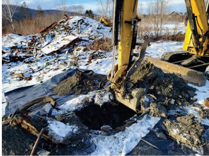
Photo 89: Excavation activities at the TP-124 location, facing south.
