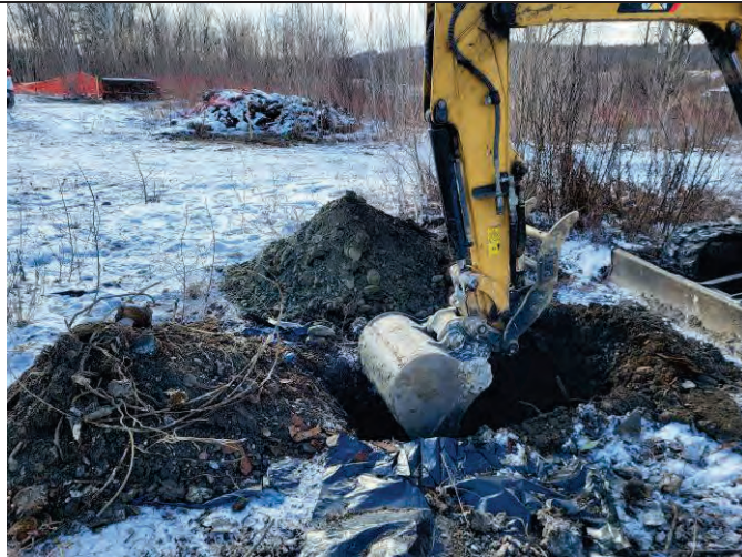
Photo 15: Excavation activities at the TP-103 location, facing east.
