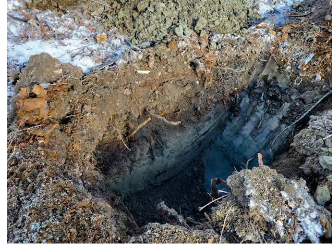
Photo 18: The TP-104 southern facing sidewall.
