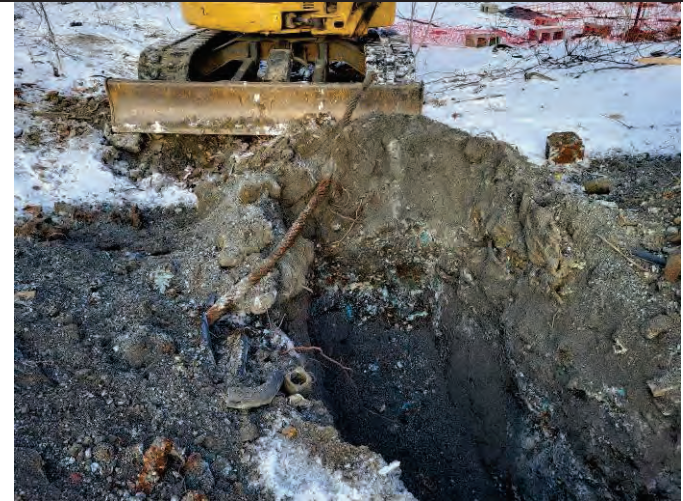
Photo 84: The sidewalls at the TP-123 location, facing south.
