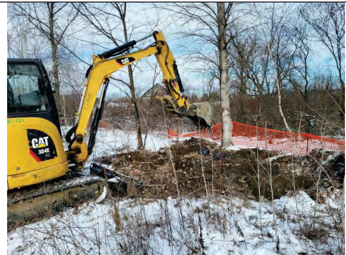
Photo 24: TP-106 excavation location, facing northeast.
