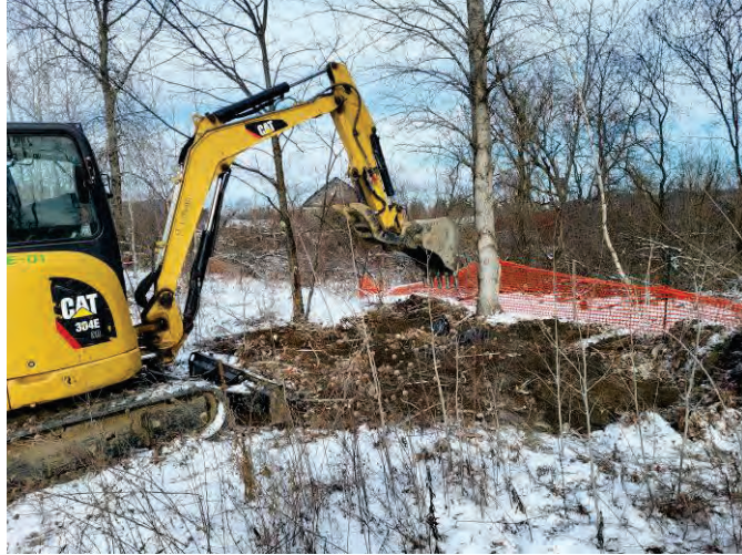
Photo 85: Excavation activities at the TP-124 location, facing north.
