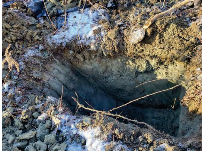
Photo 73: Completed excavation at the TP-119 location, facing west.
