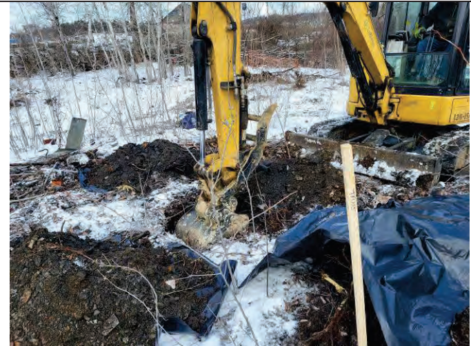
Photo 20: Excavation activities at the TP-105 location, facing north.
