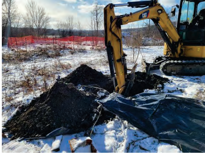
Photo 77: Excavation activities at the TP-120 test pit location. Facing southwest.
