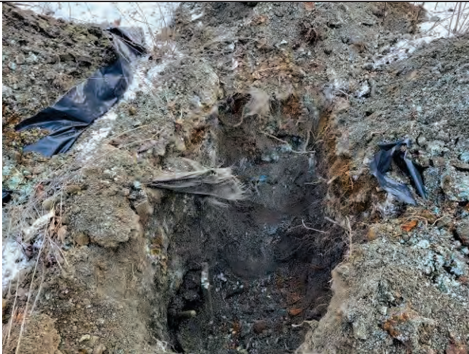
Photo 47: Sidewalls at the TP-112 test pit excavation location, facing west.
