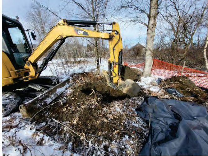
Photo 41: Excavation activities at the TP-110 location, facing north.
