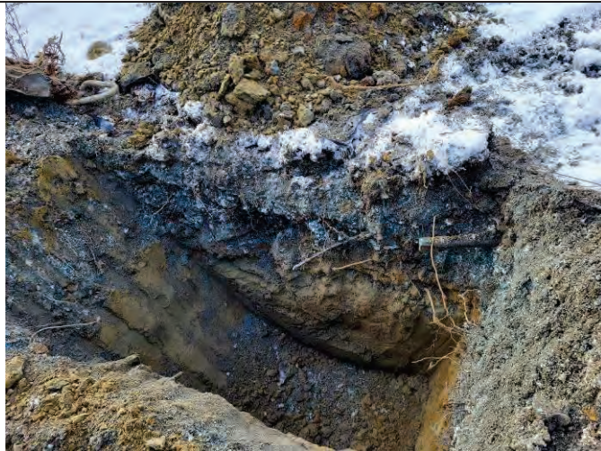
Photo 87: The completed TP-124 excavation, facing north.
