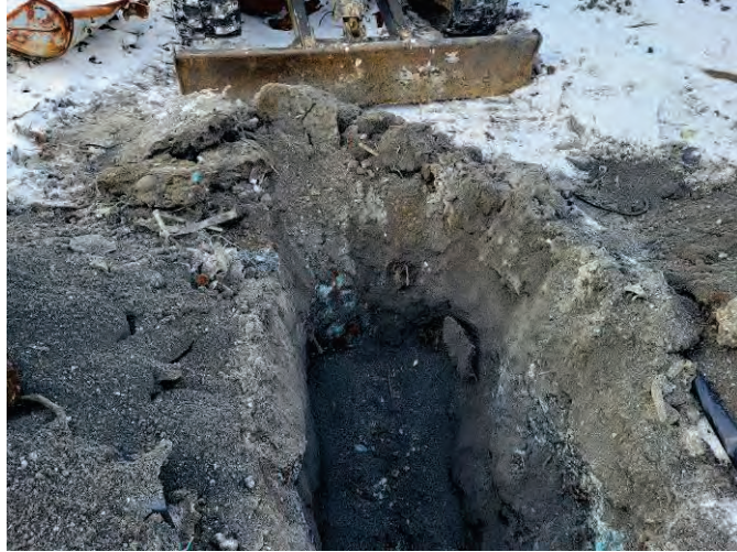
Photo 69: The sidewall at the TP-118 location, facing west.
