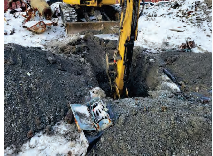
Photo 66: Excavation activities at the TP-117 location, facing north.
