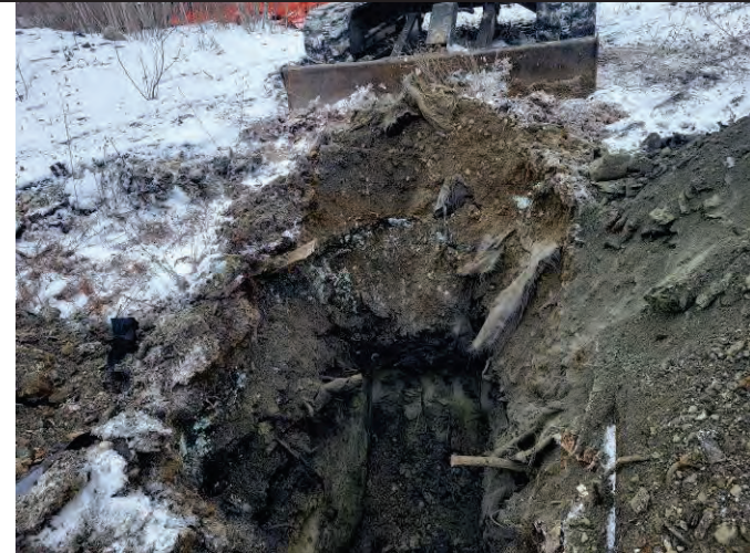
Photo 52: Test pit excavation activities at the TP-115 location, facing west.
