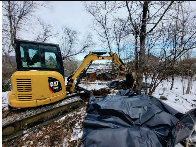
Photo 7: TP-102 excavation location, facing north.
