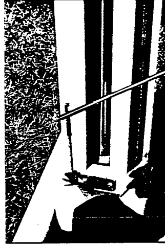
Figure 4.17. Extension Rods are attached to the MC Piston Release Rod using Extension Rod Quick Links.
