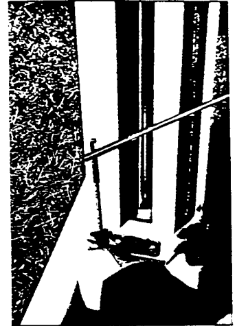
Figure 4.33. Using Extension Rod Quick Links to connect Extension Rods.
