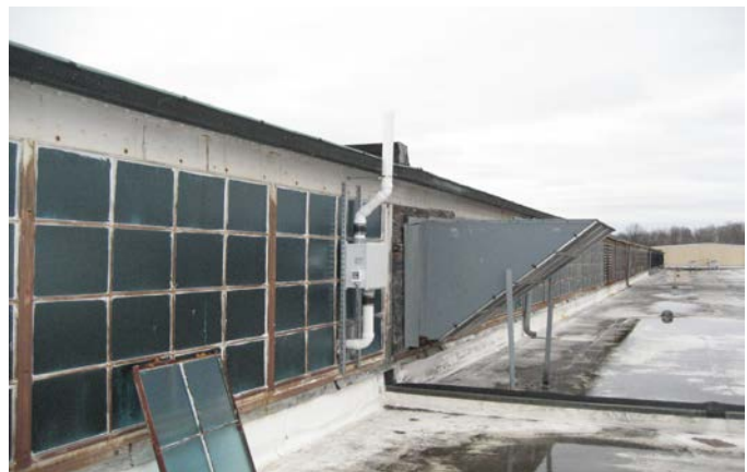
Typical SSDS fan mounted to the upper monitor windows of the 2200 Bleecker Street building.
