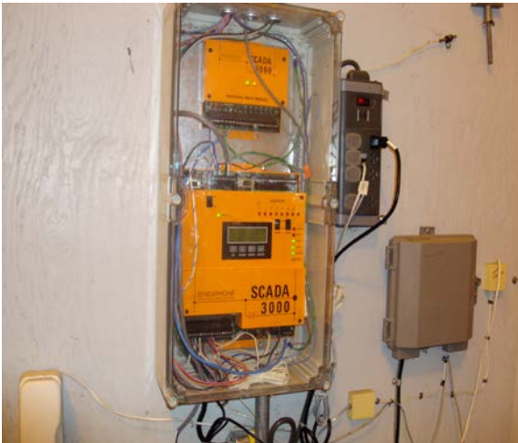
View of the SCADA 3000 auto-dialer from inside the RAF building.
