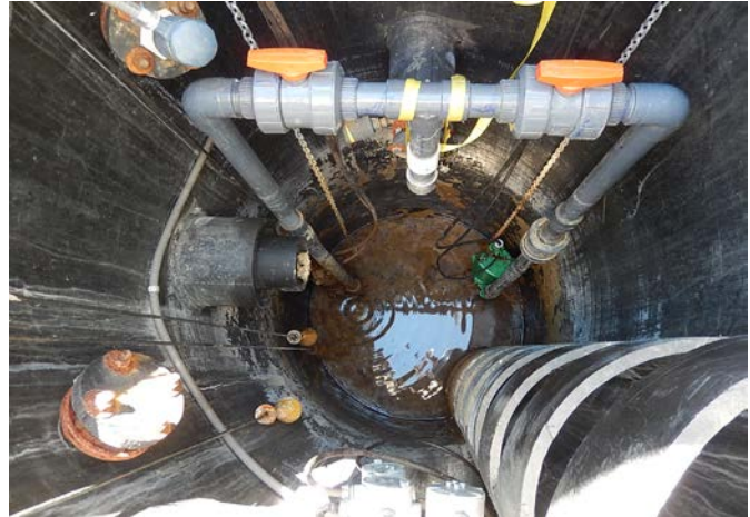
View of the leachate collection manhole with new lead pump installed.
