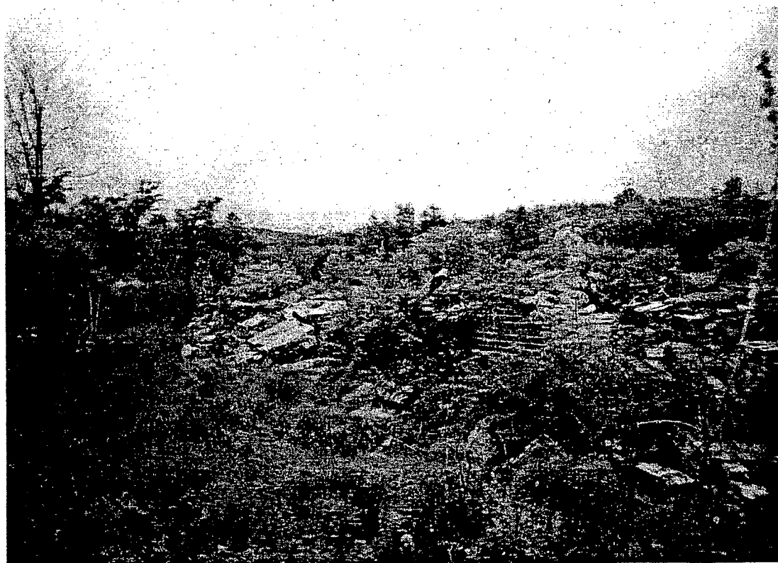
Plate 4. Extant wall segments and demolition rubble along the southern perimeter of the tannery foundation; view south.
