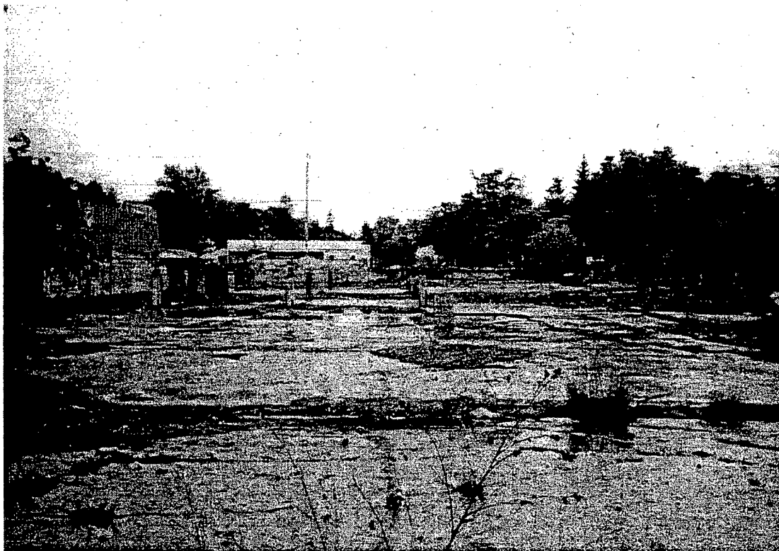
Plate 1. Concrete foundation floor of the former Hiteman Leather Tannery, from the northwest corner; view east.
