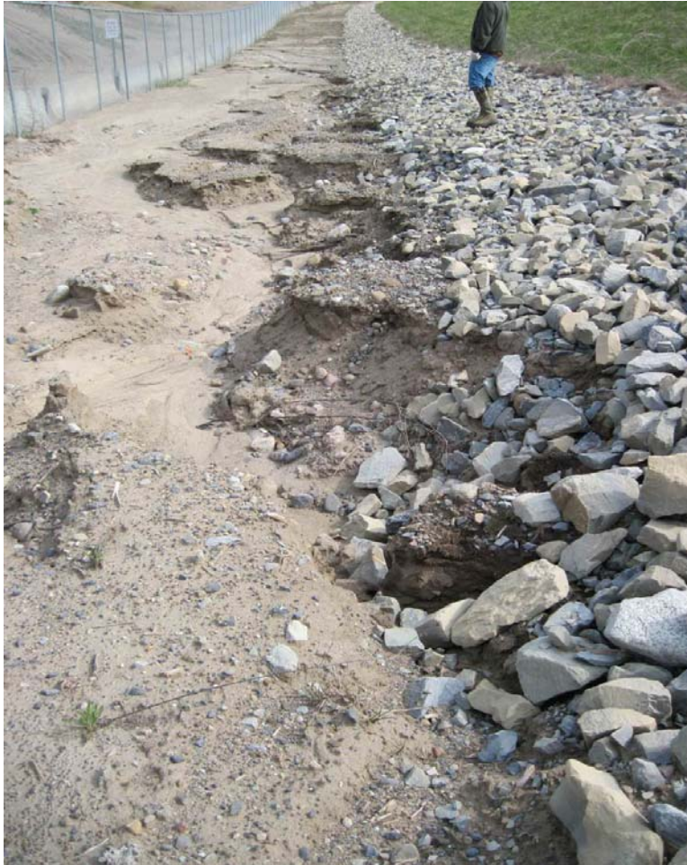
Photo 17: Close up of erosion along west side of landfill. Erosion at toe drain interface has resulted in undermining of stone channel.
