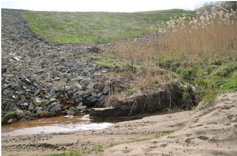
Photo 9: Inlet of North Detention Pond. Sediment in basin. Erosion occurring outside drainage channel.
