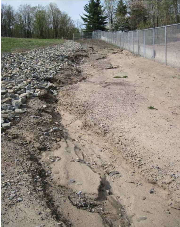
Photo 18: Erosion along west side of landfill looking south. Erosion has occurred at toe drain/channel interface.
