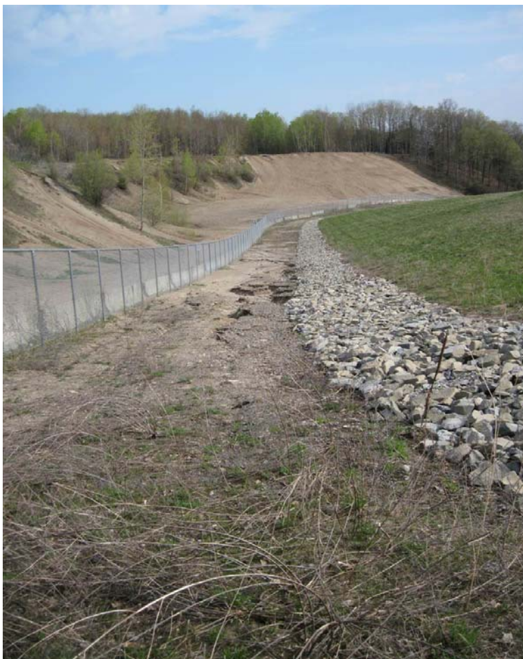
Photo 16: Erosion along west side of landfill looking north.
