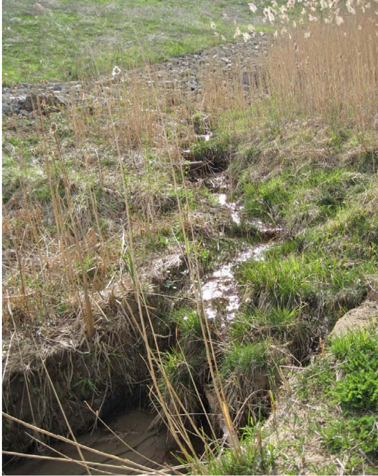
Photo 8: Eroded area leading into North Detention Pond. Note – Erosion is occurring outside drainage channel.
