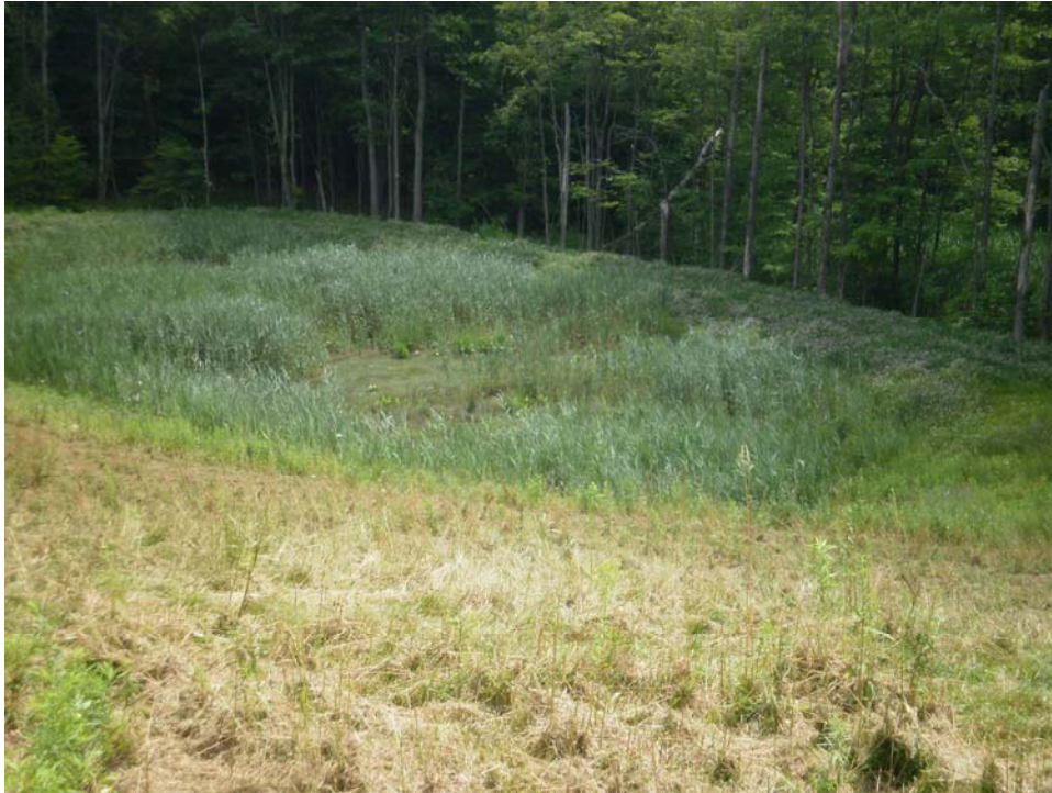
Photo 7: 7/12/2011-South Detention Pond with sediment accumulation.
