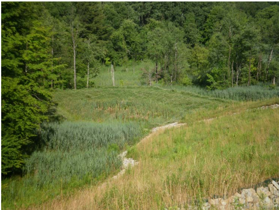
Photo 8: 7/12/2011-North Detention Pond with sediment accumulation.
