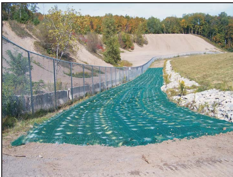
Photo Date 09-23-10. North view of newly installed erosion matt. Approximate dimensions are 310' long x 18' wide.
