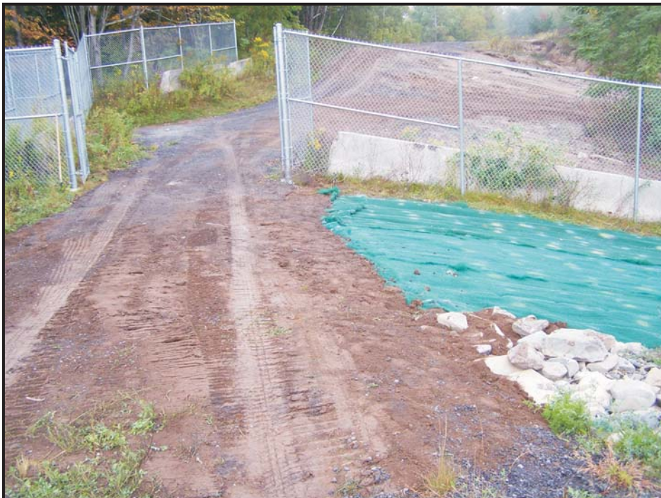
Photo Date 09-23-10. Looking west, site access gate and newly installed erosion matt pinned into soil.
