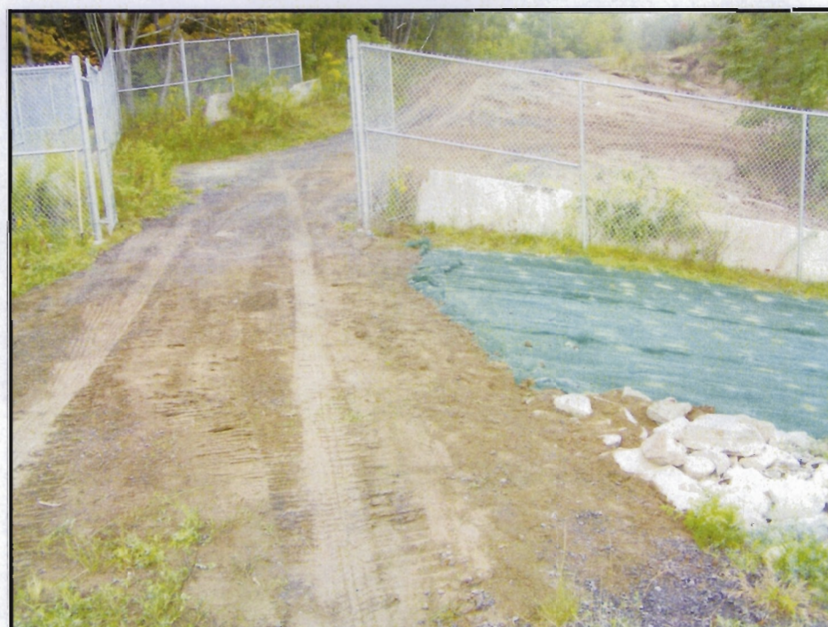
Photo Date 09-23-10. Looking west, site access gate and newly installed erosion mat pinned into soil.
