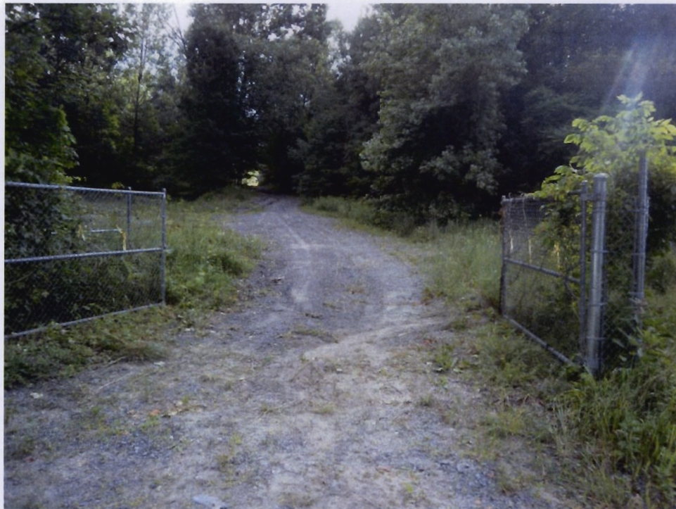
Photo 2: 7/12/2011-Erosion/rilling in access road (upper center of photograph) has reached underlying geotextile fabric and is up to 1 foot across and up to 1 foot deep. Note hogweed growing to right side of gate.
