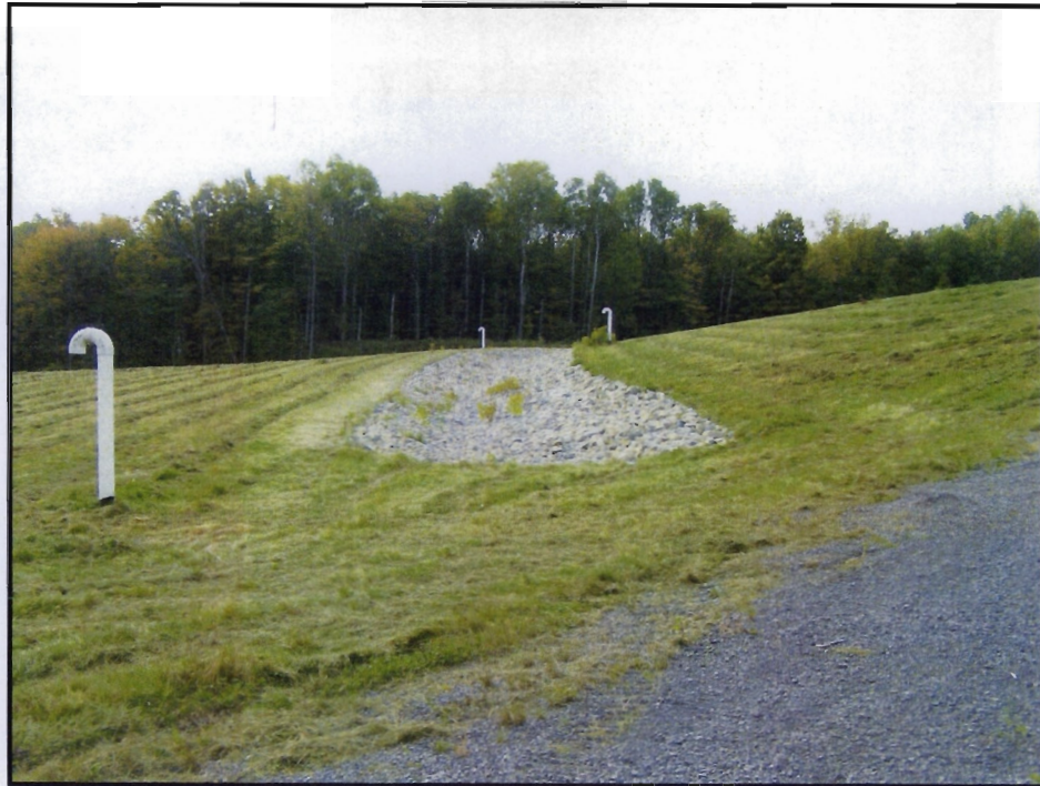
Photo Date 09-23-10. South view of mowed landfill.
