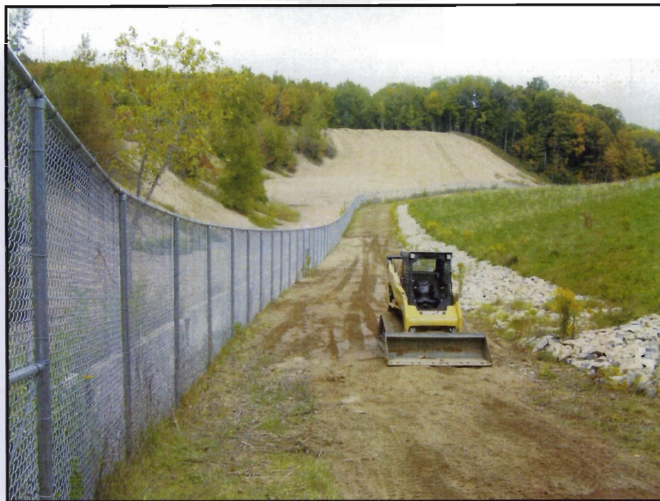
Photo Date 09-22-10. Looking north, skid steer being used to backfill and grade erosion swales.
