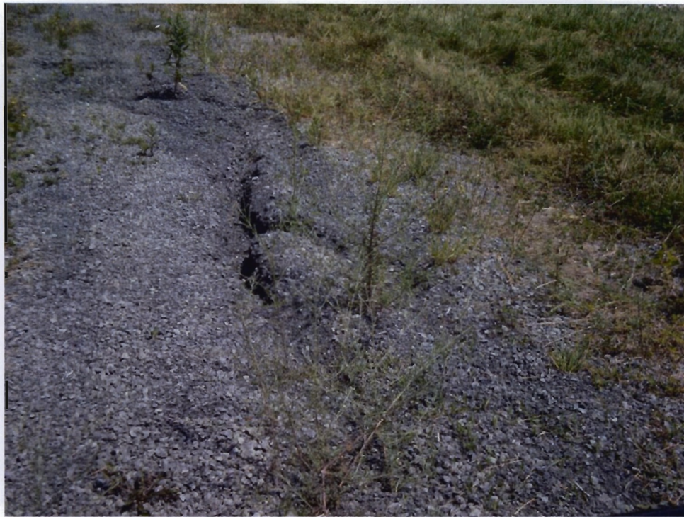
Photo 15: 7/13/2011-Rilling on gravel access road which is on top of the landfill cap.
