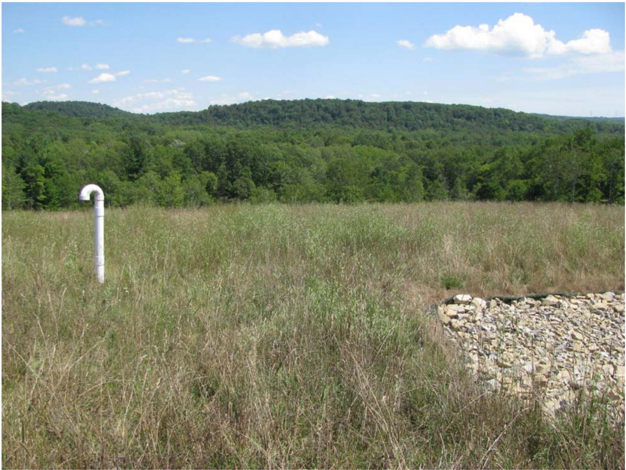
PHOTO 7: Repaired gas vent riser near mid-cap swale.
