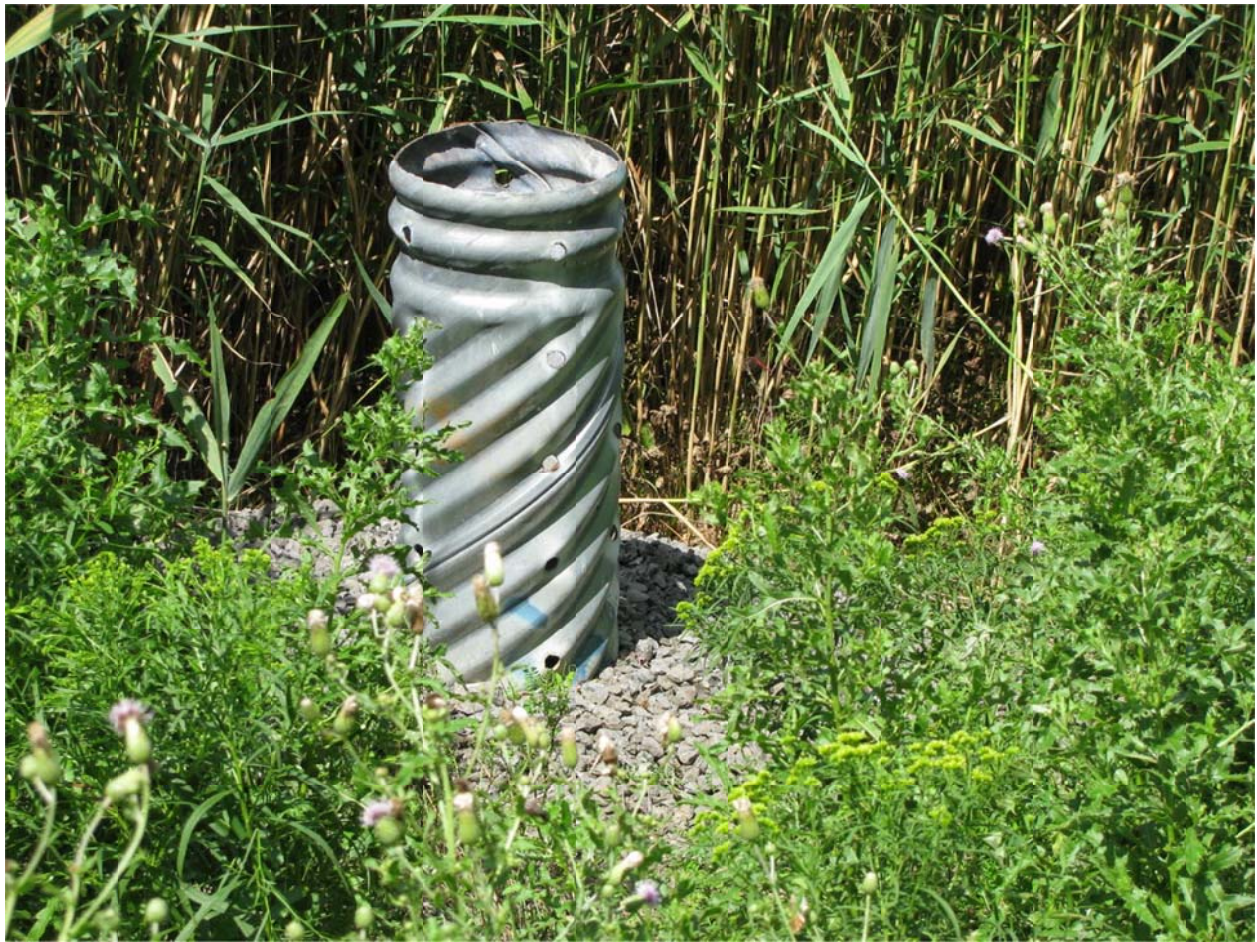
PHOTO 6: Outflow structure of south stormwater management pond. Note cleanliness of gravel blanket. The gravel does not appear to have been inundated.
