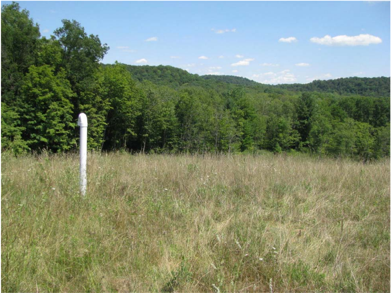
PHOTO 8: Second repaired gas vent riser.
