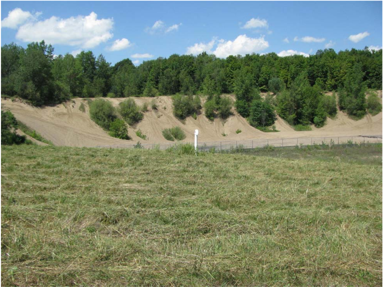
PHOTO 9: Third repaired gas vent riser in area just mowed
