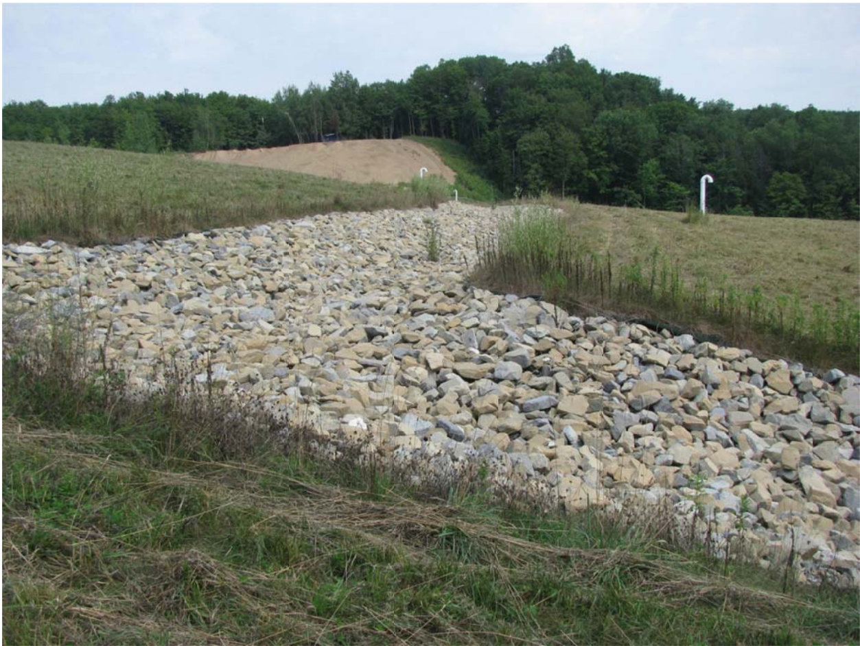
PHOTO 3: Look north at the cleanliness of the stone lining of a swale and downchute.
