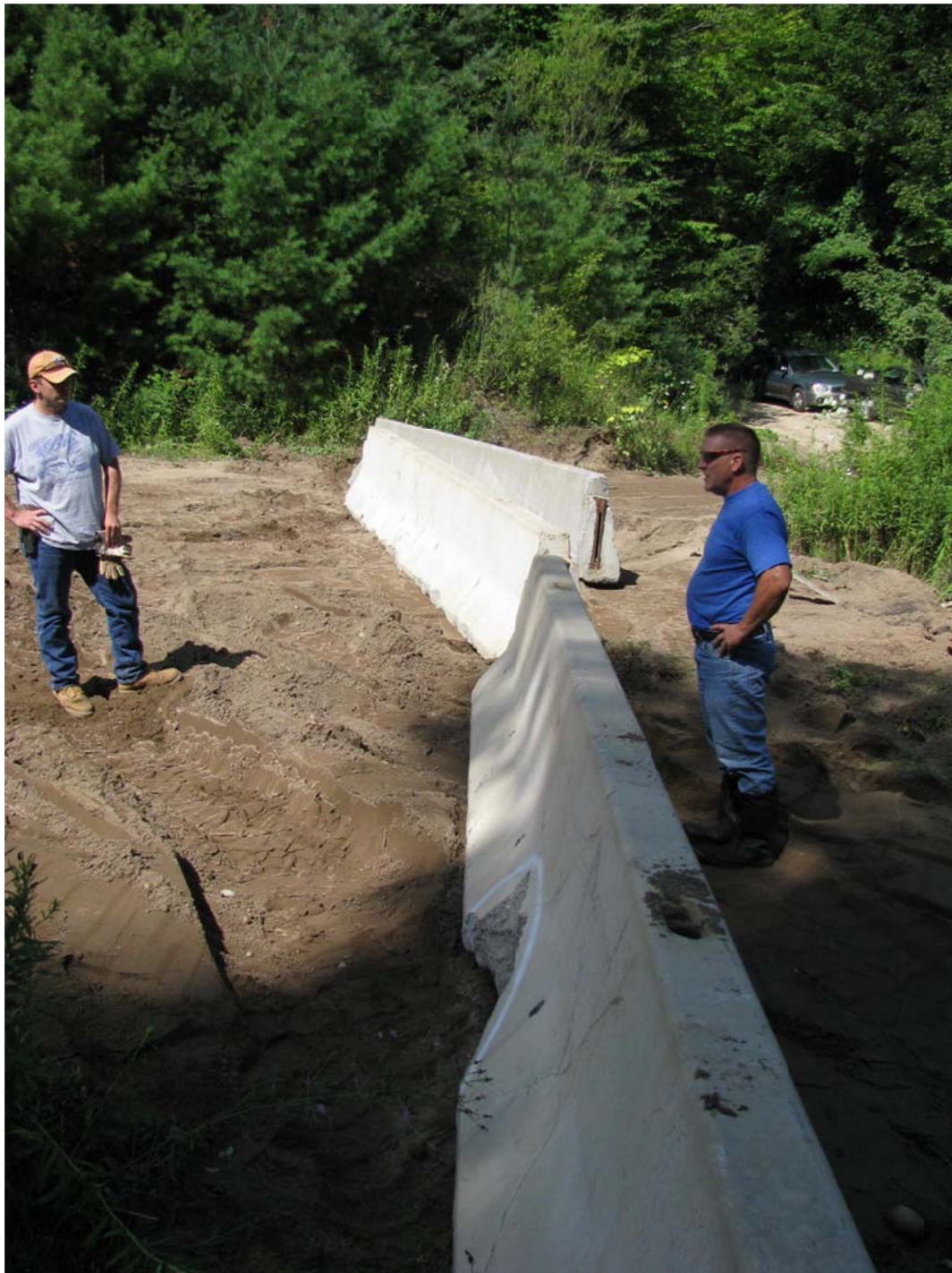
PHOTO 3: Jersey barriers in place, allowing for passage of smaller vehicles (ATVs, etc.), but not trucks
