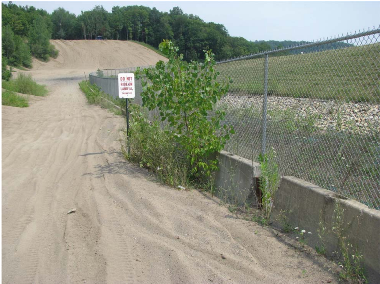
PHOTO 7: Look north along the western fence and vandalism barrier. Note the degree to which the sand has accumulated against the barriers.
