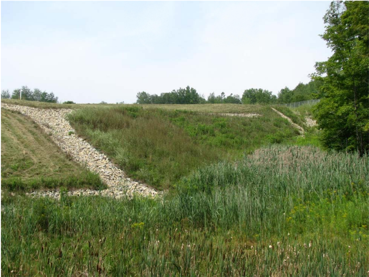
PHOTO 5: Look west from the north stormwater management pond at a portion of the final cover that Marcy did not mow. Note that this is the area in which there were two slides during construction. I discussed with Marcy's man on-site, and did not raise any objection to the area remaining un-mowed at the time. Given the steepness of the slope, this area should be minimally maintained, only to correct any erosion that may occur (none was noted) and to remove woody vegetation..
