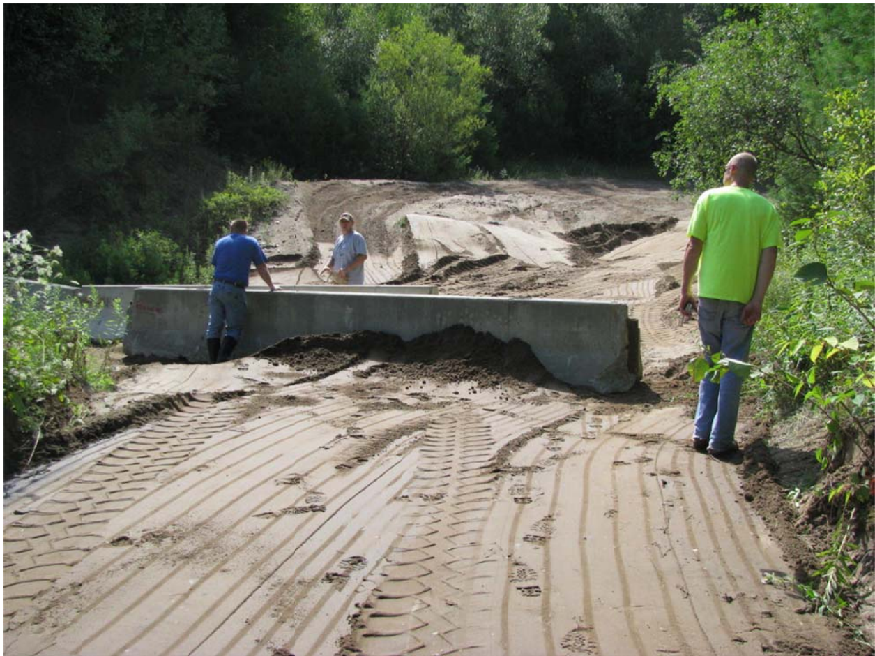
PHOTO 4: Same as in PHOTO 3. The front barrier was subsequently slid farther to the right to make passage on that side more difficult.
