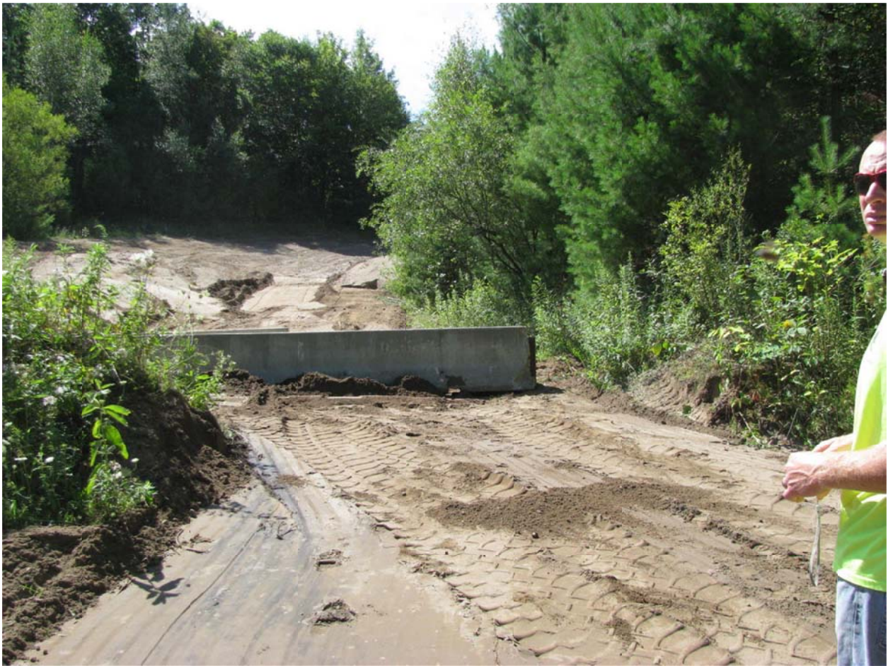
PHOTO 1: Jersey barriers across side accesss road leading onto landfill.
