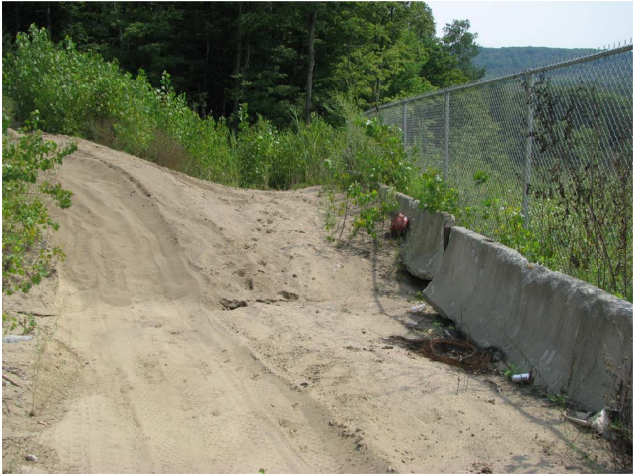
PHOTO 9: The northeast corner of the landfill perimeter. Beyond the small rise, the ground slopes steeply down, ultimately to the north stormwater management pond. The erosional problem discussed in this report occurs about halfway to the pond. Note the channel cut under barrier by stormwater runoff from the adjacent hill to the north (left). That stormwater flows under the fence and then is picked up and carried downhill by the channel whose end has collapsed as can be seen in the next photo. Thus, this flow pattern appears to be contributing to the above-mentioned erosion problem, though to an uncertain degree.
