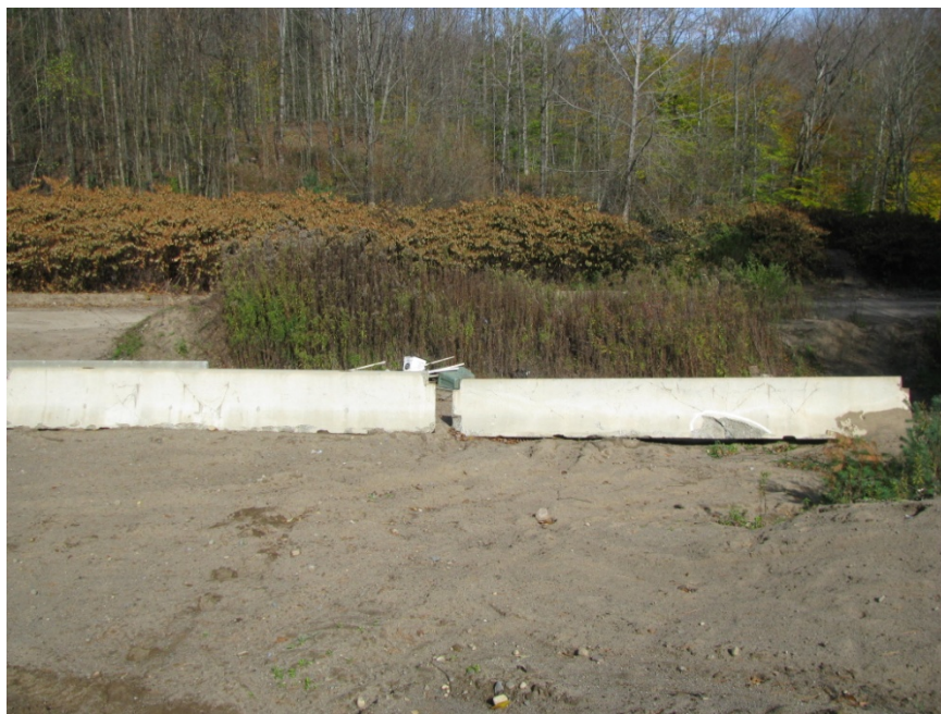
Photo 5: 10/17/12 Jersey barrier installed near Military Road to limit site access and trash disposal.
