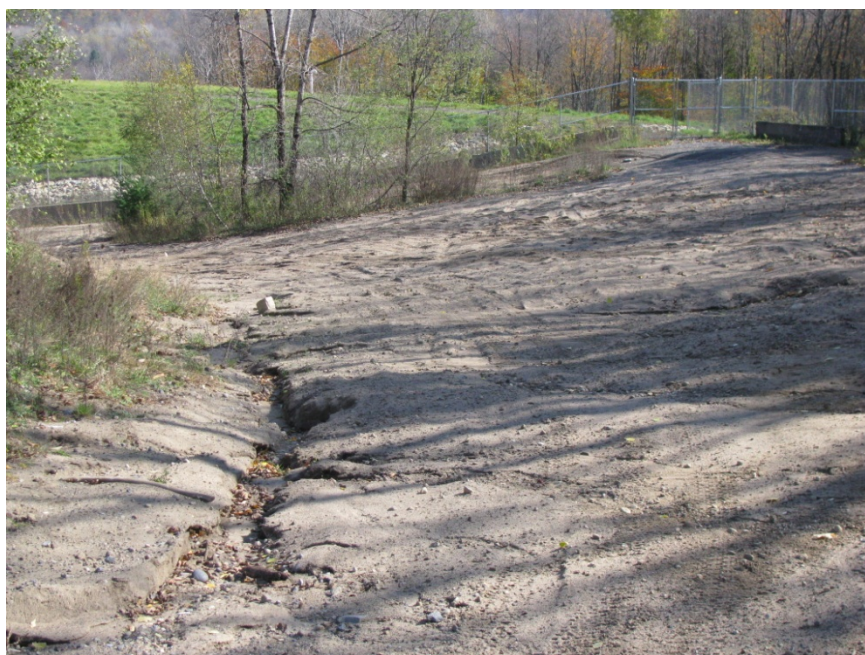
Photo 18: 10/18/12 Looking east at landfill. The rilling/erosion in this area is starting to re-occur. Erosion is up to 1 foot across and 1 foot deep.
