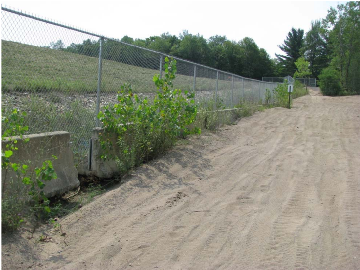
PHOTO 8: Look south along the western fence and vandalism barrier. Note the degree to which the sand has accumulated against the barriers.
