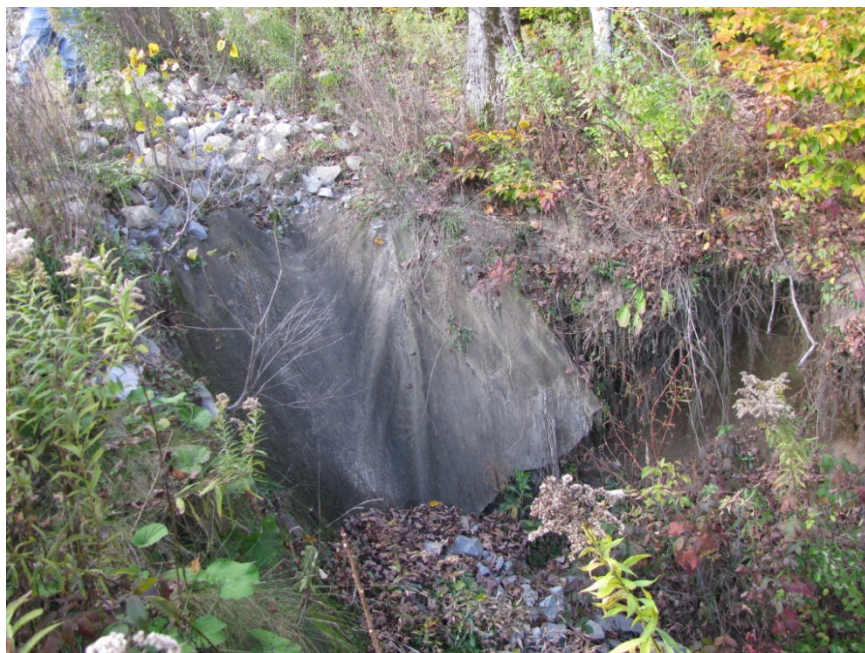
Photo 24: 10/18/12 Erosion occurring north of landfill, exposing fabric. Continued monitoring is advised.
