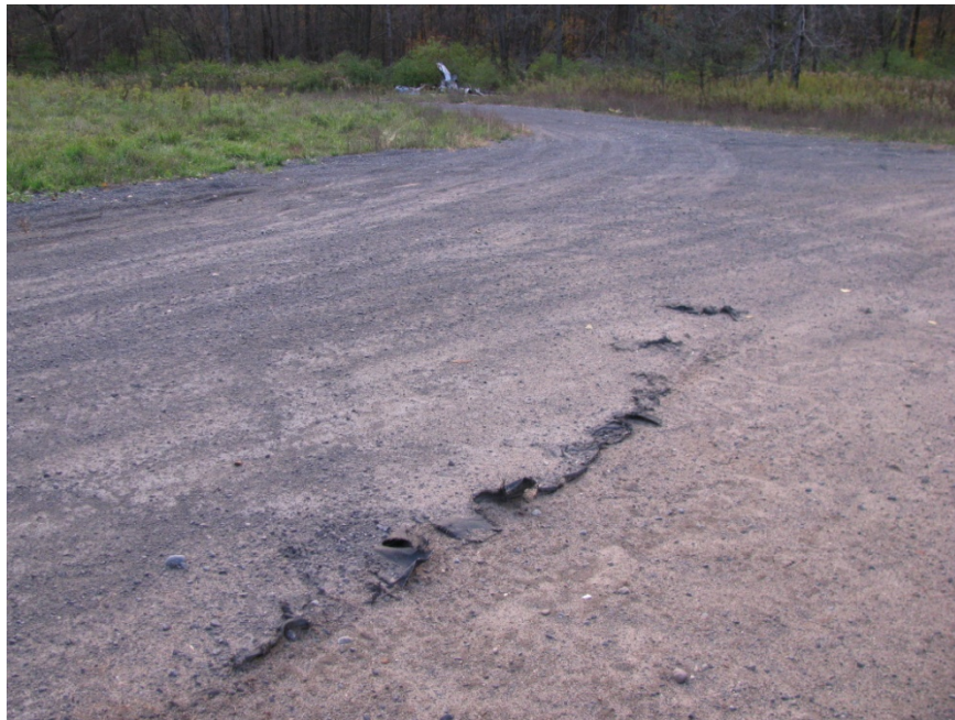
Photo 34: 10/18/12 Erosion exposing geotextile fabric at along site access road, approximately half way between front gate and actual landfill.
