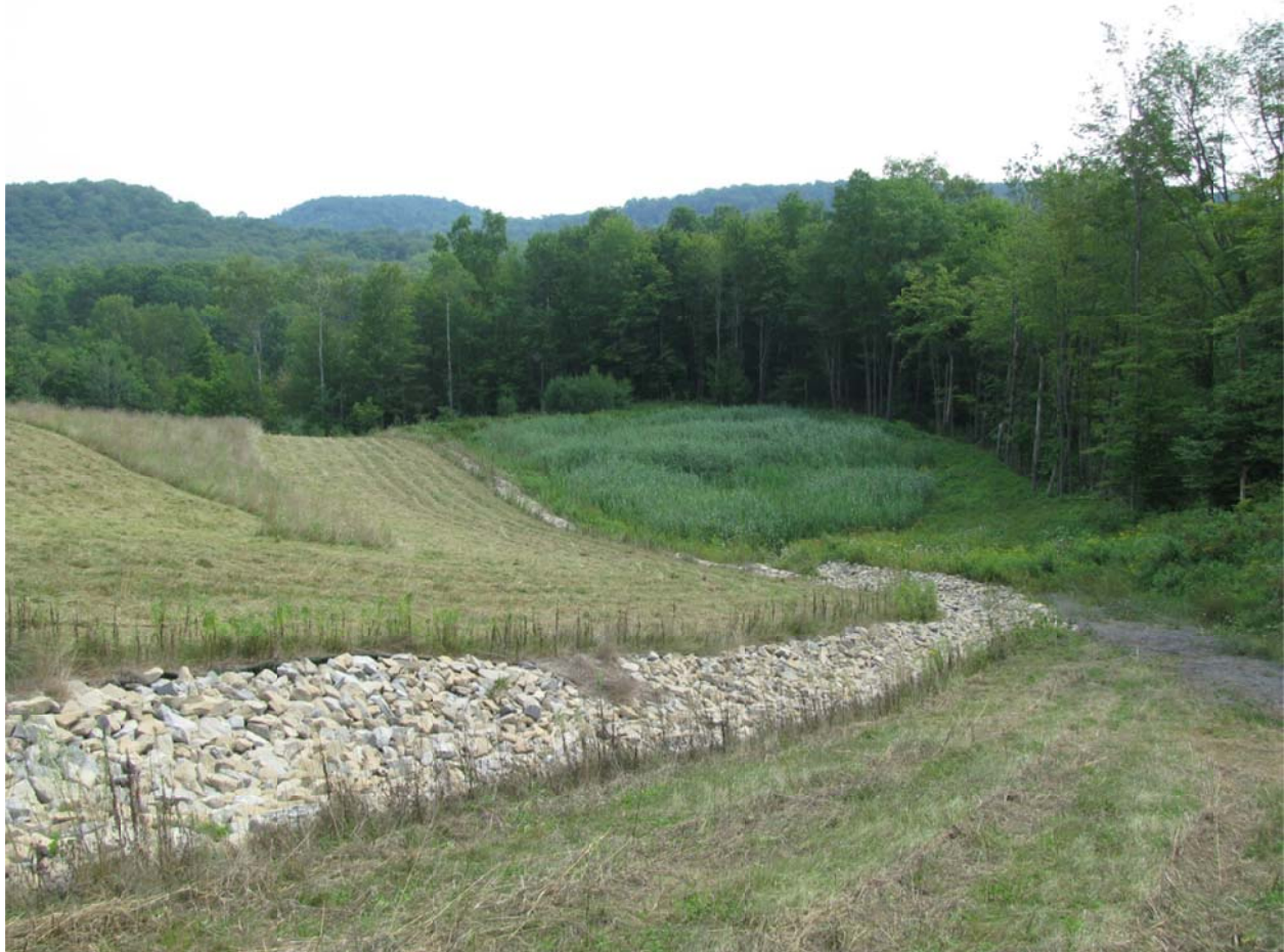
PHOTO 1: Look downslope and east along the southern boundary of the landfill at the south stormwater management pond. Note that not all of the cap had been mowed by this time.
