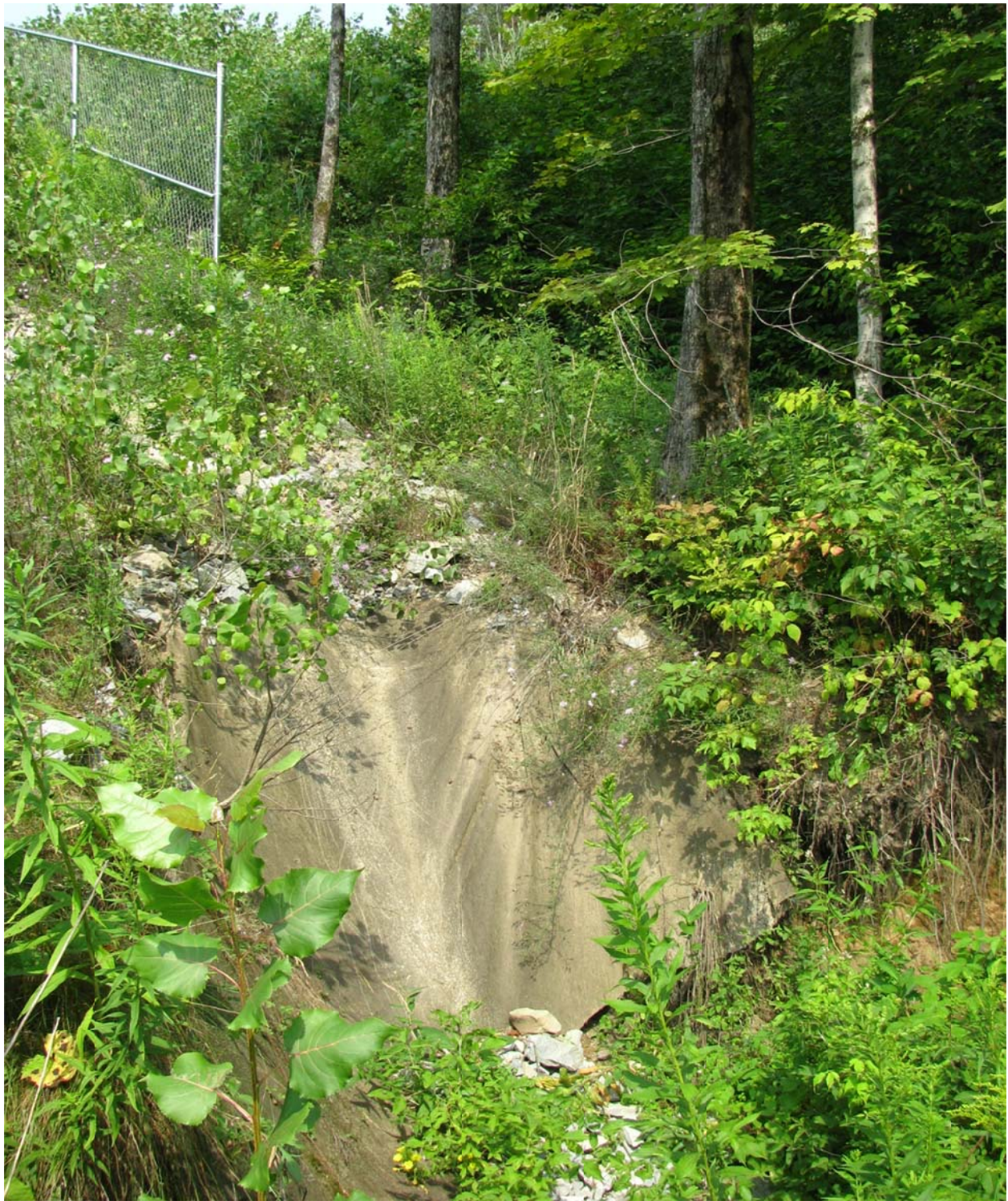
PHOTO 10: Look northwest at the erosion problem discussed in this report. Note the location of the fence and trees for future reference.
