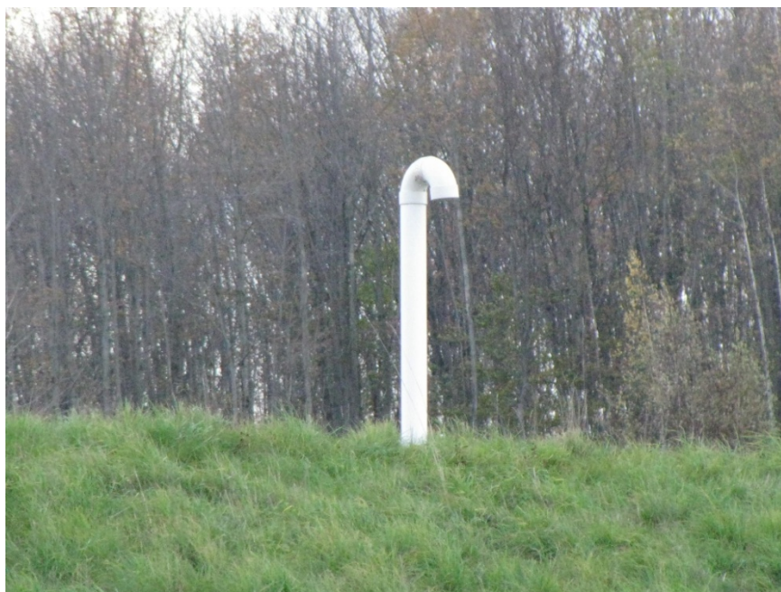
Photo 32: 10/18/12 Close-up of gas vent.
