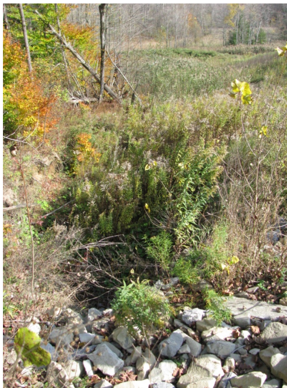
Photo 25: 10/18/12 Erosion occurring at area where rip-rap terminates. Looking east towards North Detention Pond.
