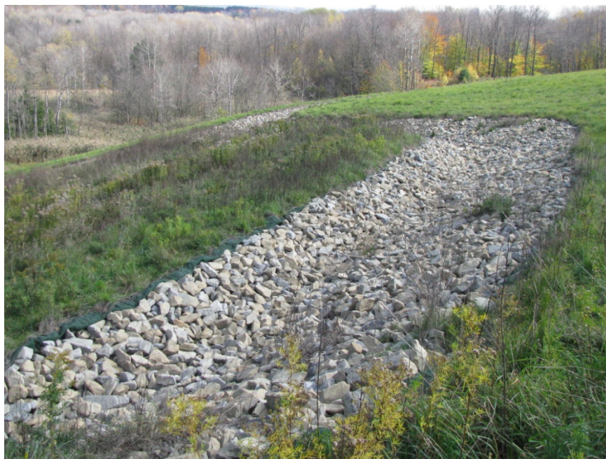
Photo 23: 10/18/12 Standing on north side of landfill looking southeast at rip-rap lined drain chutes.
