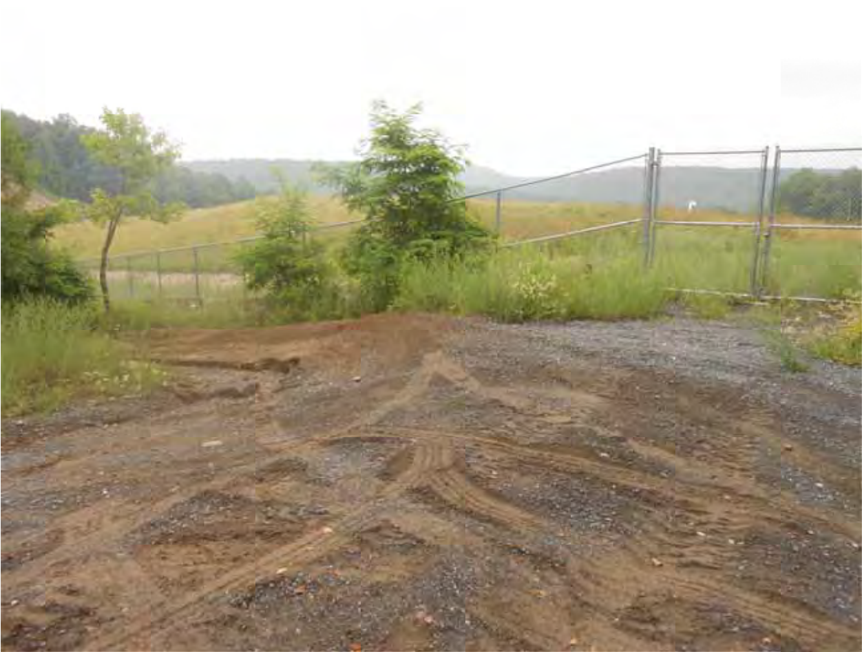
Photo 13: 07-10-13 Looking east towards top of landfill. Traffic from all-terrain vehicles are causing erosion rills to form on the access road.
