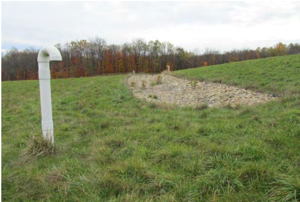
Photo 8: 10/16/13 Standing at the center of the landfill, looking south at gas vents and rip-rap lined drain chutes.
