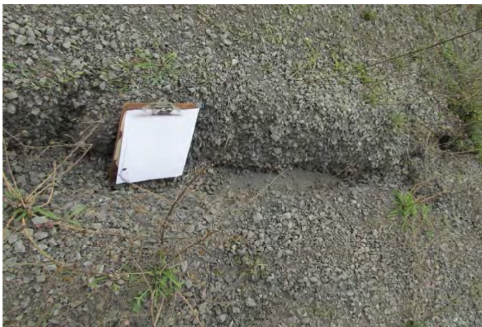
Photo 6: 10/16/13 Close-up of erosion/rilling occurring in access road on top of landfill. Note fabric has been exposed.
