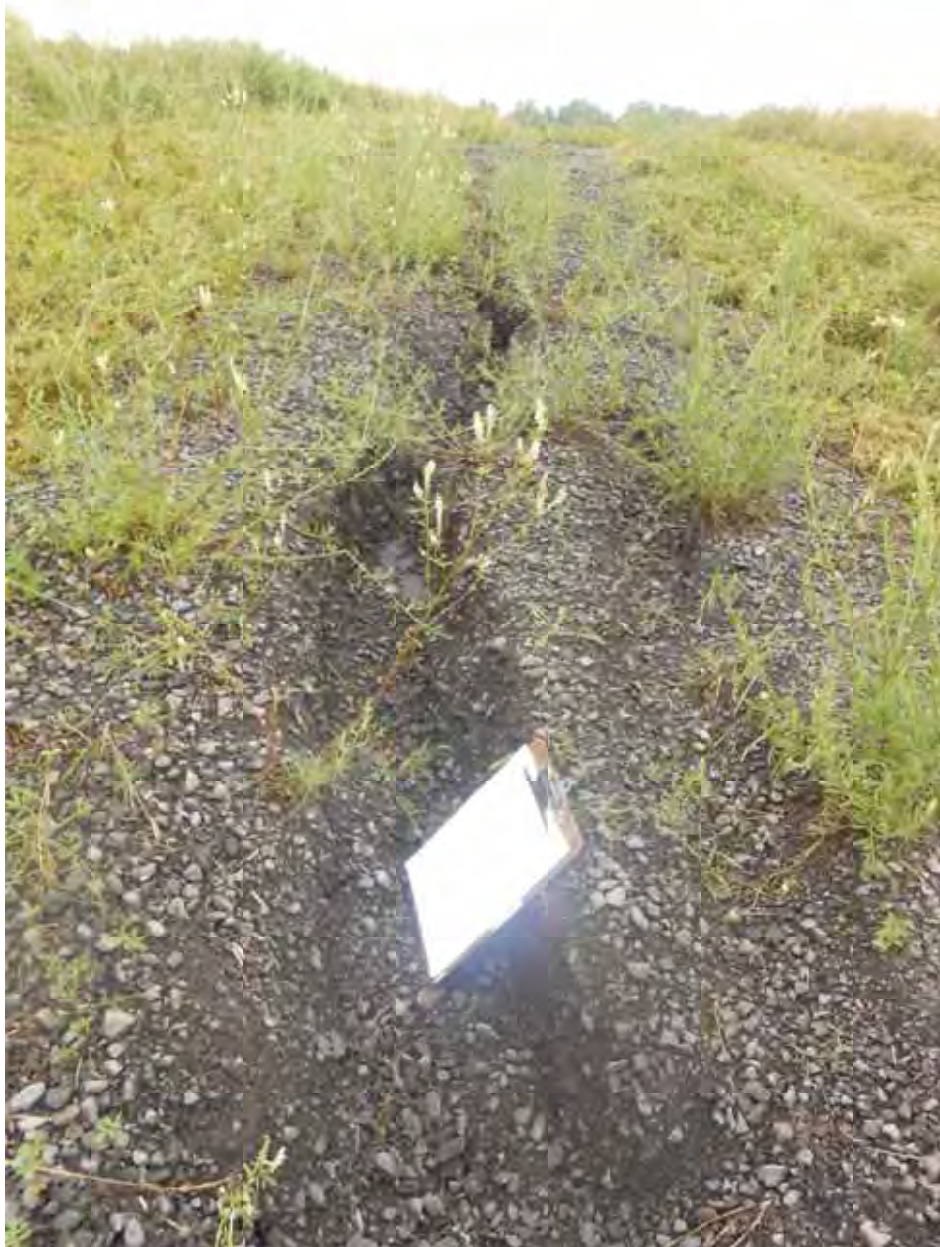
Photo 6: 07-10-13 Looking southwest at top of landfill. Erosion rills approximately 10 inches deep are forming on the access road on top of the landfill.
