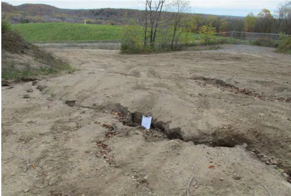
Photo 1: 10/16/13 Looking east towards the landfill. The erosion/rilling in this area is starting to re-occur.
