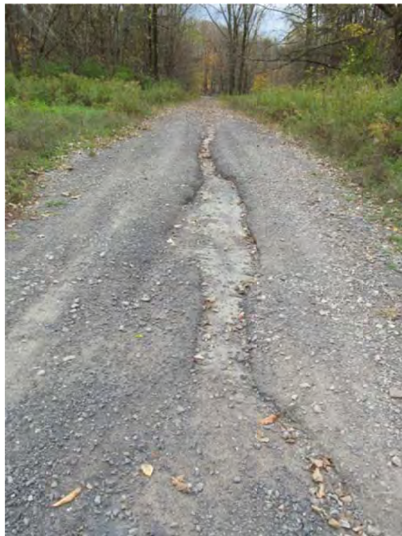
Photo 24: 10/16/13 Erosion/rilling in gravel access road west of landfill.
