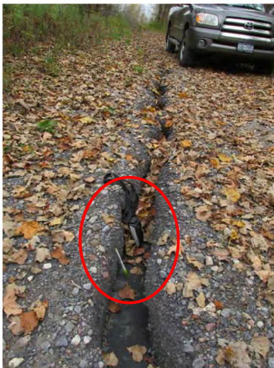
Photo 25: 10/16/13 Erosion/rilling in access road west of landfill. Note camera case and pen for scale.
