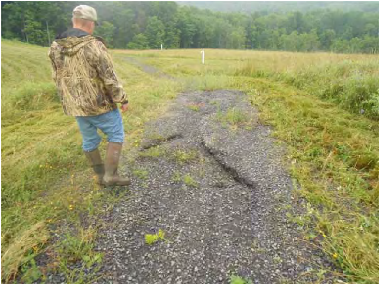
Photo 5: 07-10-13 Looking northeast at top of landfill. Erosion rills approximately 10 inches deep are forming on the access road on top of the landfill.
