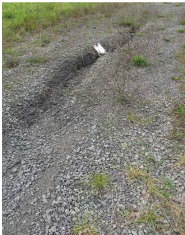
Photo 5: 10/16/13 Erosion/rilling in access road on top of landfill. In some areas the erosion is approximately 12 inches deep.
