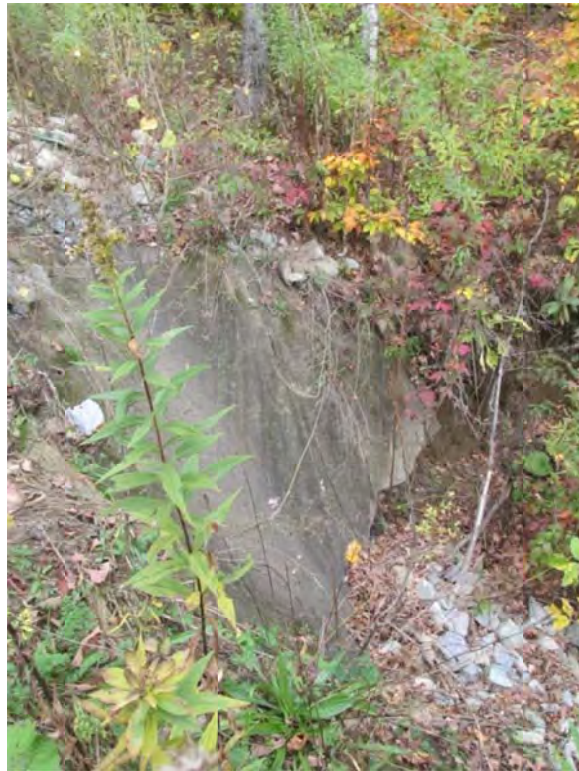
Photo 11: 10/16/13 Erosion occurring north of landfill, exposing fabric.
