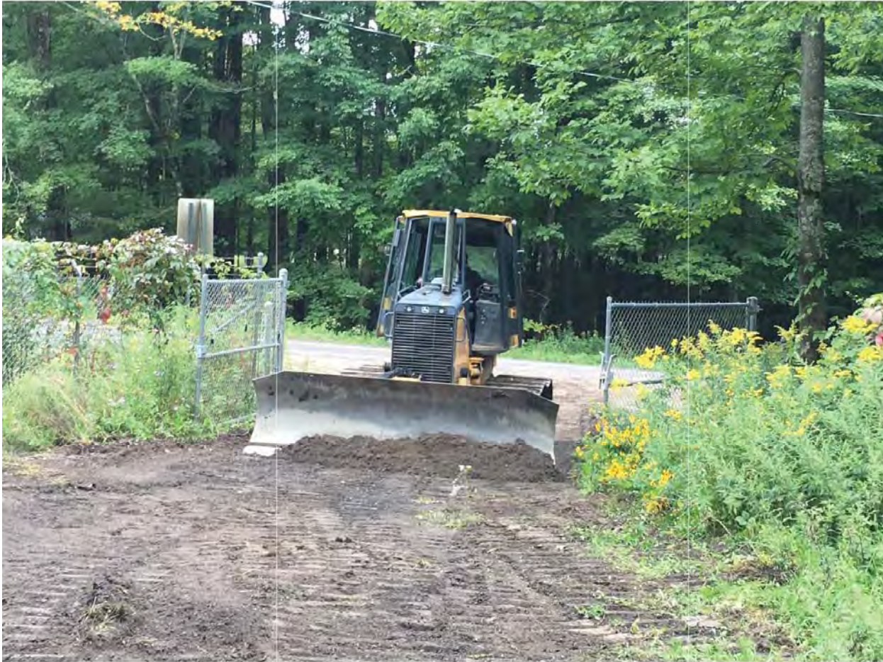
Photo 8 – Looking Southwest– Entrance gate area being regraded to facilitate gate operation.
