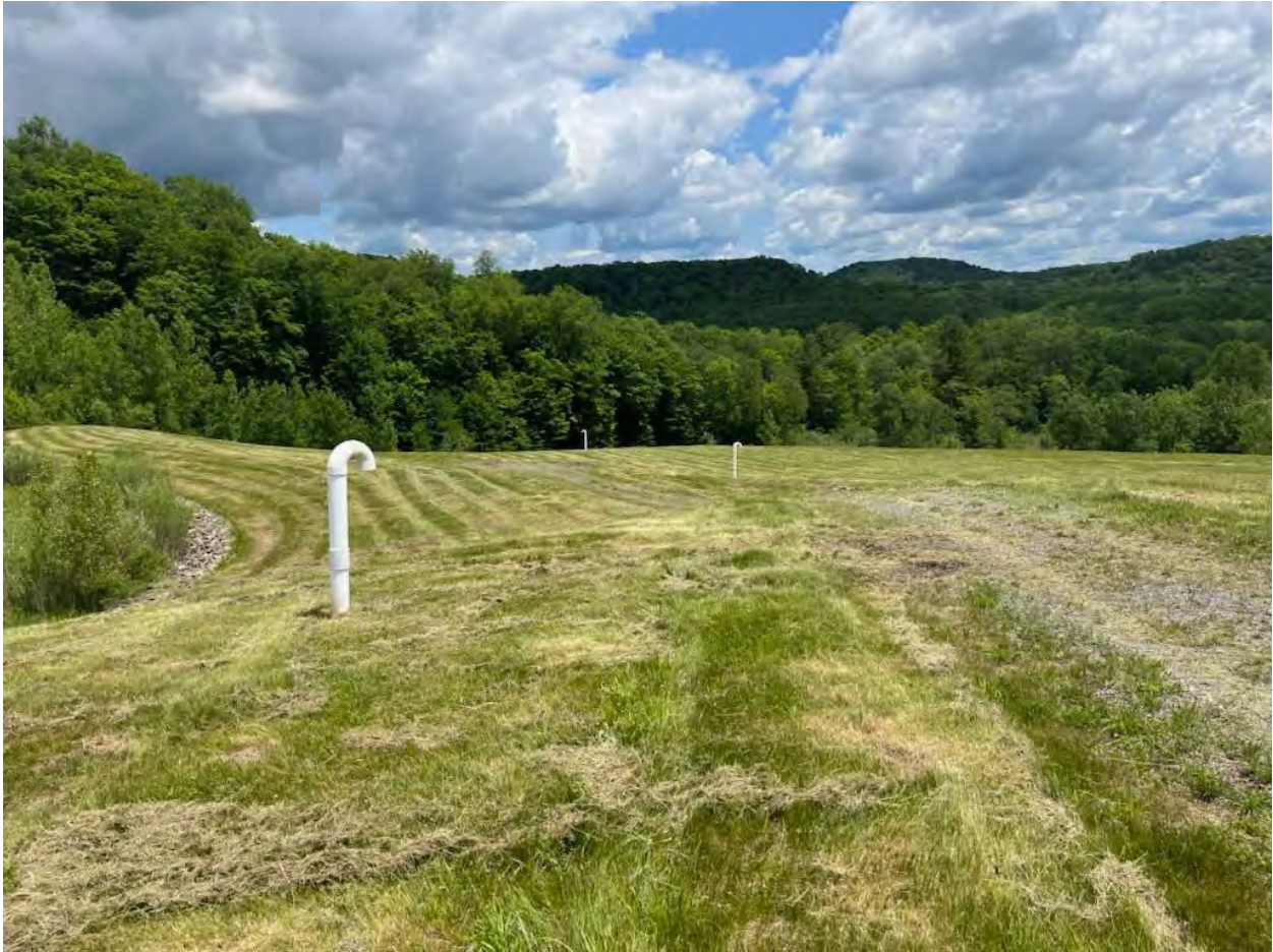
Photo 26 – Looking south – Methane vents on a recently- mowed portion of the landfill cap.
