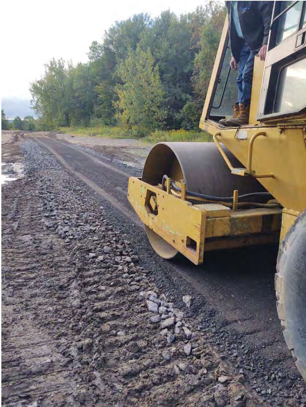
Photo 9 – Looking East – Smooth drum roller used to compact crusher run on top of No. 4 stone.
