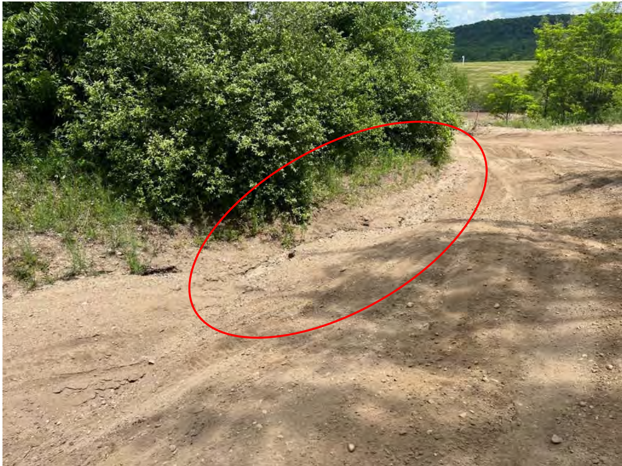
Photo 11 – Looking east towards the landfill from the landfill access road. Erosion and washouts are occurring along the shoulder (circled).
