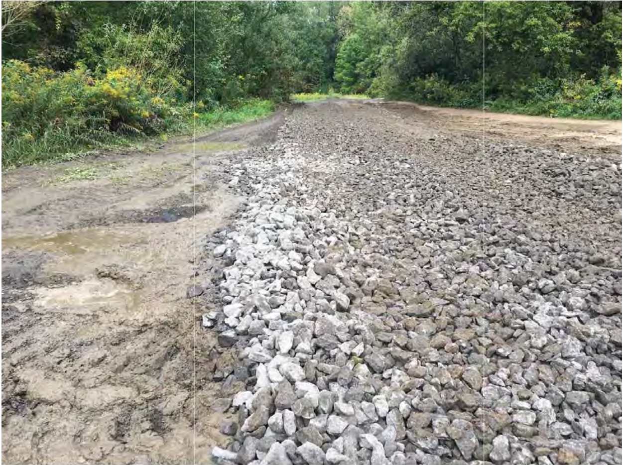
Photo 16 – Looking Northwest – After regrading and draining ponded surface water, No. 4 stone placed to create stable subbase in wet unstable portion of site access road.
