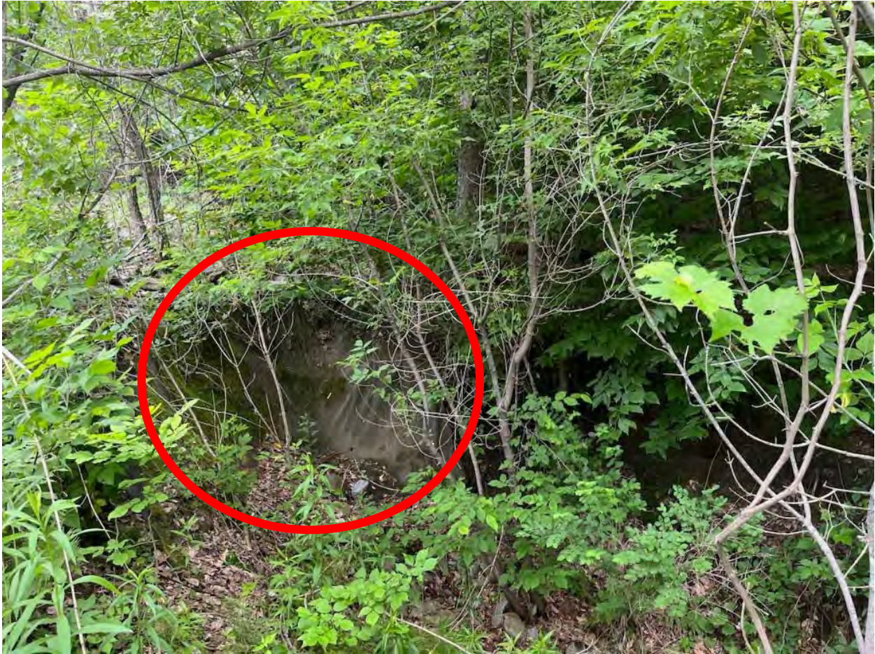
Photo 15 – A location that AECOM uses to evaluate sloughing in the outer perimeter swale on the northern edge of the landfill. Some filter fabric is exposed (circled). No additional sloughing or erosion has been observed over the past several site visits.
