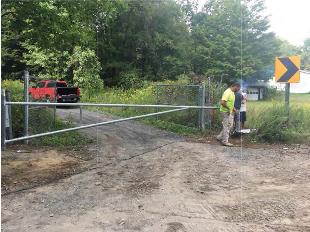
Photo 7 – Looking Northeast– Newly installed crash gate located at site entrance. The crash gate is outside of the existing double swing gate.
