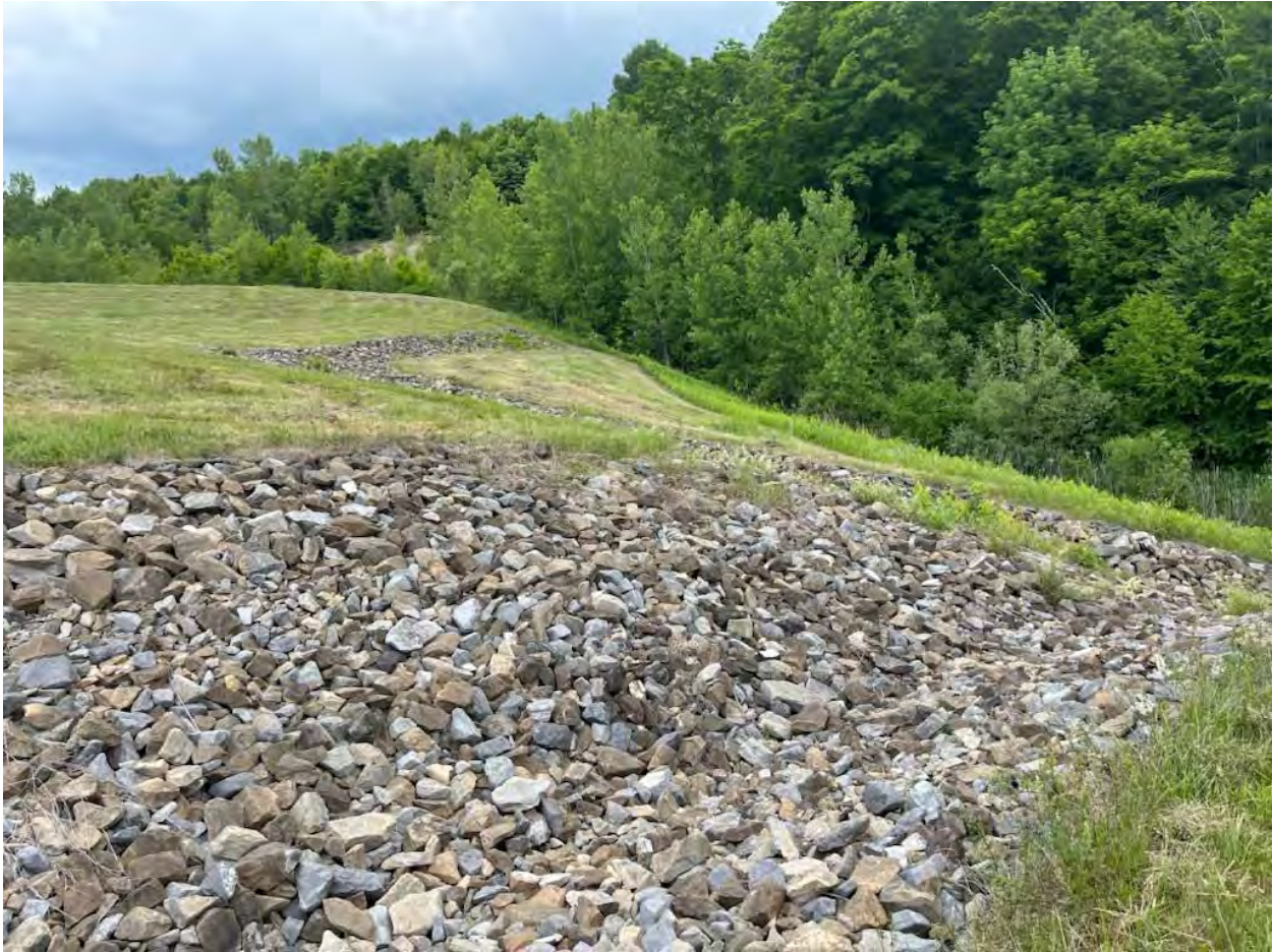
Photo 19 – Looking north at the landfill cap drainage swale after woody vegetation had recently been cleared out of the swale by AECOM.
