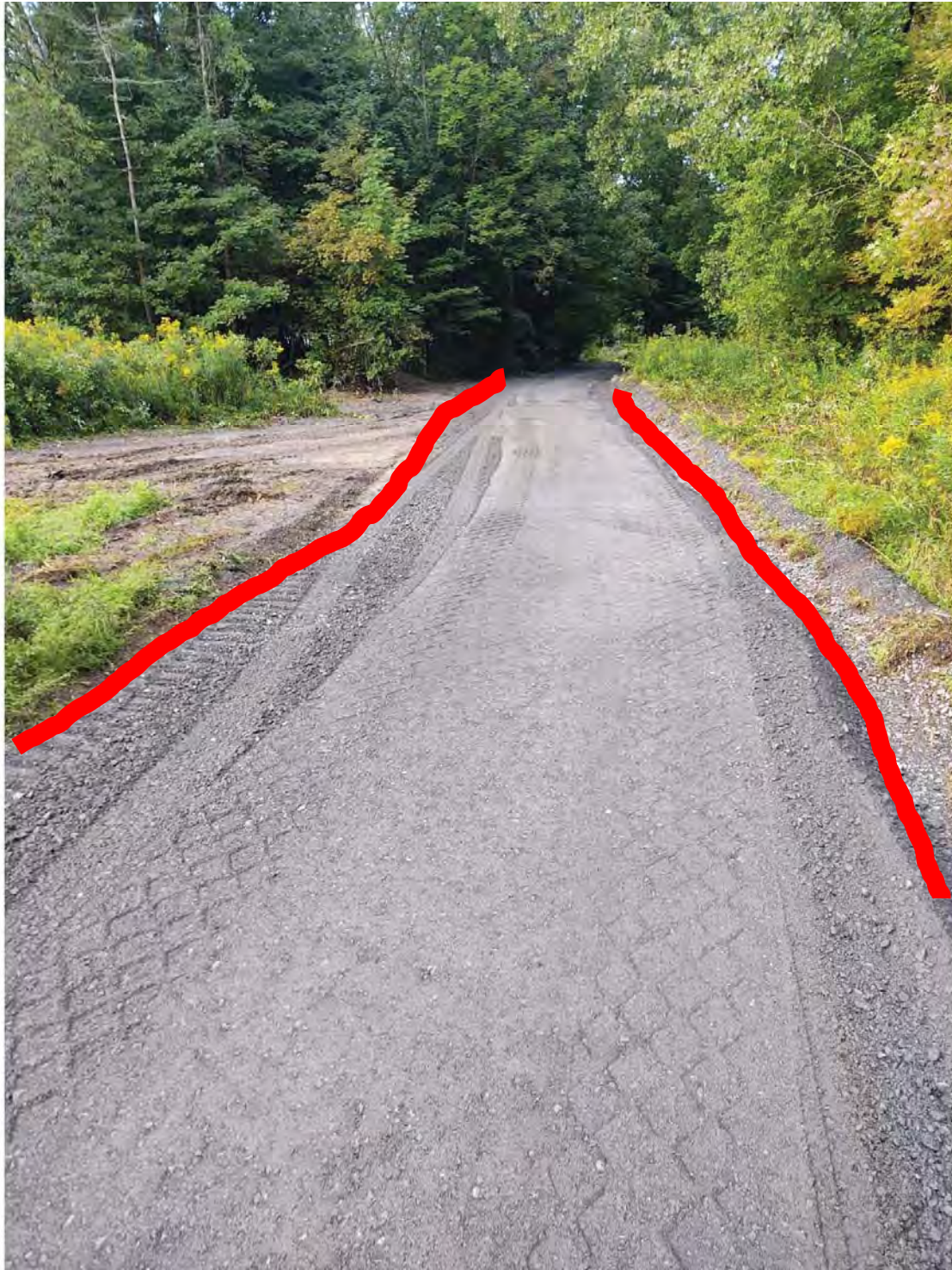
Photo 10 – Looking Southwest – Access road following repairs. Also shown (red lines) are surface water diversion swales.
