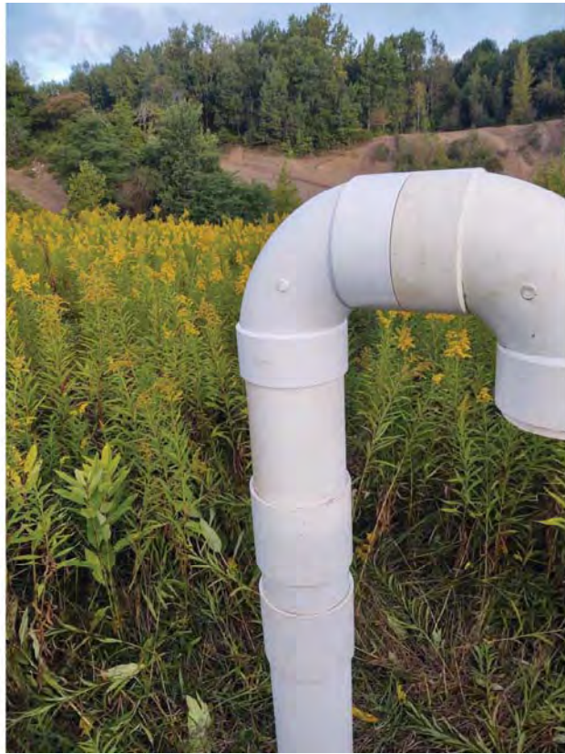
Photo 11 and 12 – Two repaired methane gas vents.
