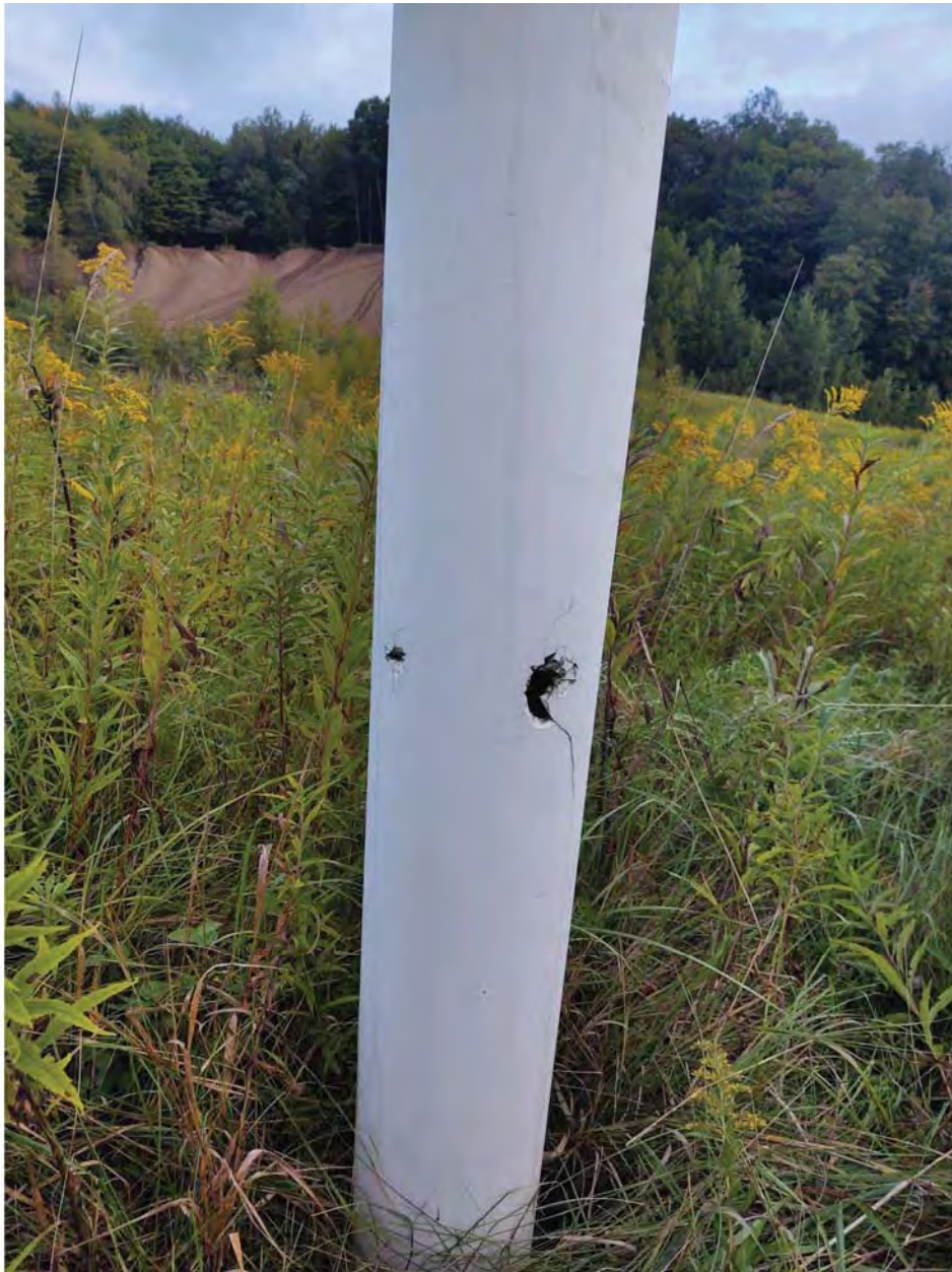
Photo 10 –Damaged methane gas vent prior to repair (bullet hole).
