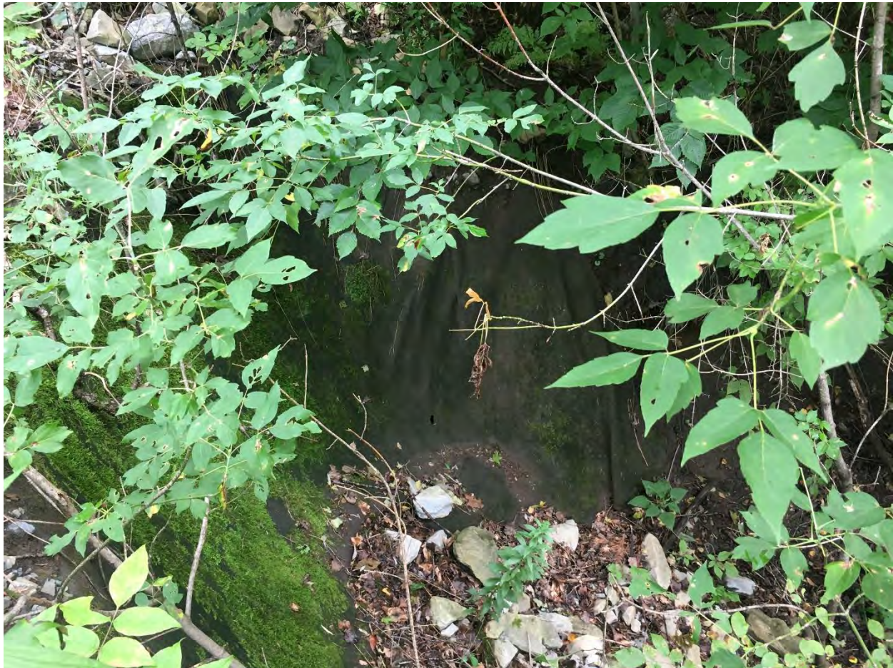
Photo 15 – Diversion channel liner. Head cutting was initially observed here during the August 9, 2012 inspection. No significant change to the extent of the head cutting has been observed since.
