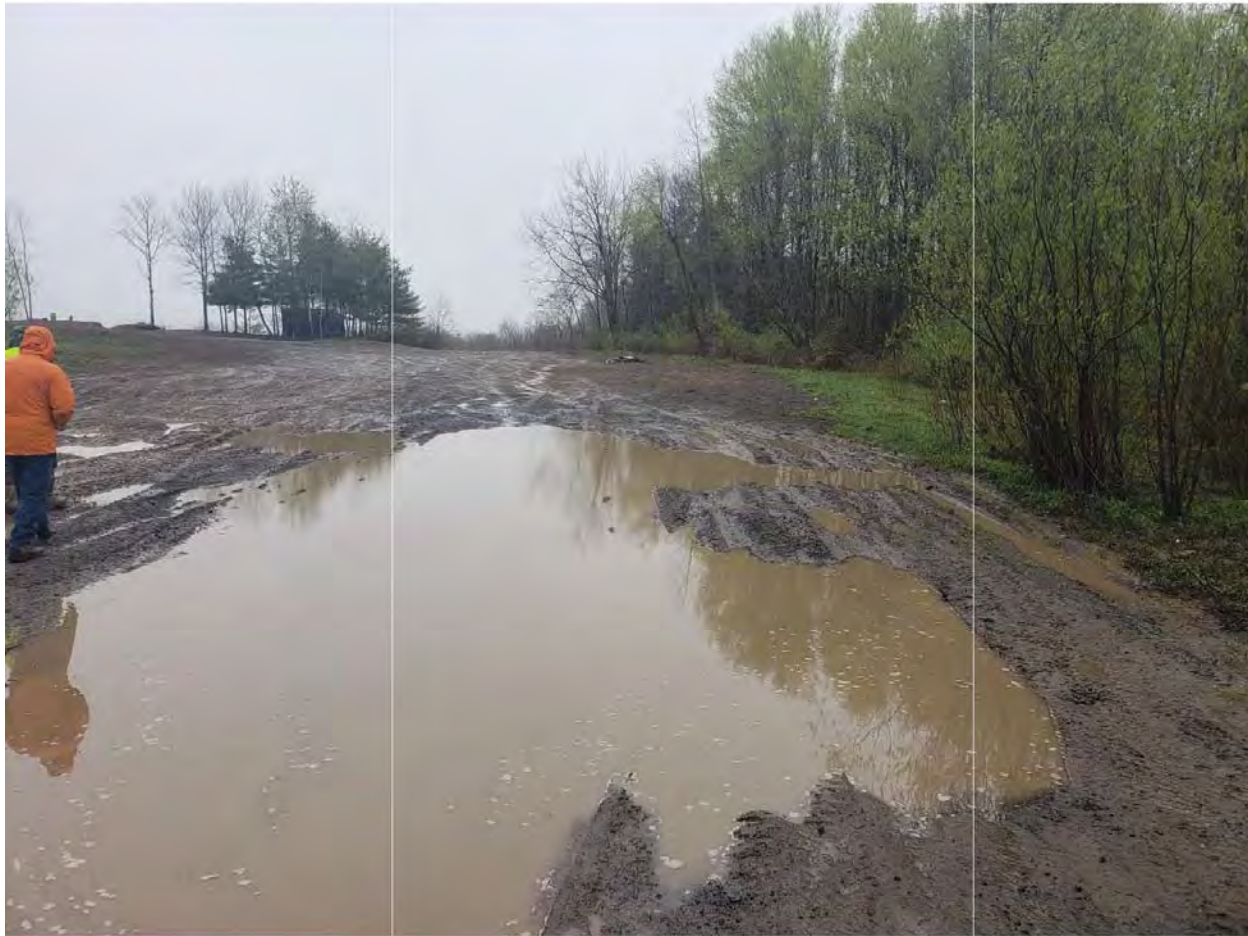
Photo 18 – Looking East – Wet, unstable portion of site access road prior to regrading for improved surface water drainage, and placement of No. 4 stone as shown in Photo 16.
