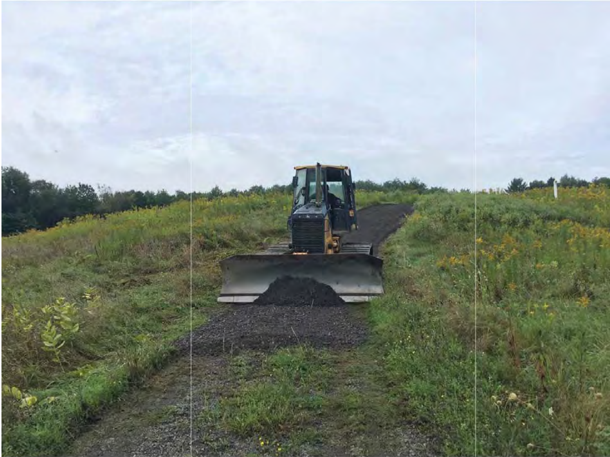
Photo 14 – Looking Southwest – Grading of material placed as shown in Photo 13.
