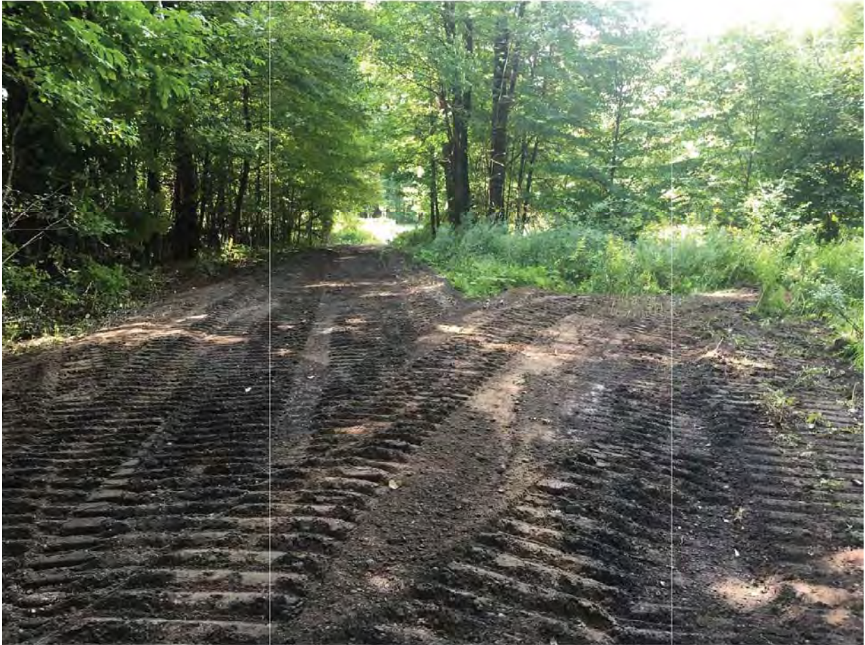
Photo 6 – Looking West – Site access road rough-graded to divert surface water away from site access road.
