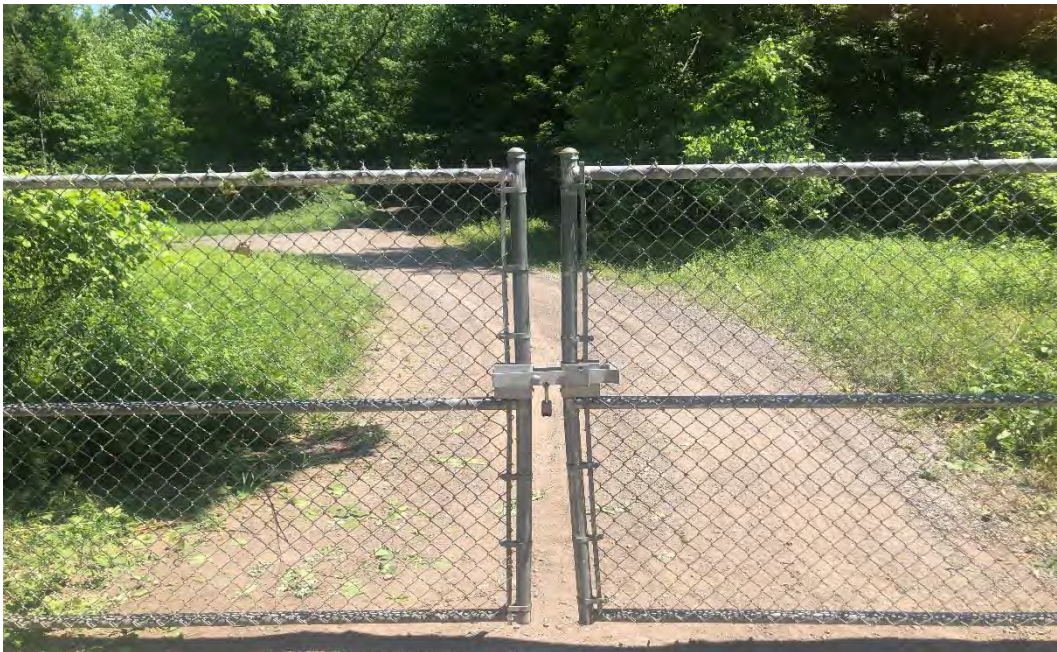
Photos 5 and 6 – Looking east at the main gate after repairs and installation of the new latch and padlock.
