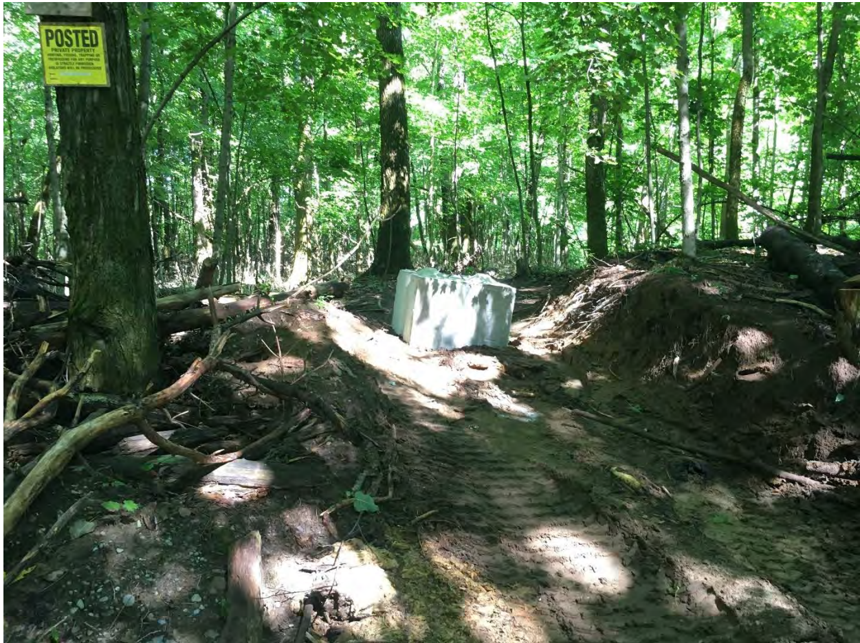
Photo 6 – Concrete block installed to limit ATV access to the Site from east side of Bromley Road.
