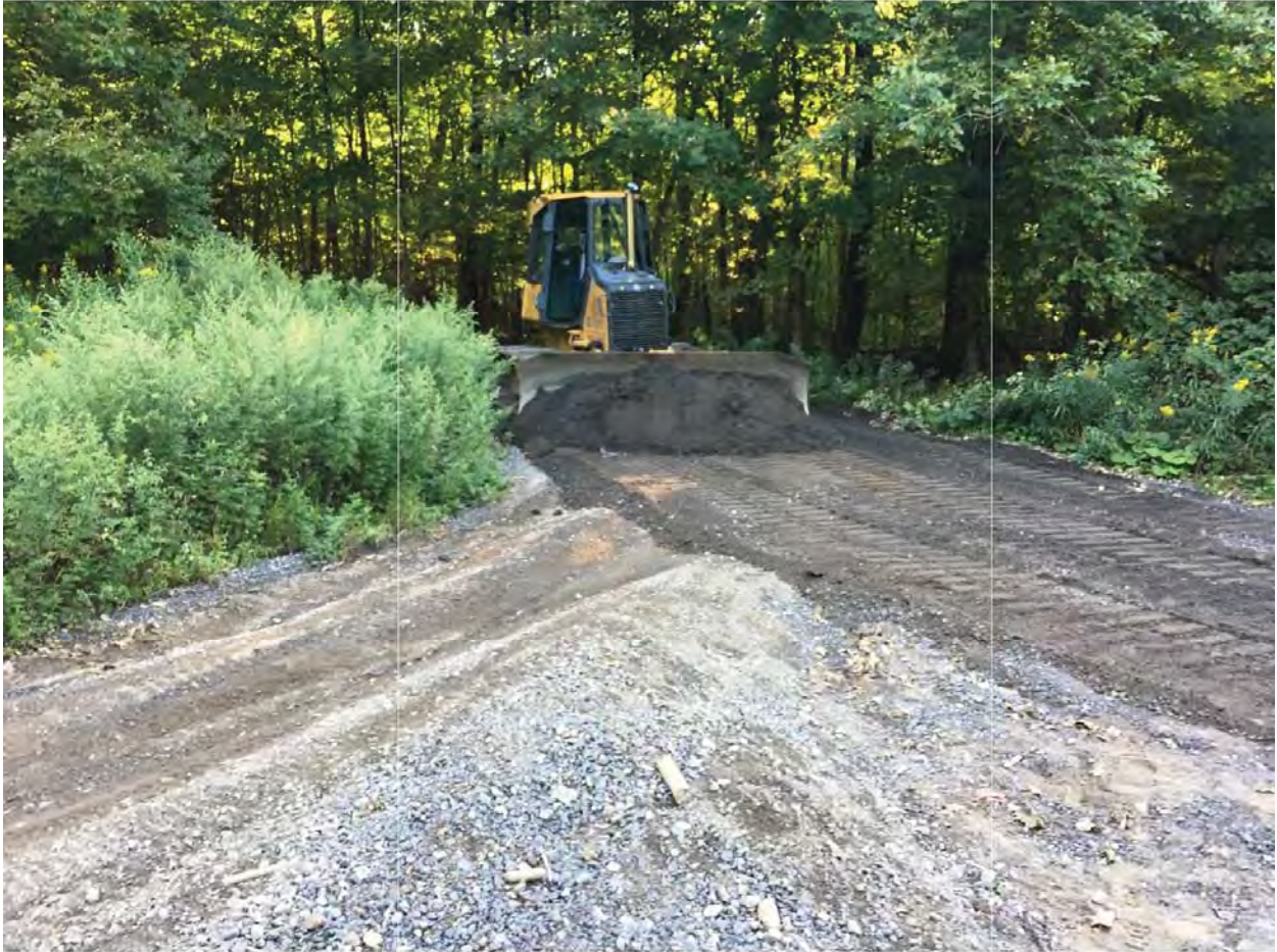
Photo 5 – Looking Southwest – Rough grading site access road with existing crusher run.
