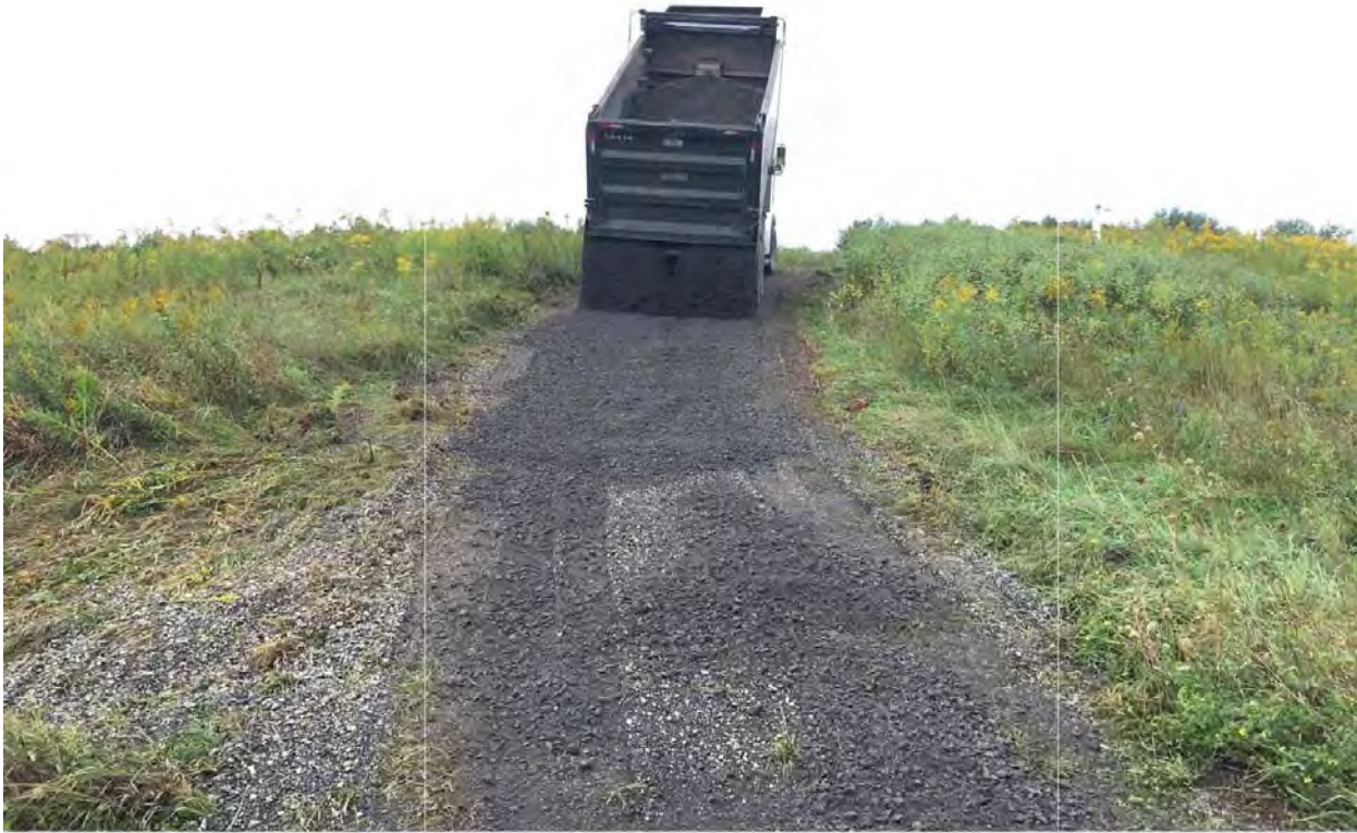
Photo 13 – Looking Southwest – Tandem dump truck placing crusher run on the landfill road to fill eroded portion of road.
