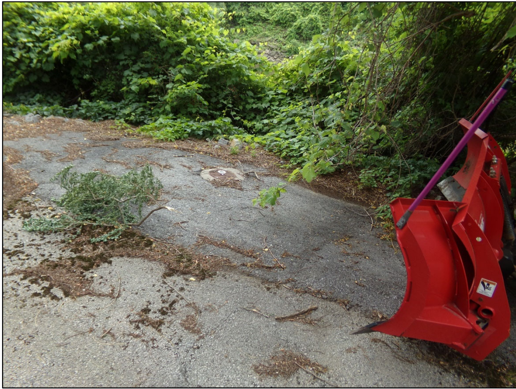
Site Conditions on July 26, 2024
