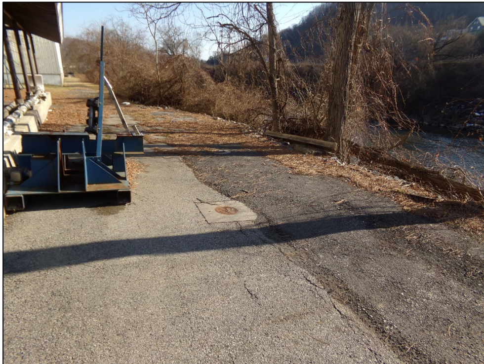
Site Conditions on December 15, 2023
