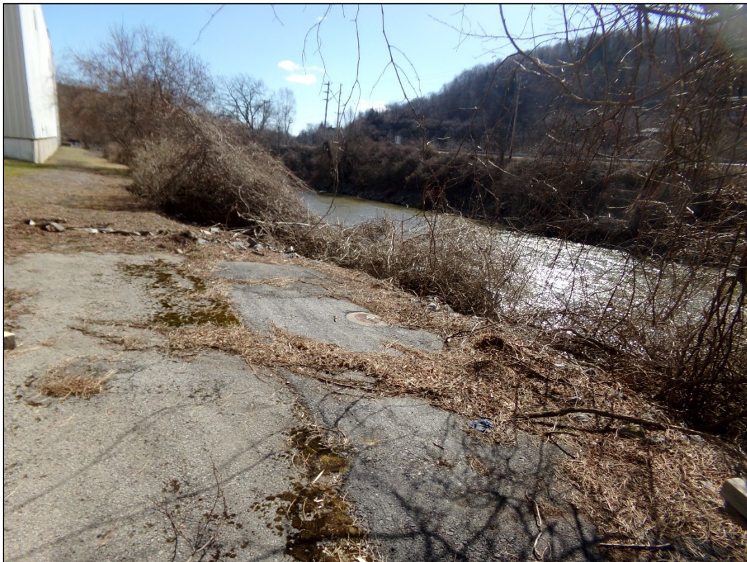
Site Conditions – March 2025
