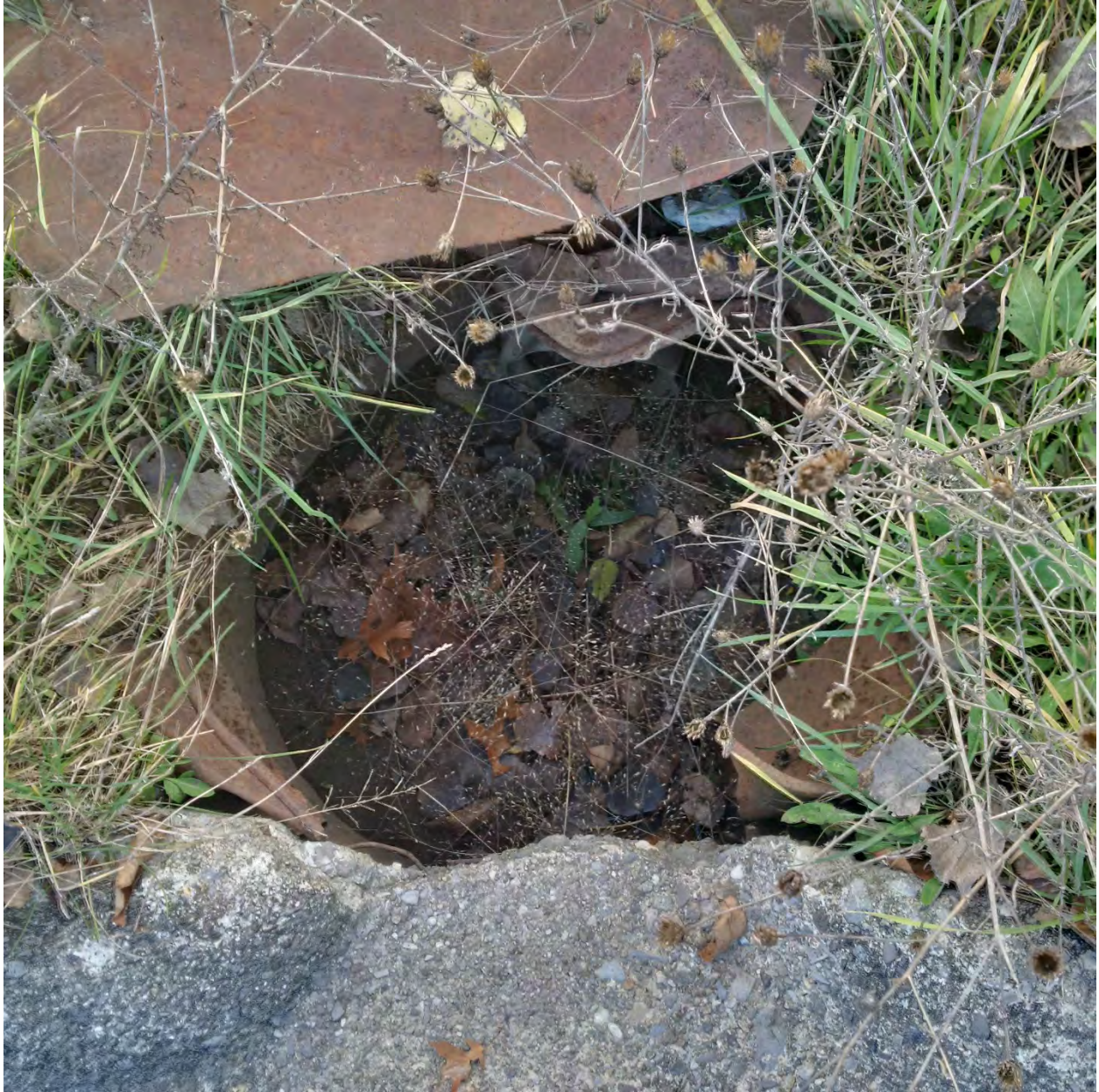
Figure 13 - Laundry Pad 2 Sump
