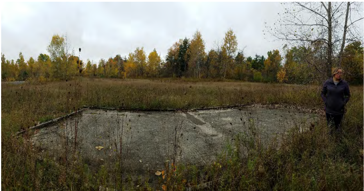
Figure 9 - Laundry Pad 1 Looking Toward Leachate Field
