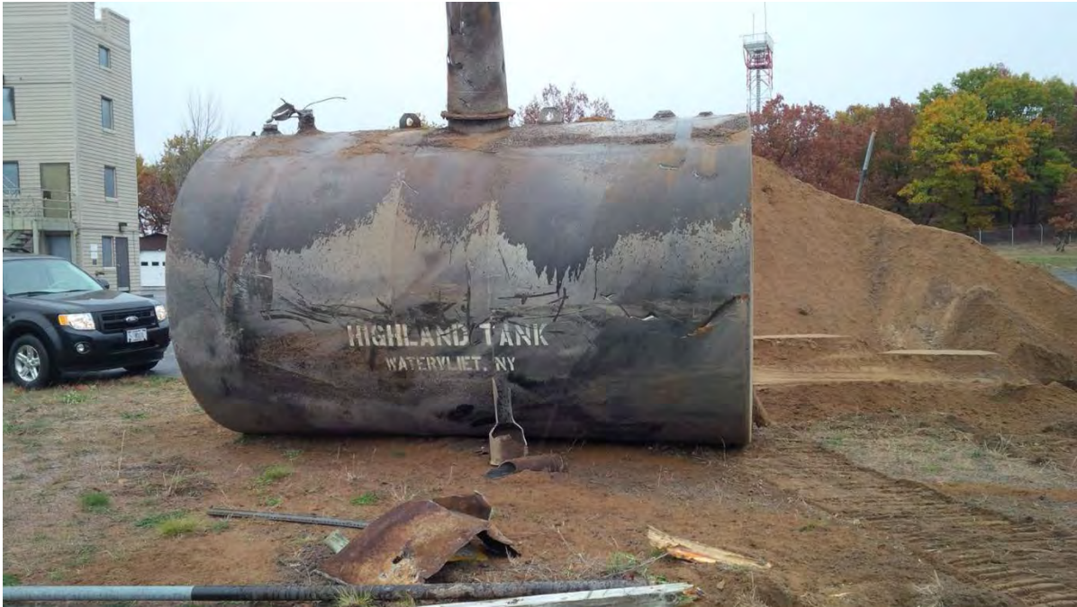
Figure 4 - 5,000 Gallon Steel Storage Tank
