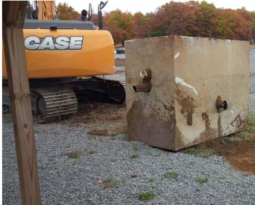
Figure 6 - Oil Water Separator
