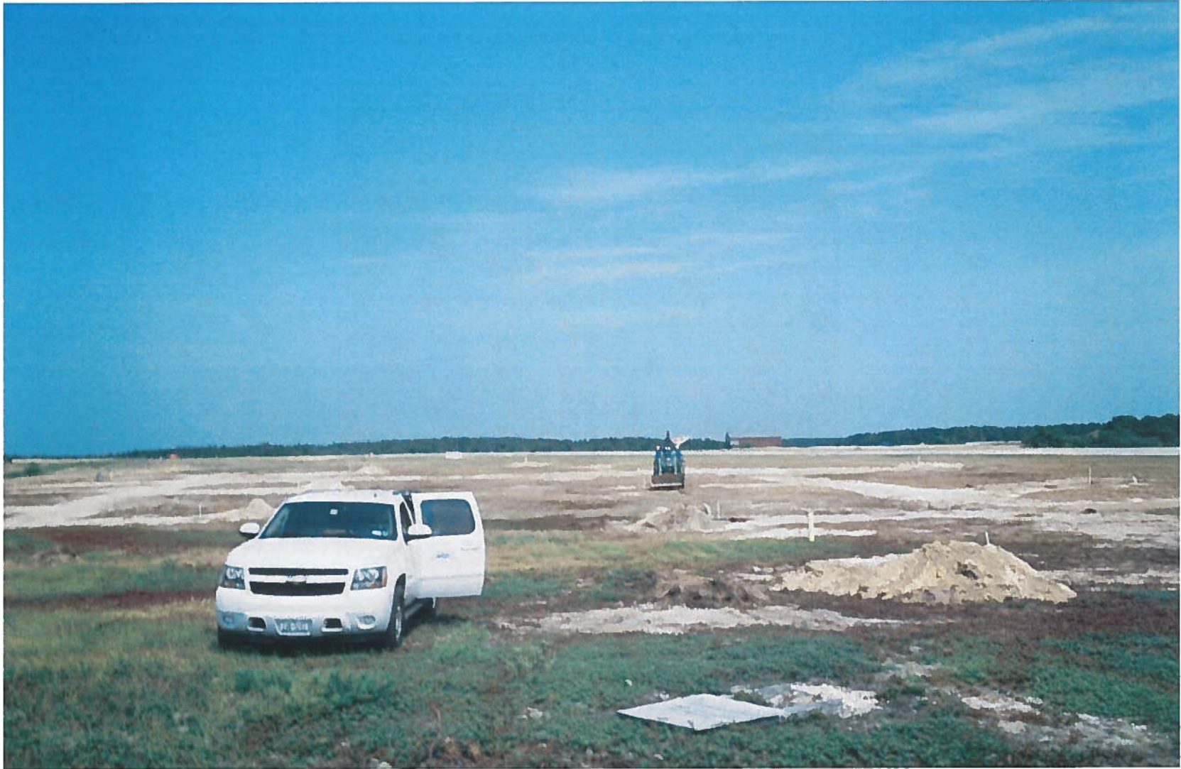
Photo 8. Air Biosparging Vault Installation and Backfilling of System Lines Across Site 4
