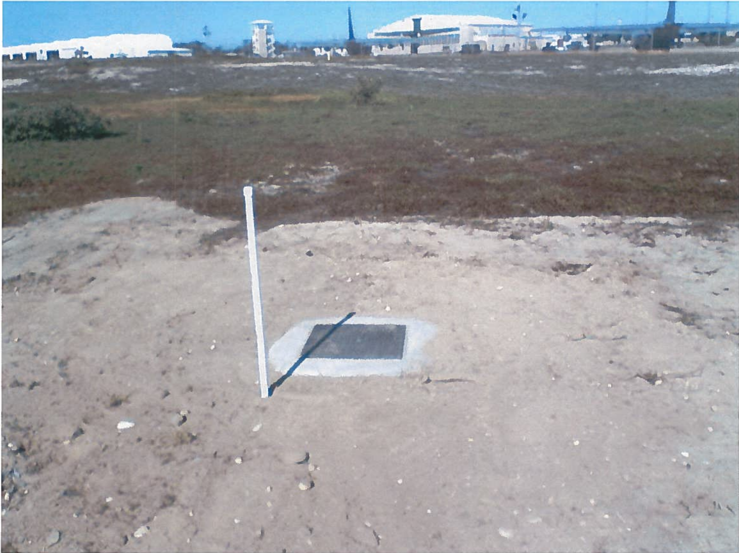
Photo 17. Typical Completed Air Biosparging Well Vault
