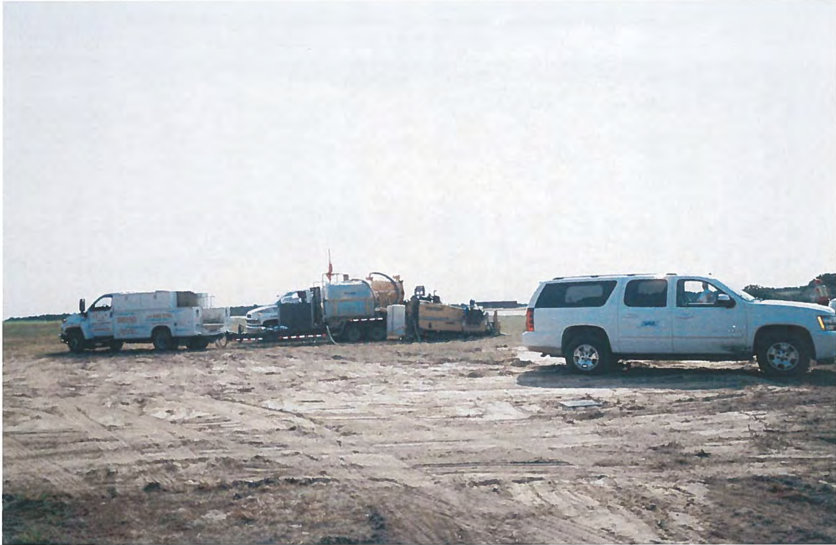
Photo 6. View of Directional Drill Rig Equipment in Operation
