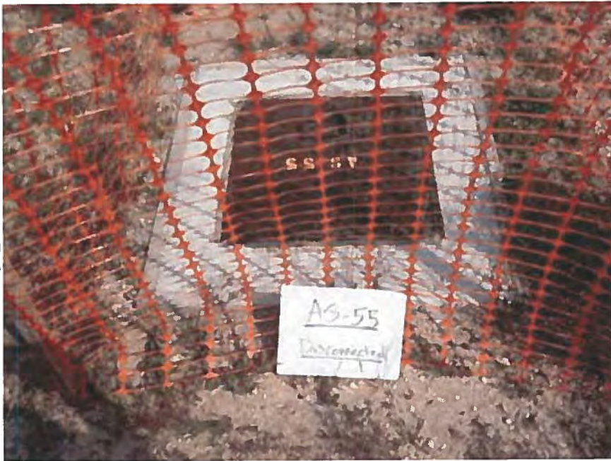
1. Valve Vault Protective Measure Example
