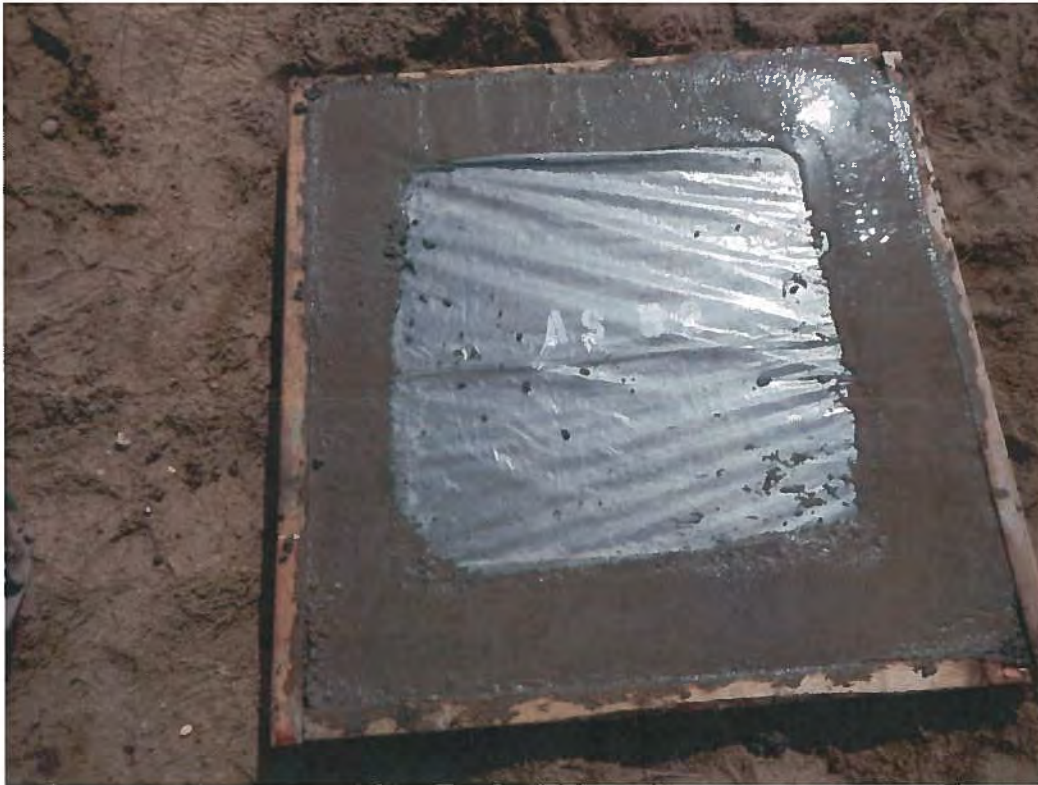
Photo 7: Installation of New Sparge Vault
