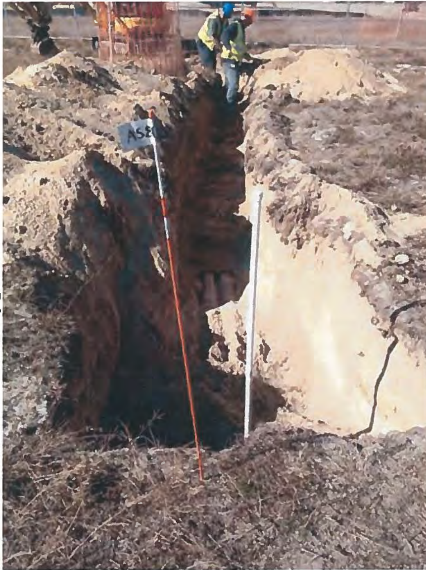
11. Trench to New AS-81 Sparge Well
