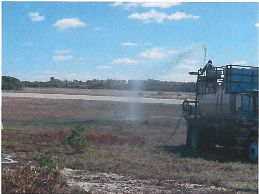
Photo 23: Disturbed land was restored using hydroseed
