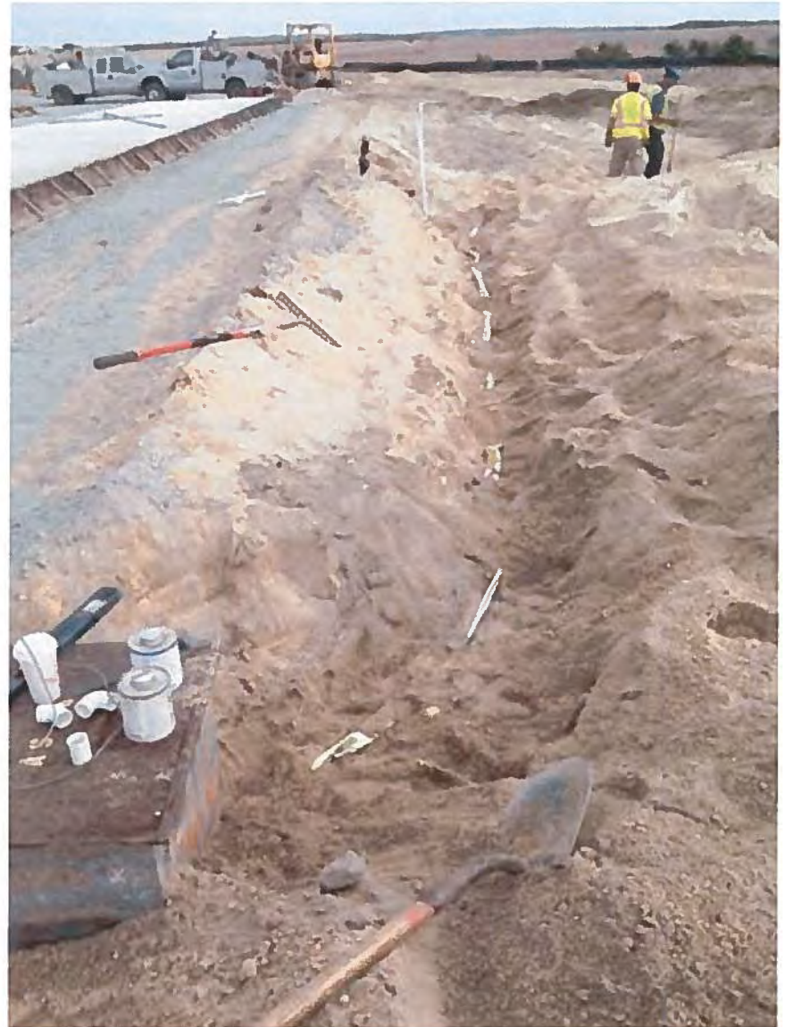
30. Utility Locate Wire Installation at AS-66
