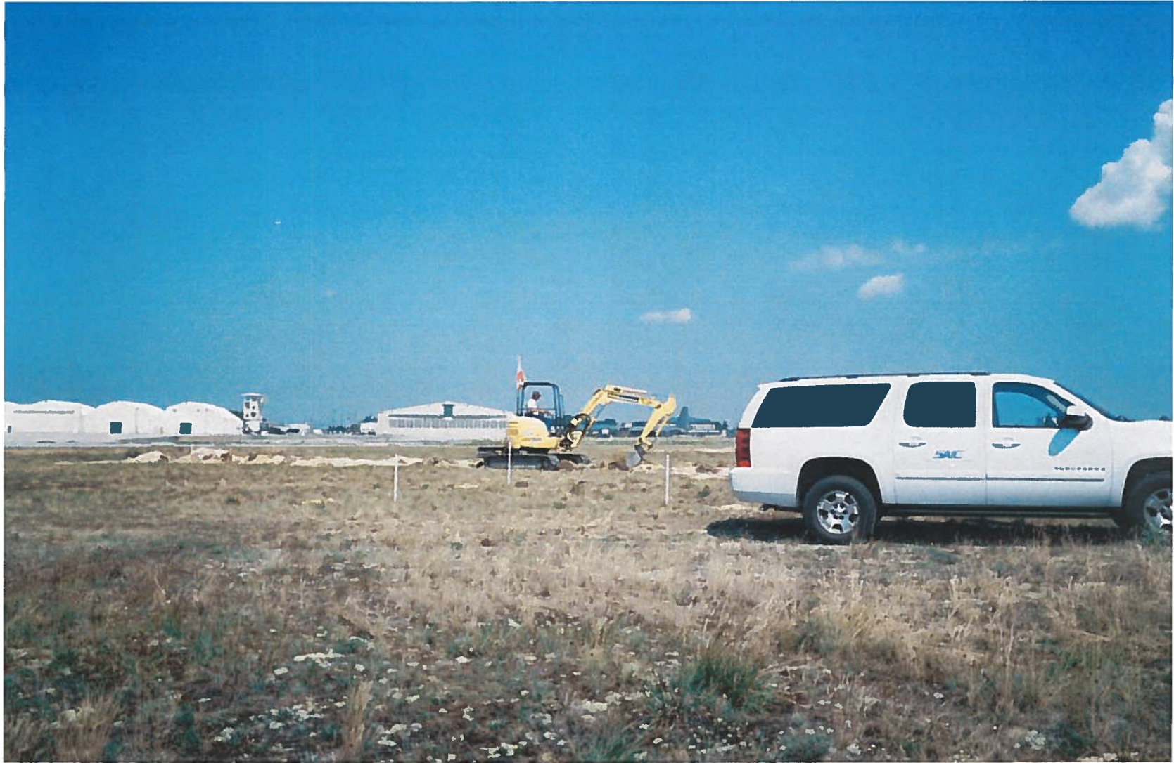
Photo 9. Backhoe Used for Backfilling Air Biosparging System Lines
