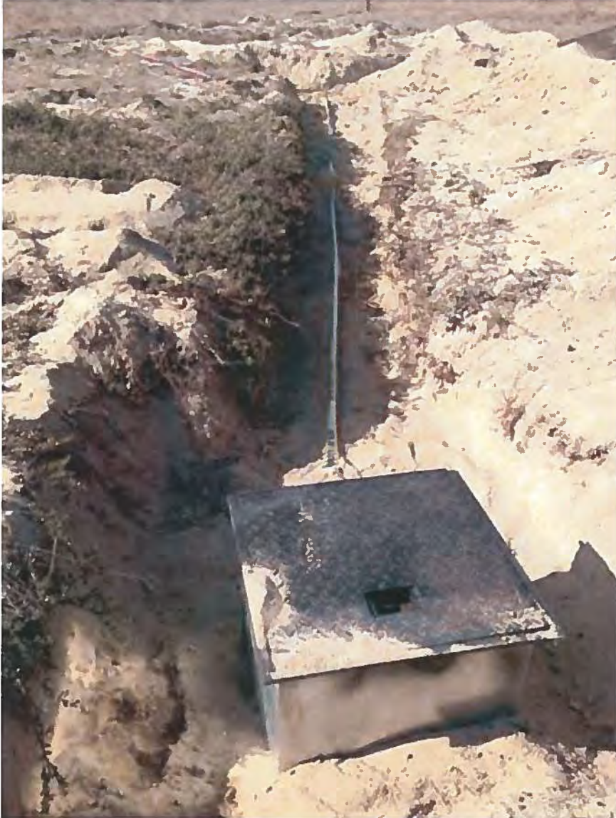
21. Vault Placement at AS-78 Sparge Well
