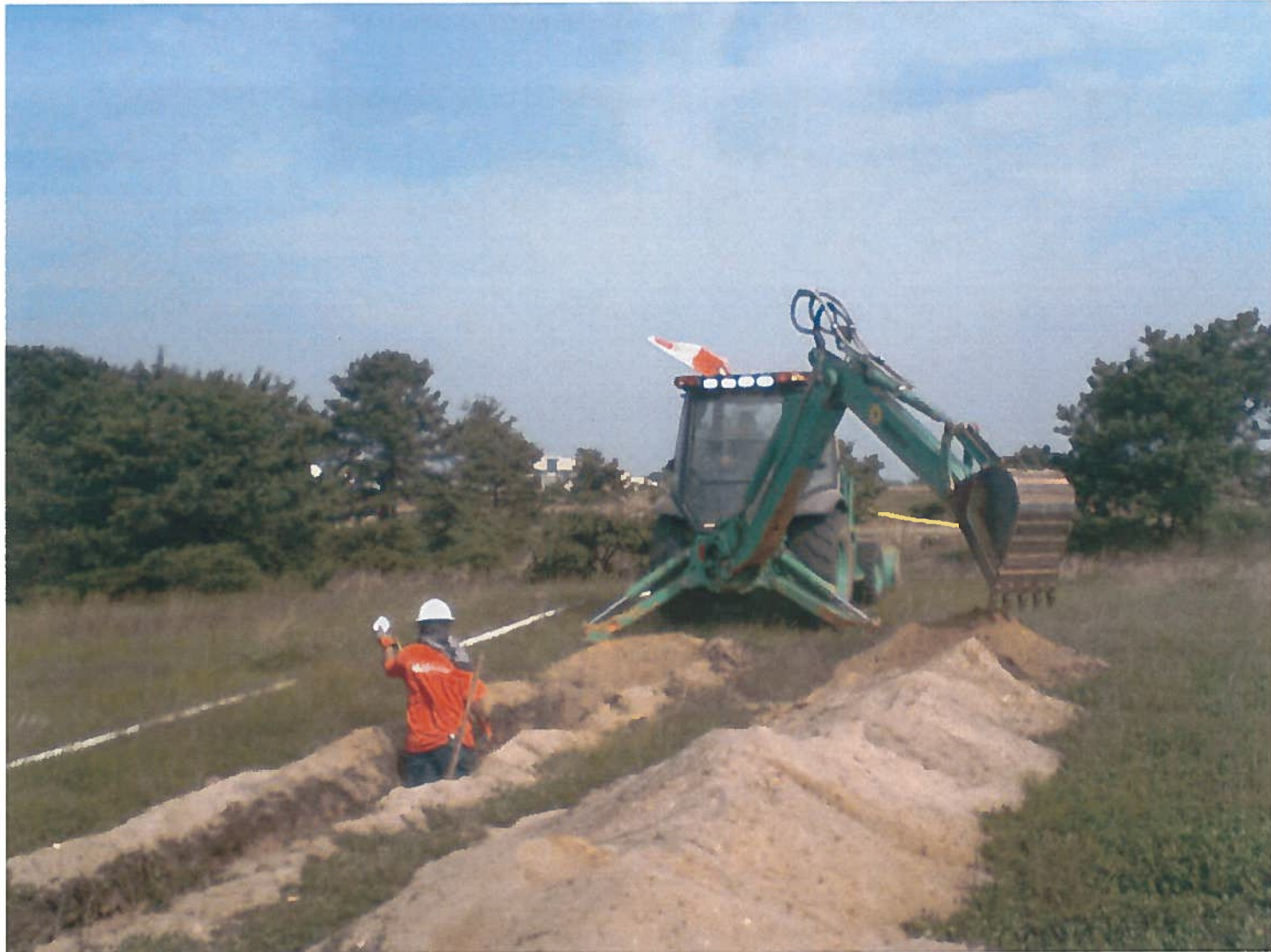
Photo 14. Worker Measures Excavation to Ensure Consistent Depth for Air Supply Line
