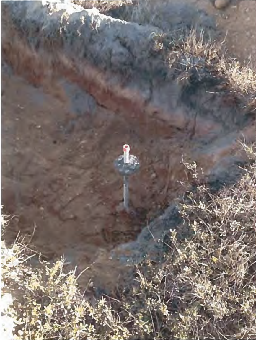
9. Trench to New AS-78 Sparge Well
