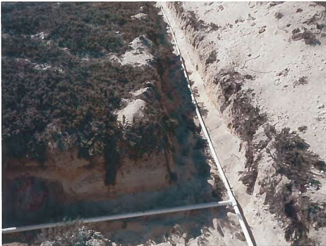
Photo 11: Installation of 1-in Branch Line to New Sparge Wells
