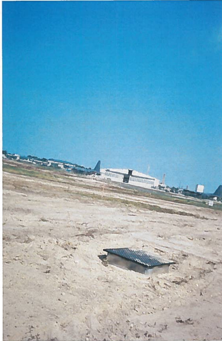
Photo 4. View of Air Biosparging Well Vault Prior to Backfilling Vault Sides
