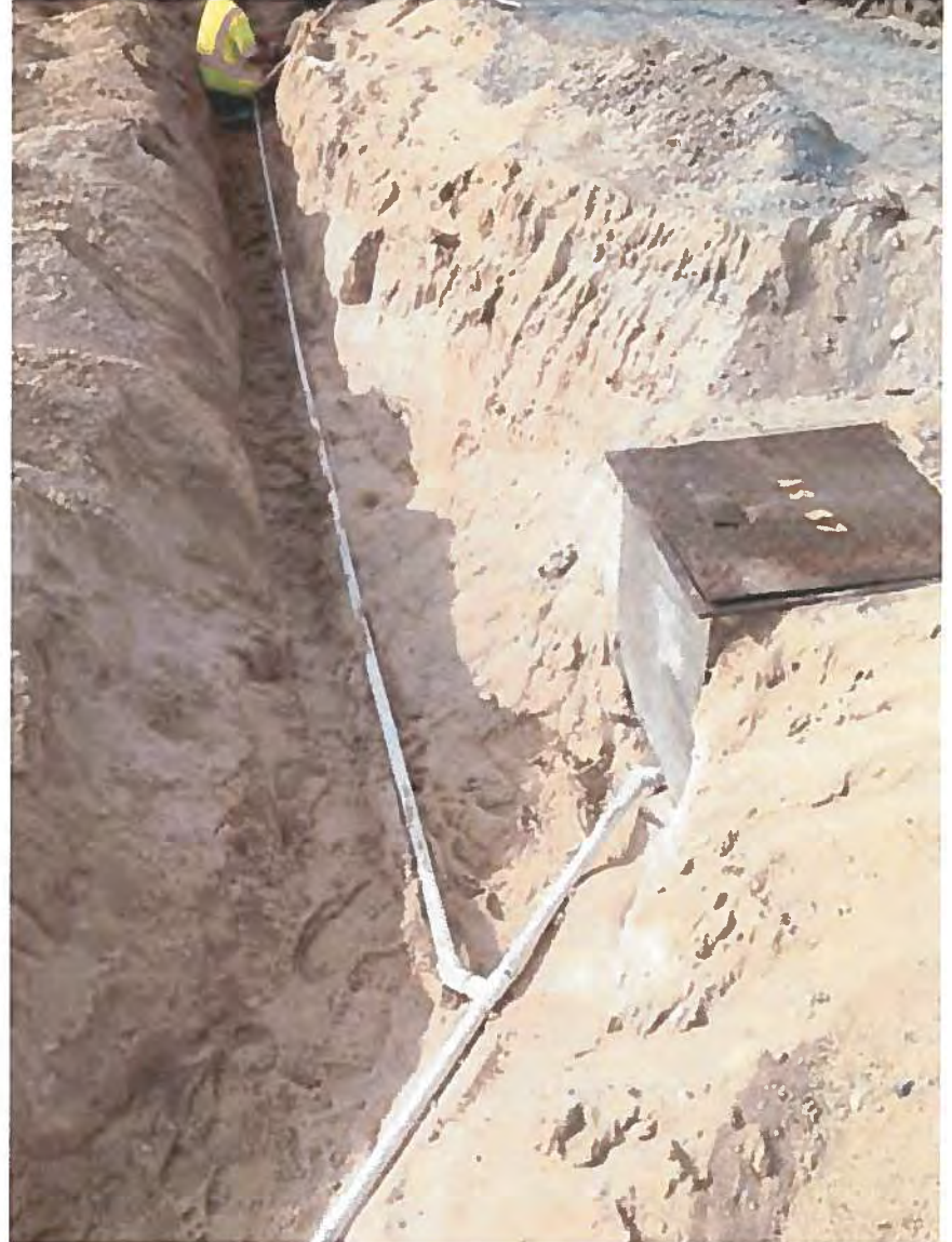
26. PVC Piping Installation to AS-66 and AS-67 Sparge Well
