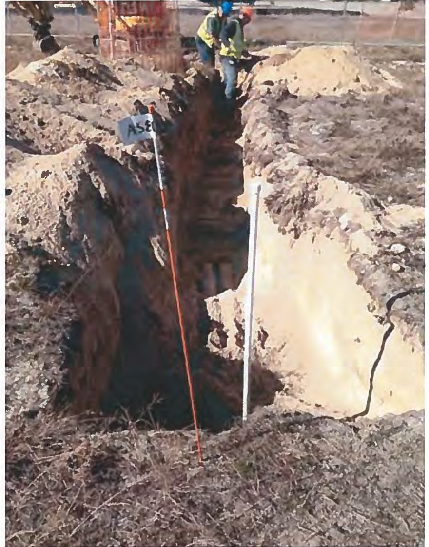
10. Trench to New AS-81 Sparge Well
