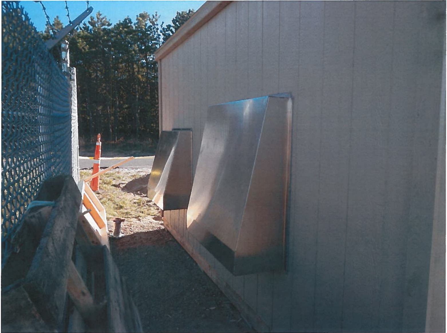
Photo 22 : Vent Hoods Located on Back Side of Storage Shed
