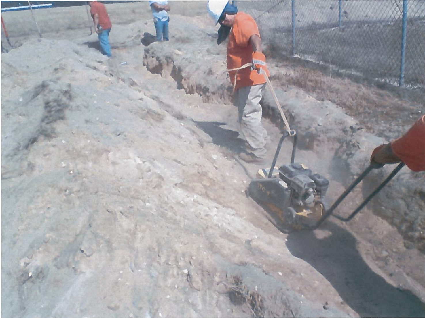
Photo 11. Tamper Used to Achieve Compaction Following Backfilling of System Air Lines
