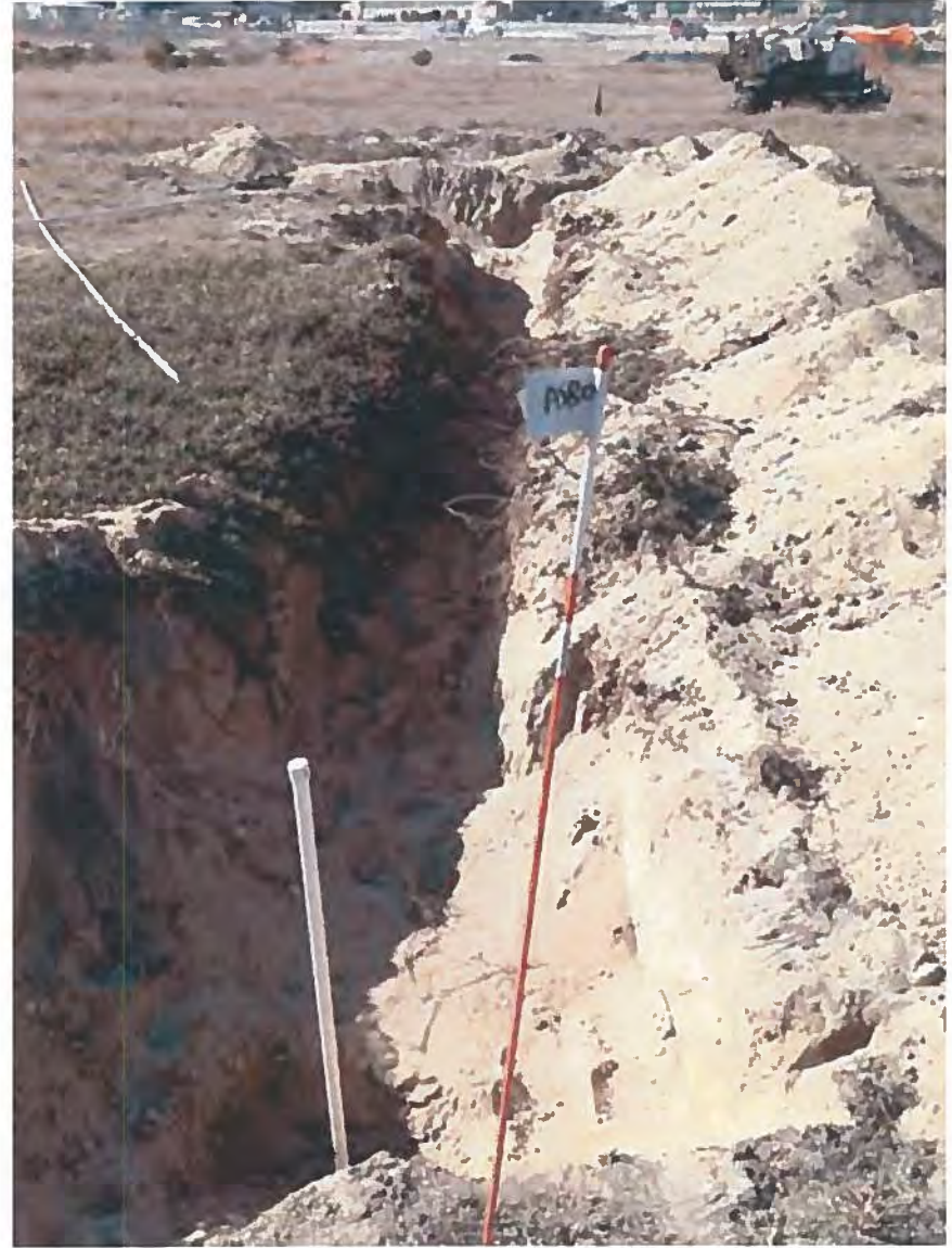
12. Trench to New AS-P2 Sparge Well
