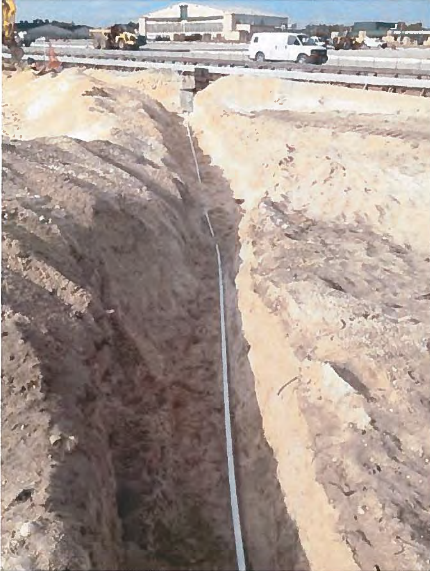
25. PVC Piping Installation to AS-67 Sparge Well
