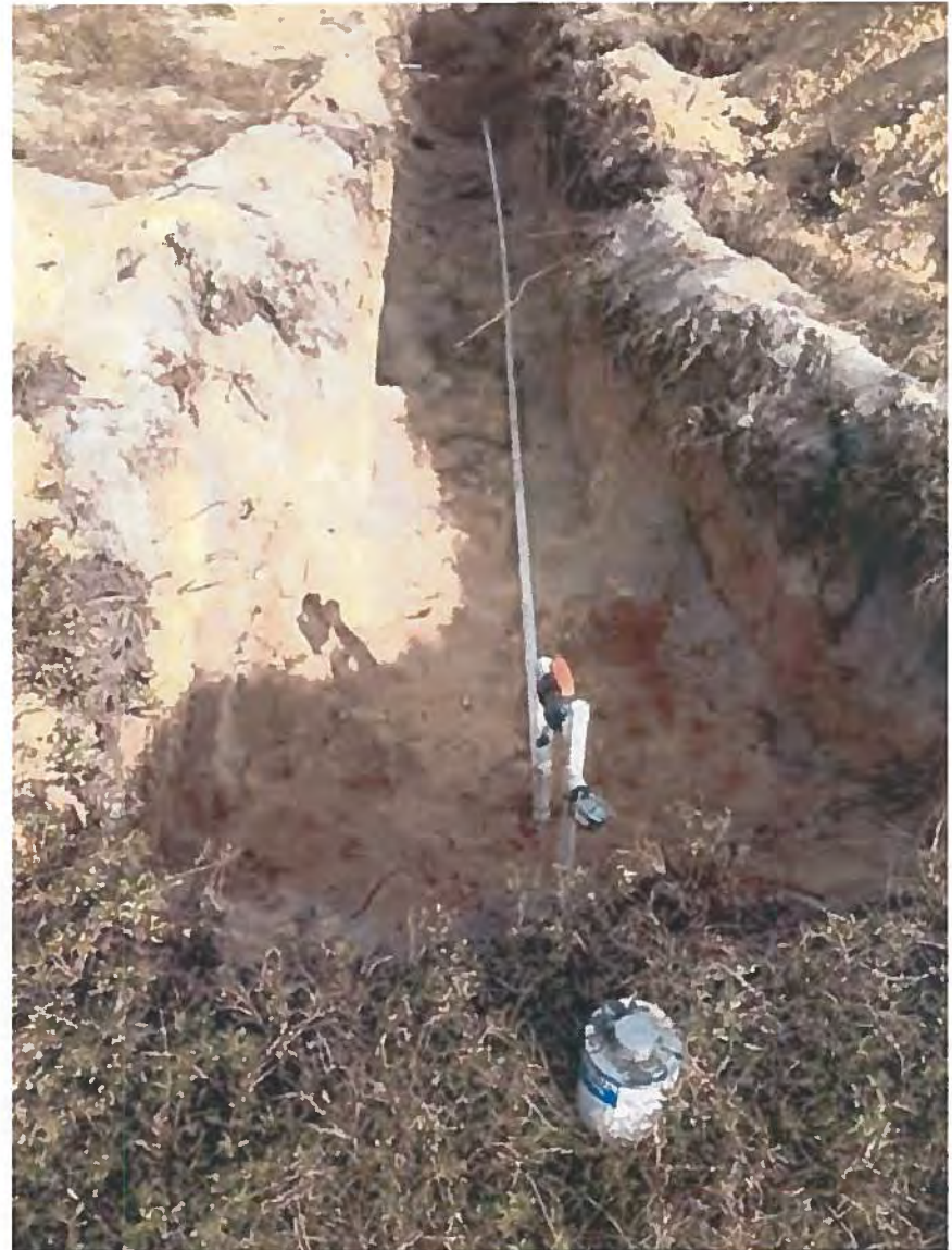
20. PVC Piping Installation at AS-78 Sparge Well
