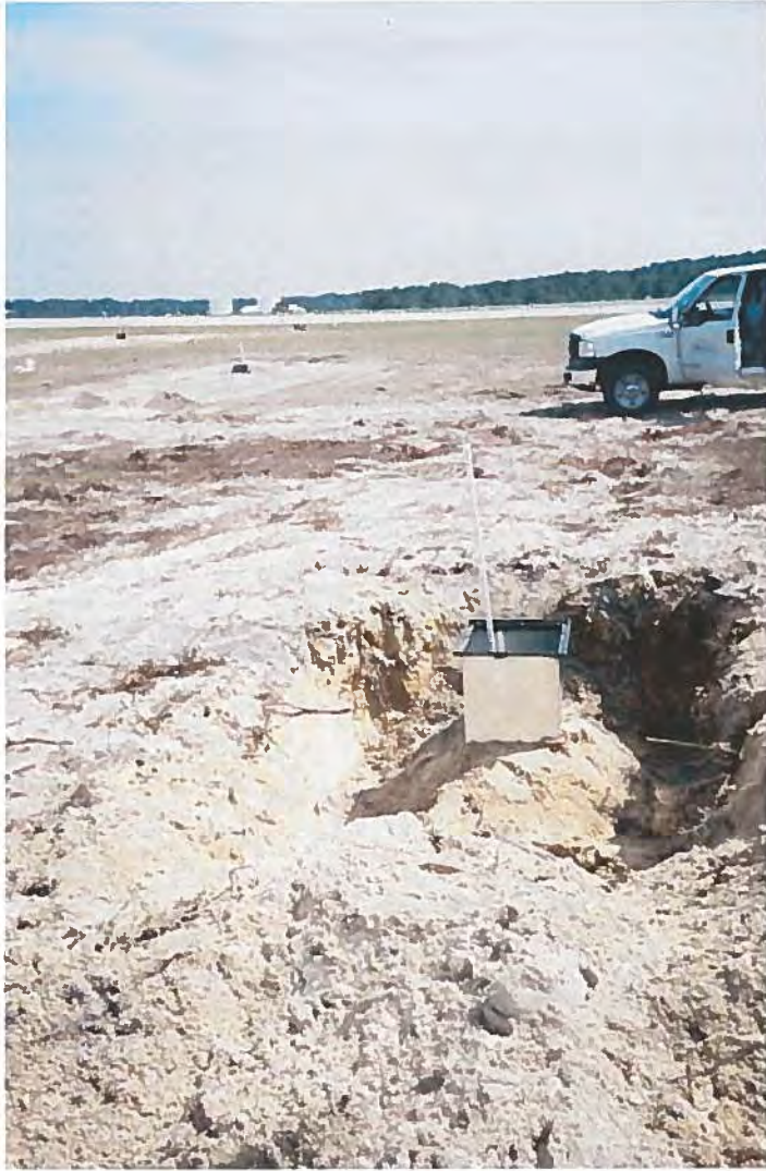
Photo 7. Installation of Air Biosparging Well Vaults Across Site 9
