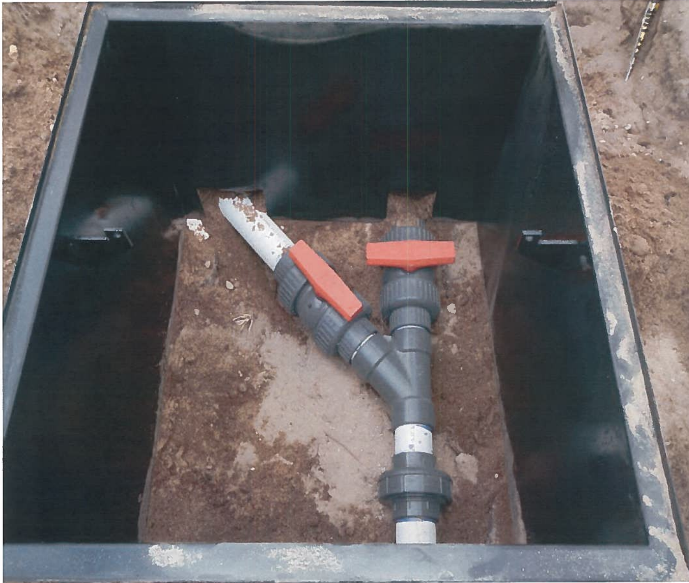
Photo 19: View of Existing and New Trunk Line Connection
