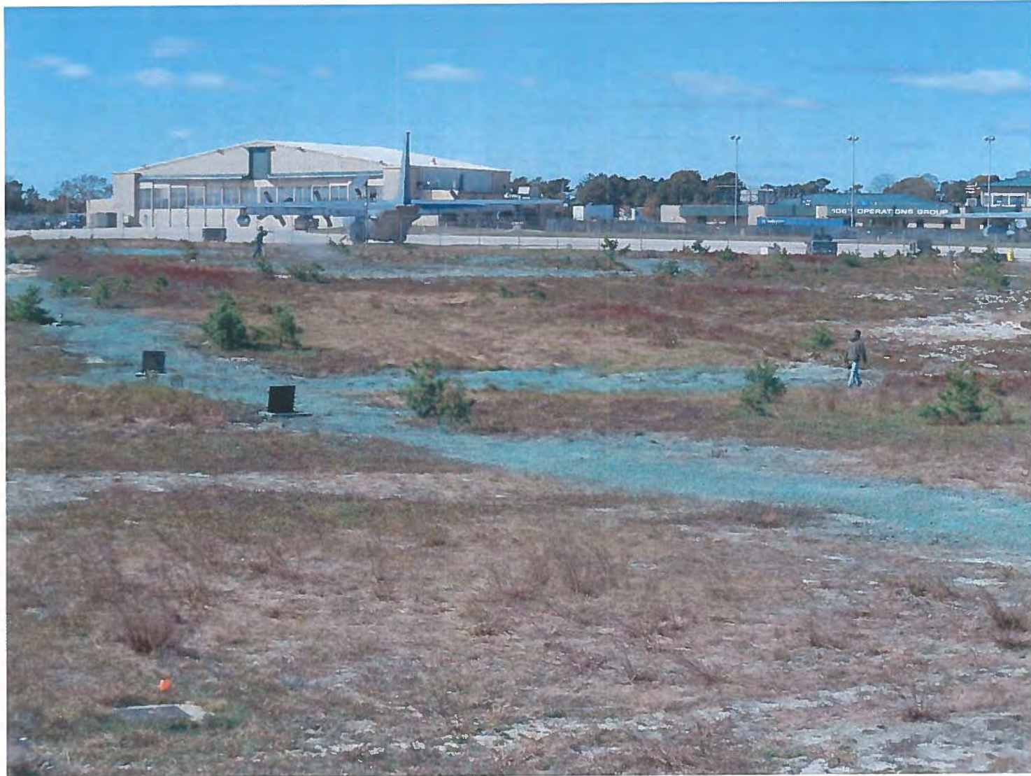
Photo 24: Hydroseeding At Completion
