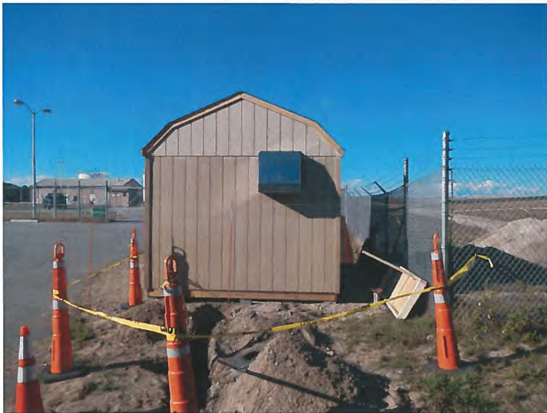
Photo 10: Installation of Electrical Supply Line
