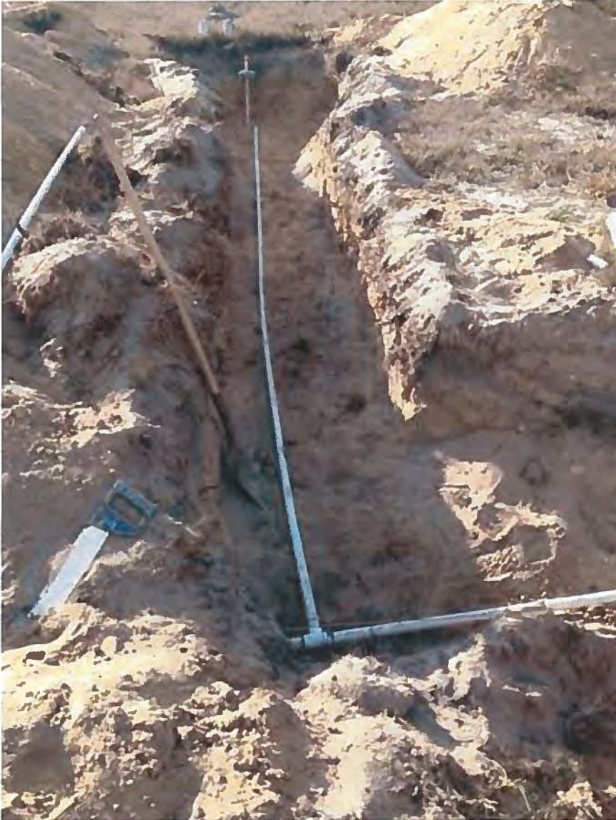
17. PVC Piping Installation to AS-78 Sparge Well
