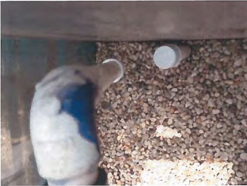
7. PVC Piping Protective Measure Example
