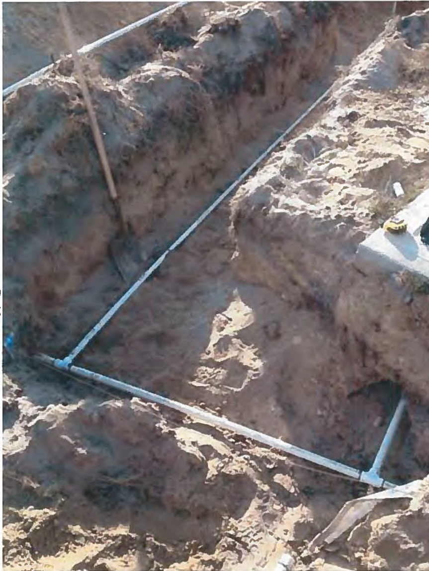
19. PVC Piping Installation to AS-78 and AS-P2 Sparge Well
