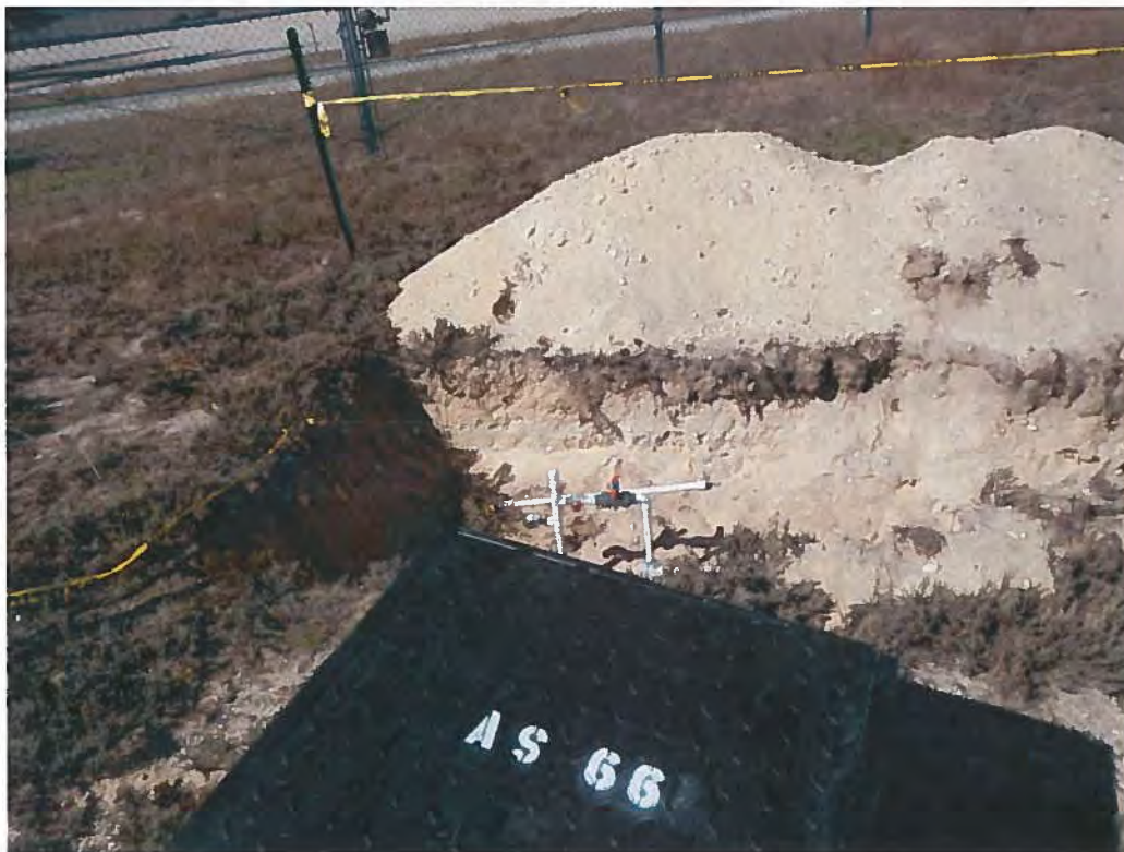
Photo 12: Installation of New Biosparge Well Completion
