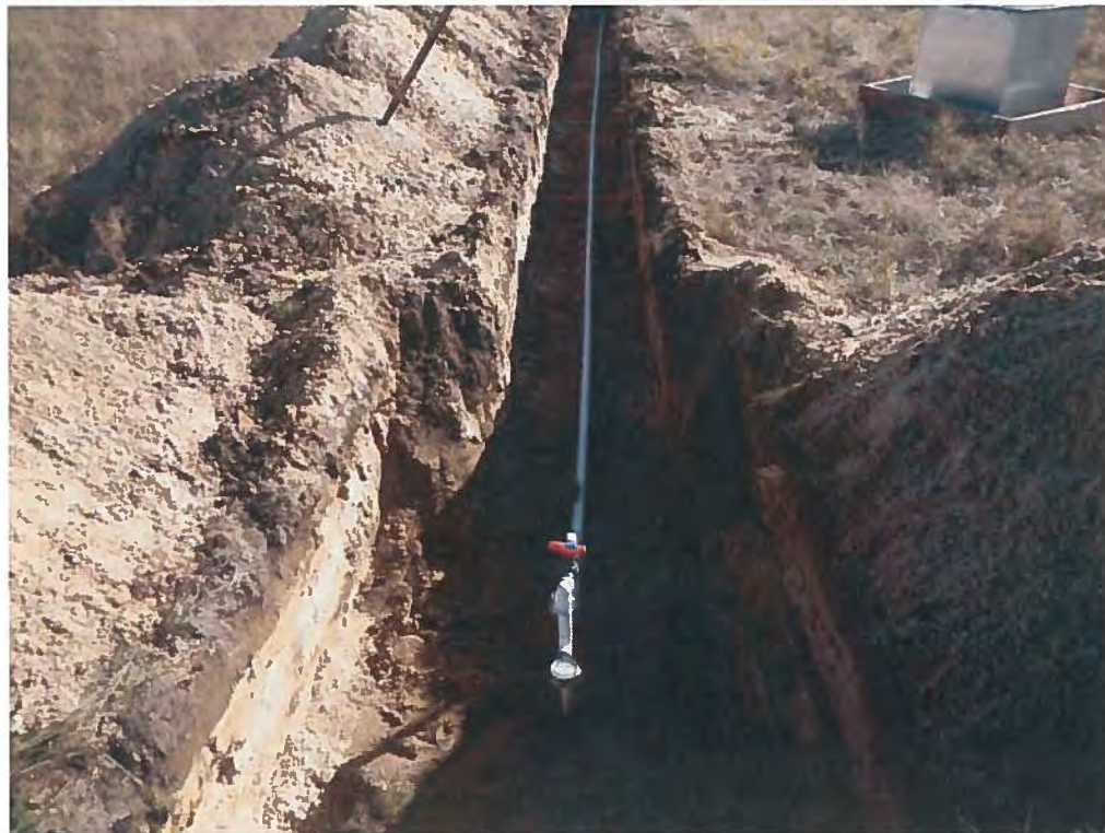
Photo 6: Installation of New Biosparge Well Completion
