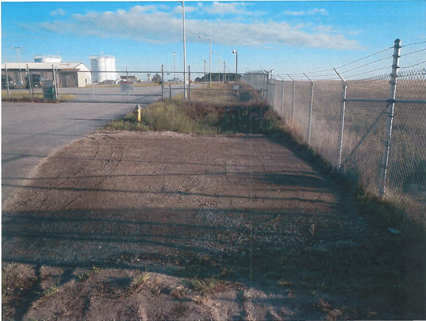
Photo 2: Installation of Compacted Base Layer Prior to Shed Installation
