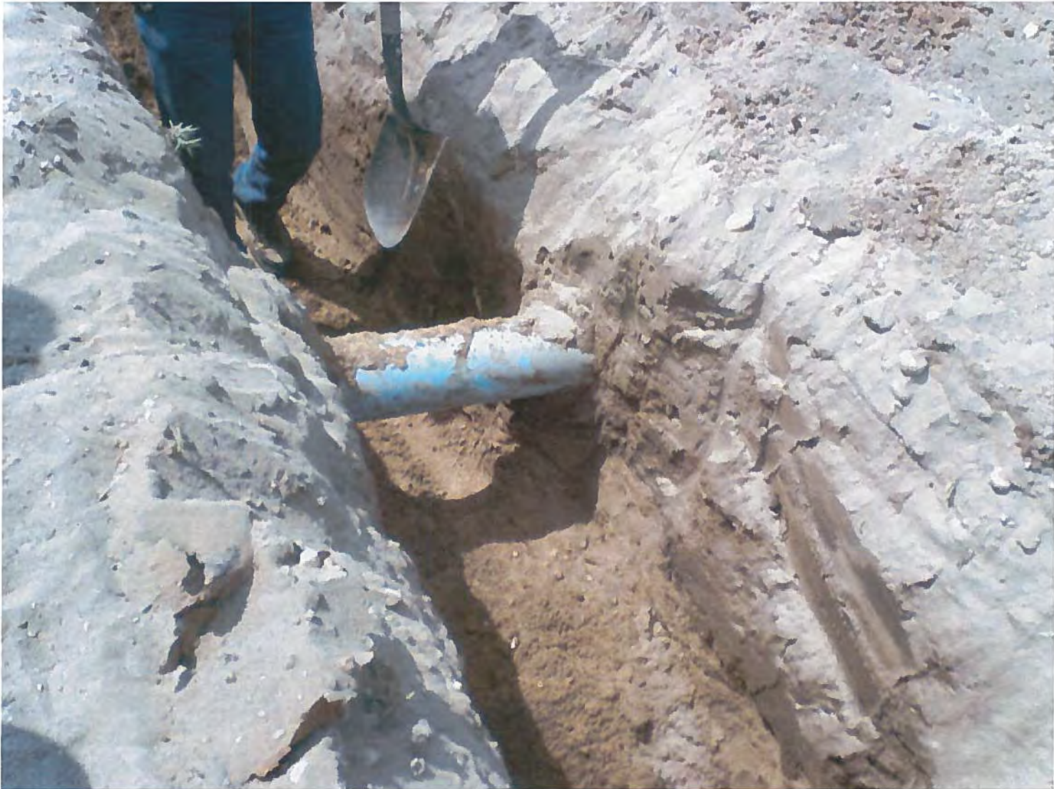
Photo 15. Hand Clearance of Septic Line While Crossing Road in Site 9 Vicinity
