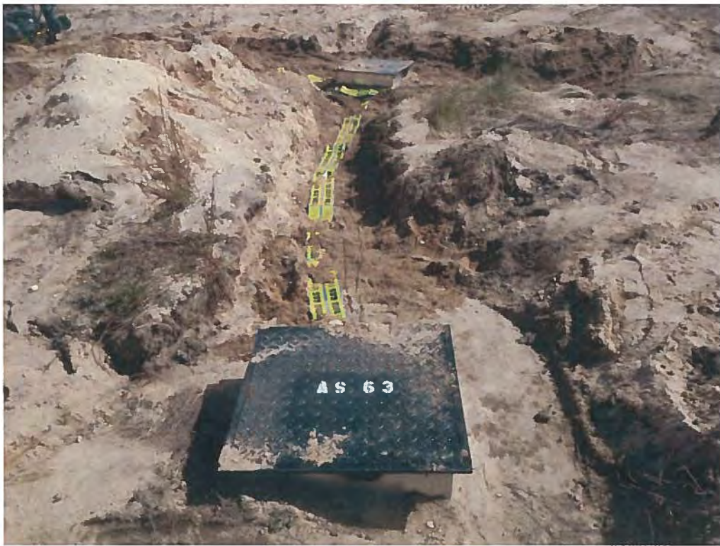
Photo 8: Installation of Sparge Vault with Utility Tape and Locator Wire
