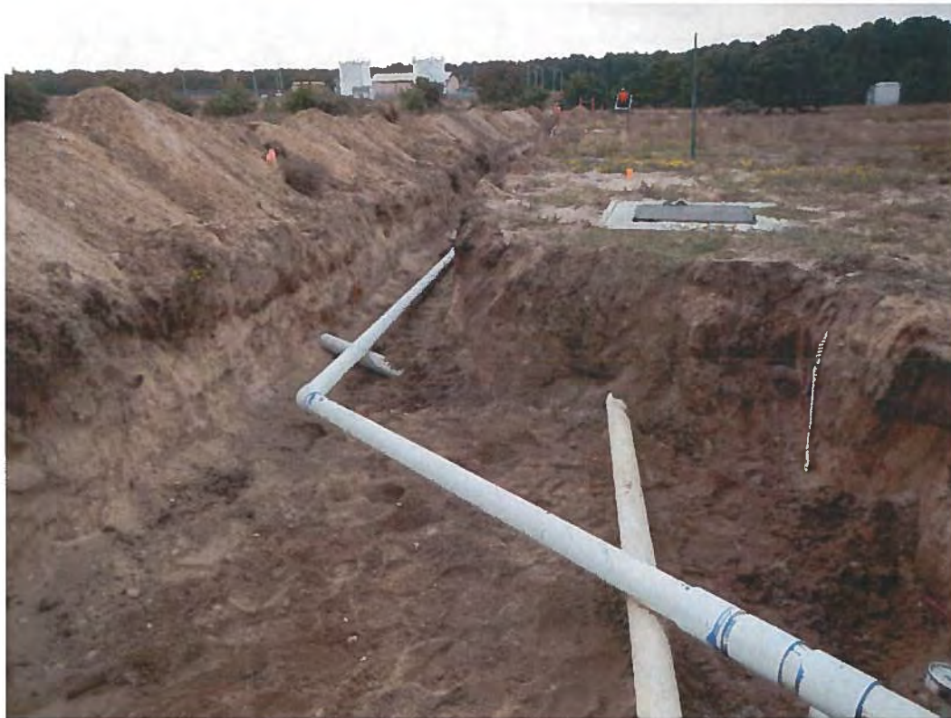
Photo 5: Pressure Testing of 3-in Trunk Line (Top) and Trunk Line North
