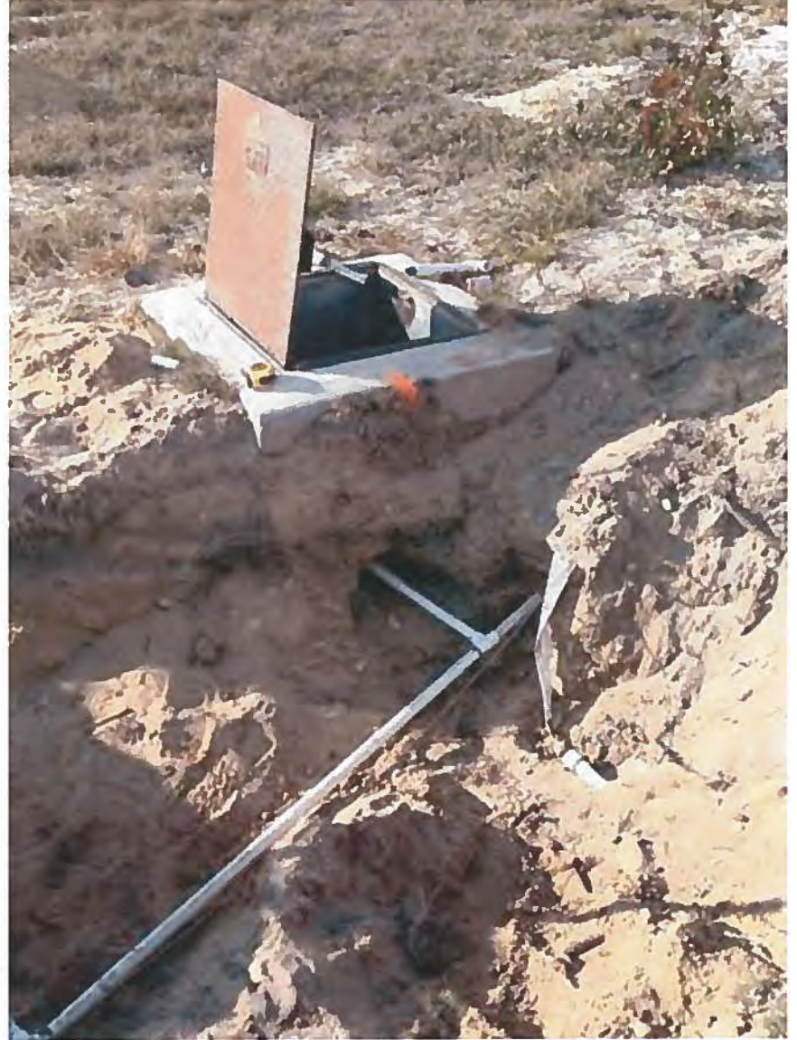
18. PVC Piping Installation at AS-P2 Sparge Well
