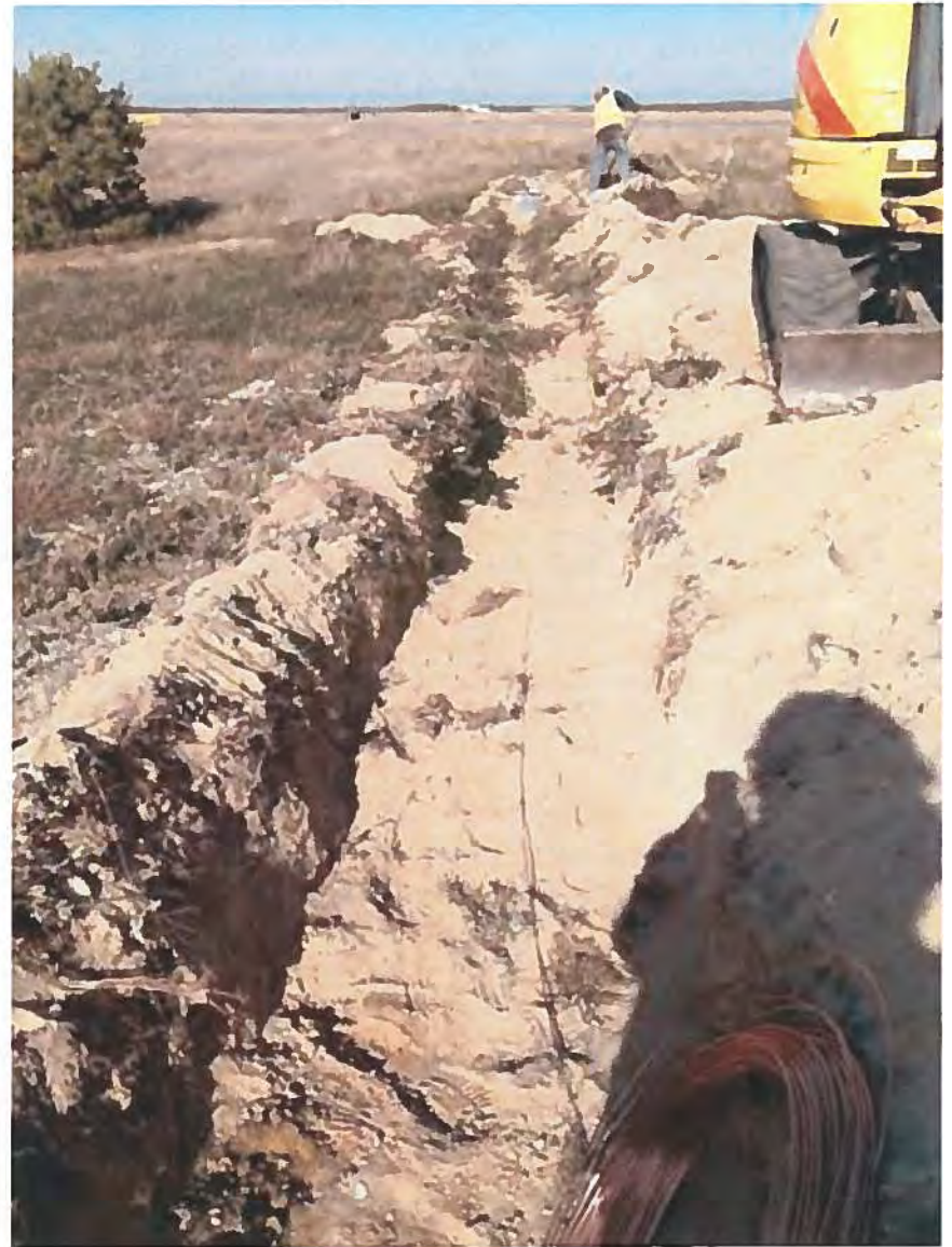
14. Utility Locate Wire Installation
