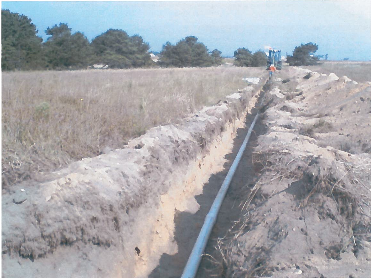
Photo 12. Installation of Main Air Supply Line Across Site 9
