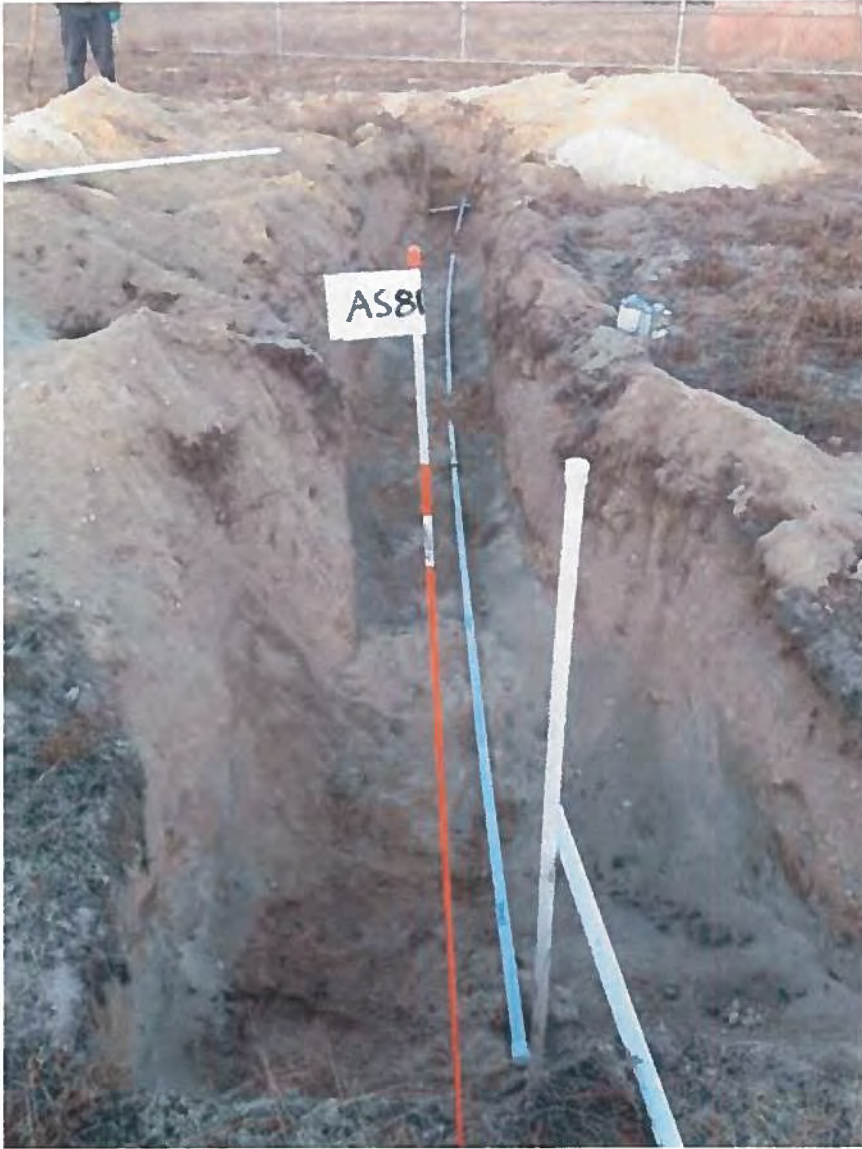
15. PVC Piping Installation to AS-81 Sparge Well
