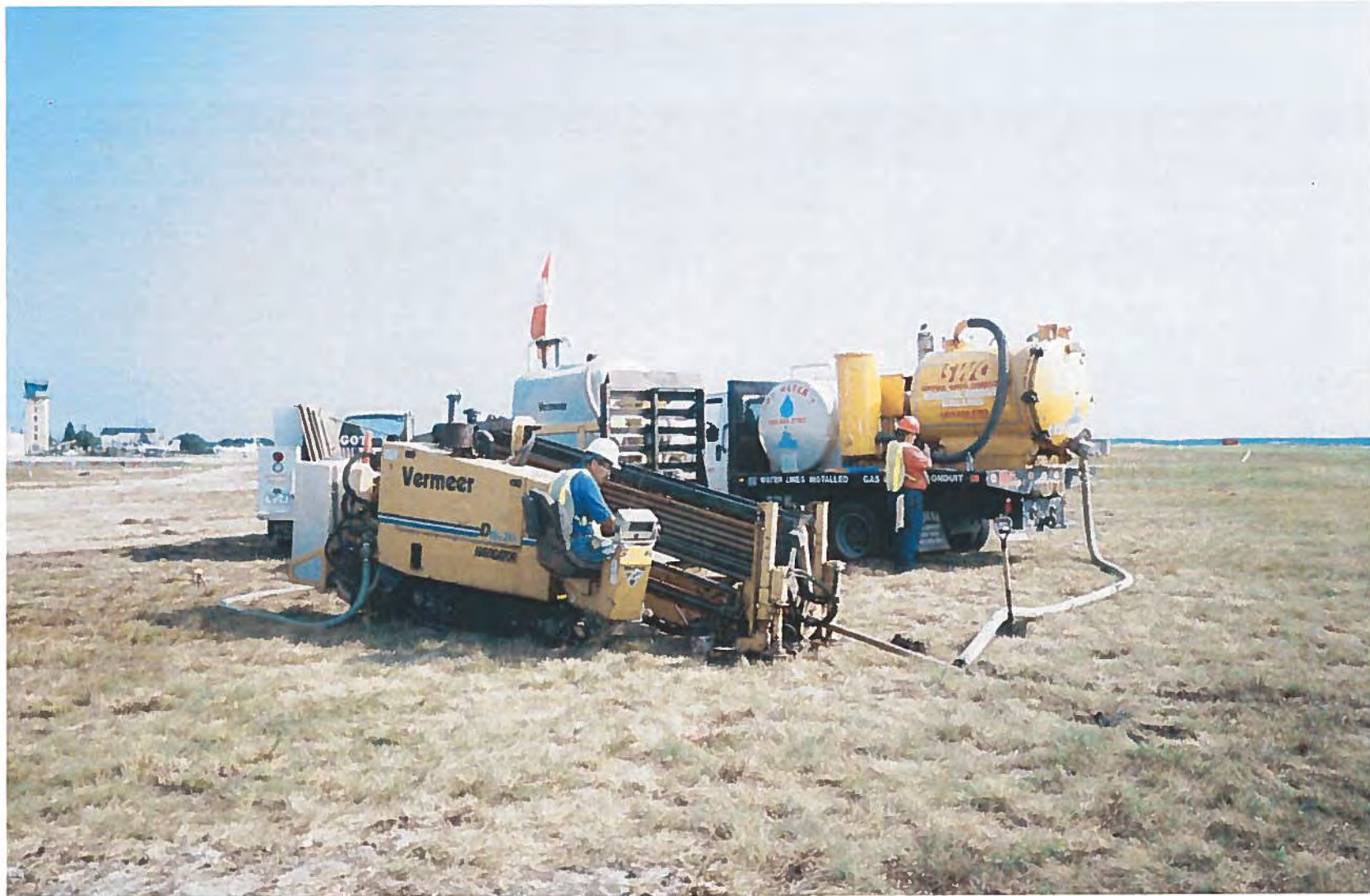
Photo 5. Directional Well Drill Rig Creating Borehole for Main Air Supply Line Beneath the High Speed Taxiway
