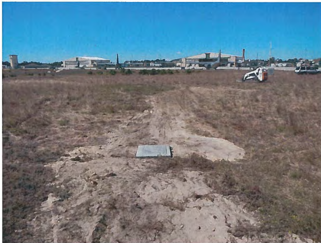
Photo 9: View of a Typical Sparge Vault at Completion
