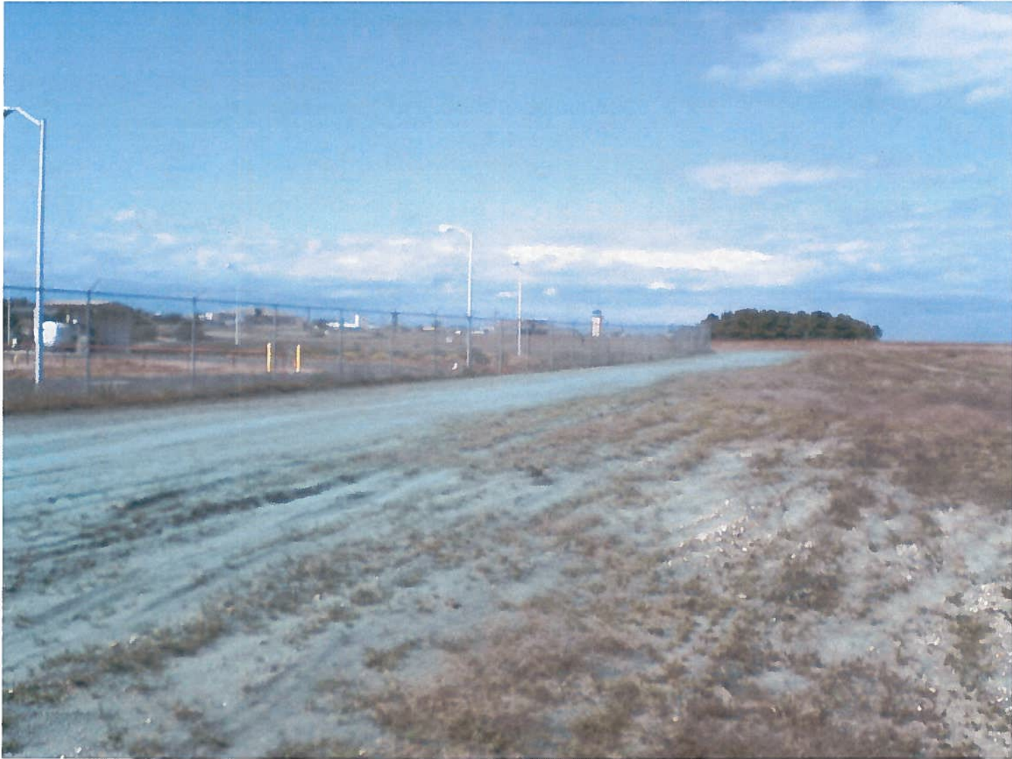
Photo 21. Main Air Supply Run Following Raking, Seeding, and Hydro-Mulching
