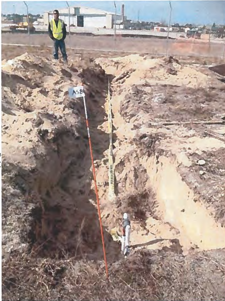
23. Utility Locate Wire Installation at AS-81
