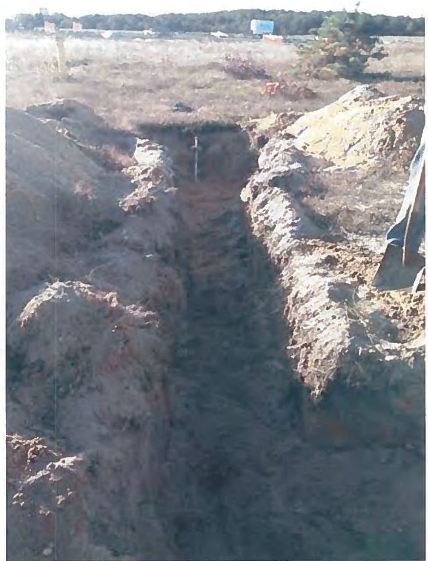
8. Trench to New AS-78 Sparge Well
