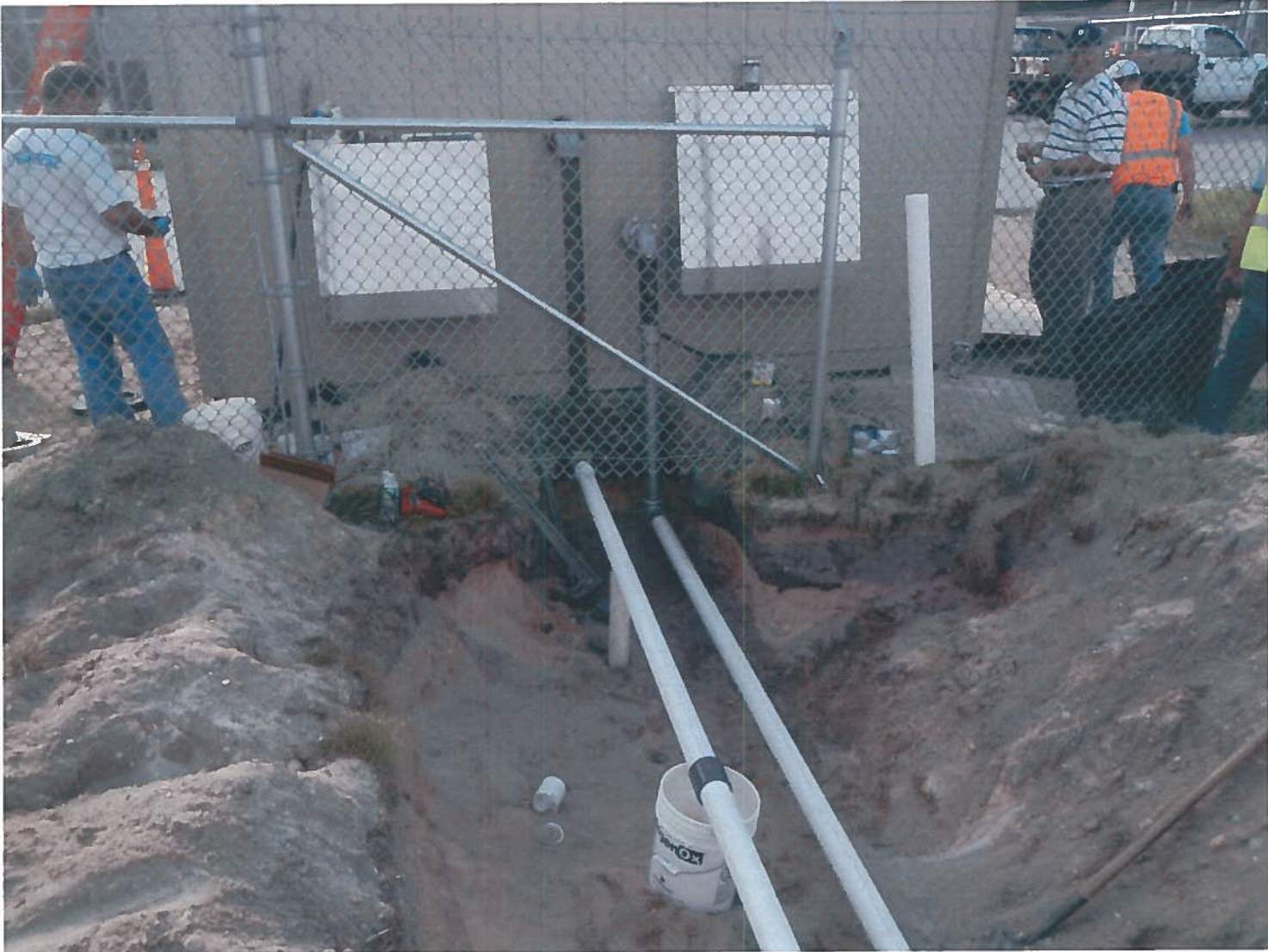
Photo 23: New and Existing Sparge Lines Into Storage Shed
