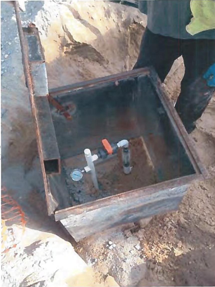
27. Vault Placement at AS-66 Sparge Well
