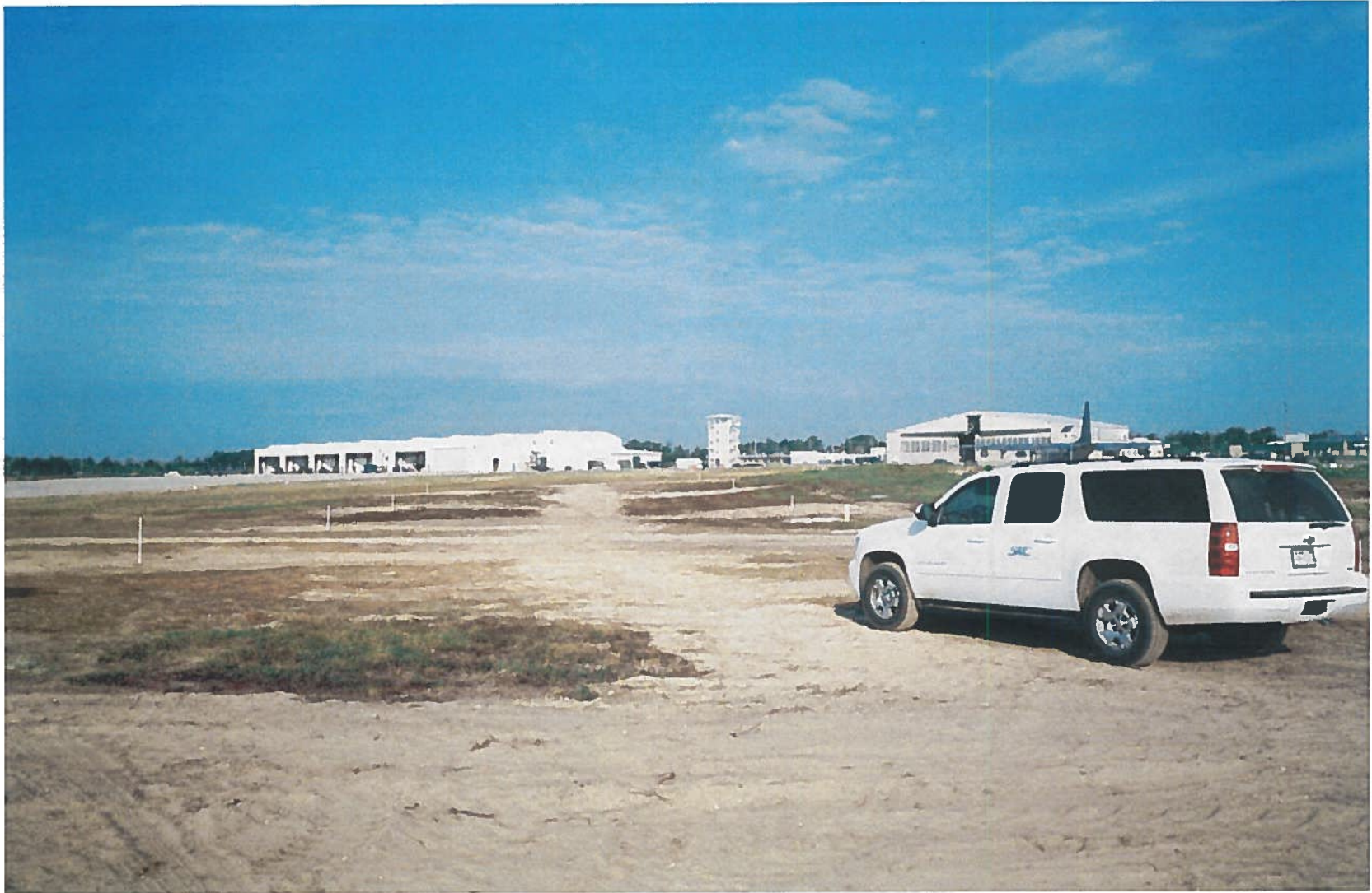
Photo 2. View of Backfilled System Lines Across Site 4
