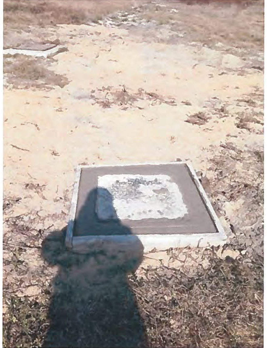
22. Concrete Placement at AS-78 Sparge Well
