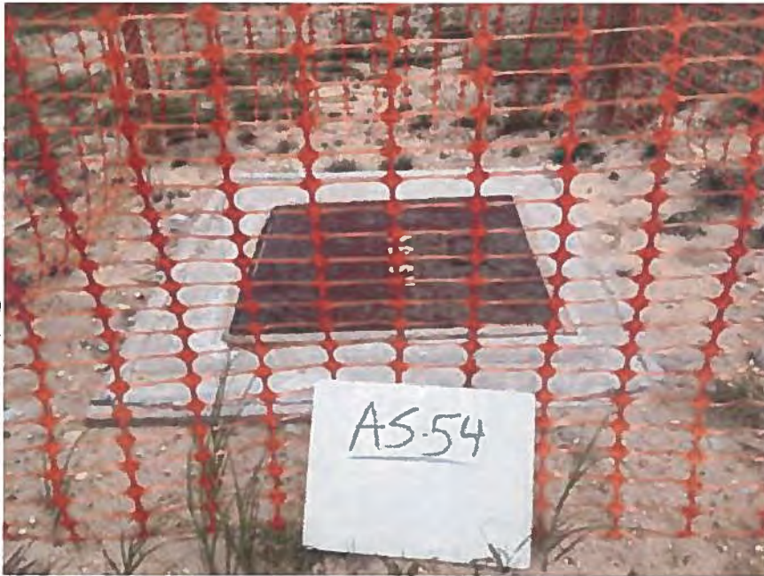
3. Valve Vault Protective Measure Example
