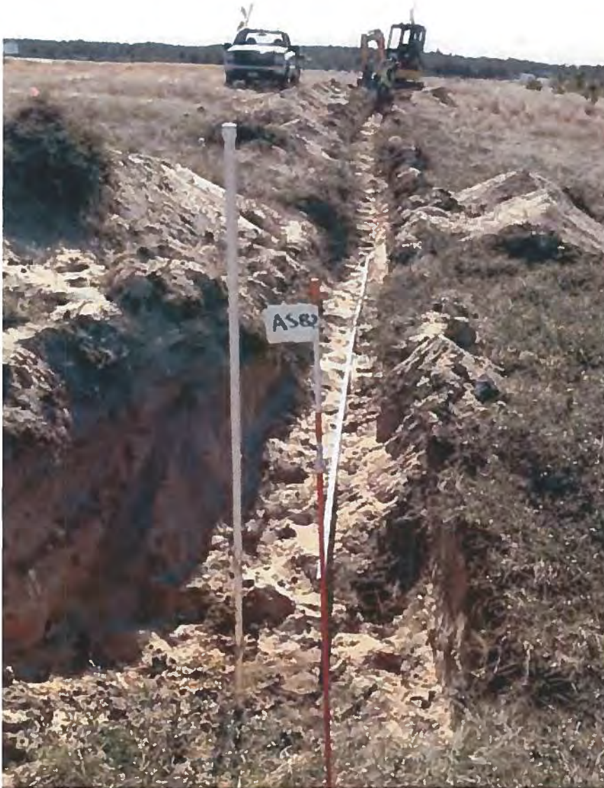
13. Trench to New AS-P2 Sparge Well
