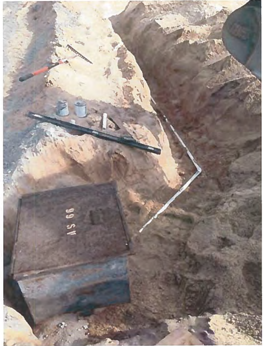
28. Vault Placement at AS-66 Sparge Well
