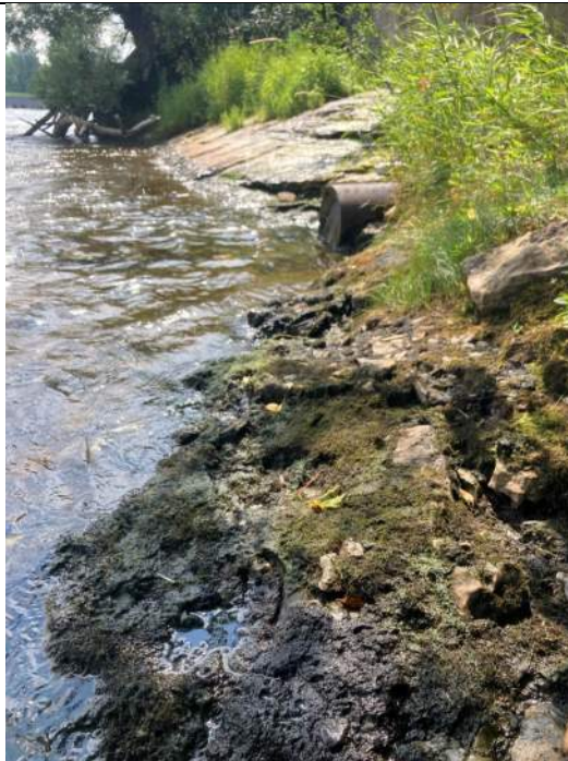
Photograph #5 (7/12/22) – Area of S4/S5 deposit. View looking upstream (southeast). Plugged 15" diameter outfall pipe in background.
