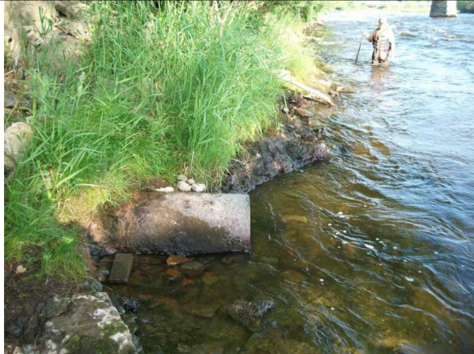
Photograph #4 – Area of S4 deposit. View toward downstream direction (6/18/10). Plugged 15” diameter outfall pipe in foreground. Hard tar visible downstream of pipe along water edge.
