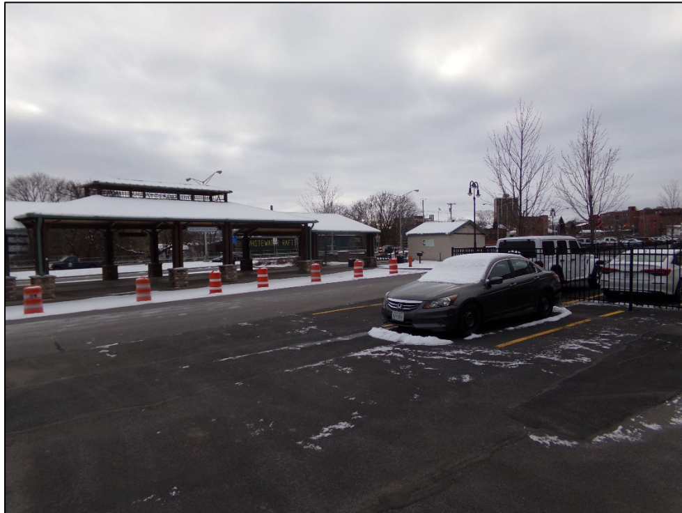
Site Conditions on March 21, 2024
