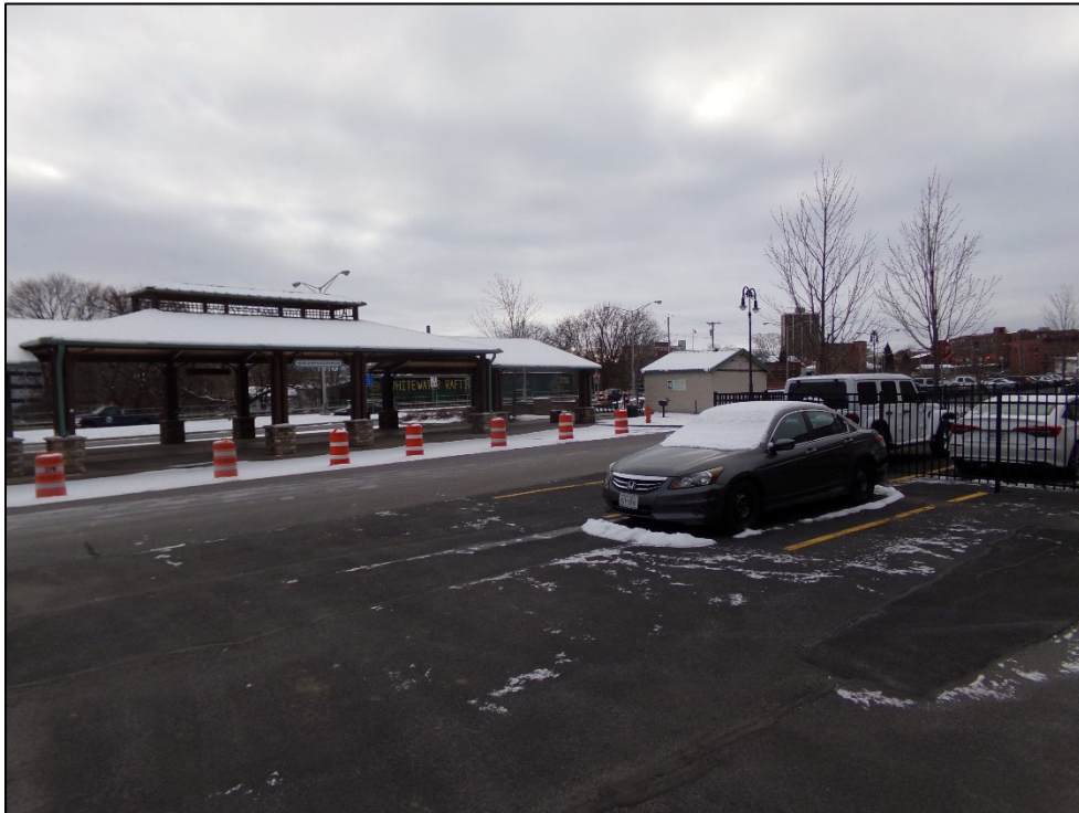
Site Conditions on March 21, 2024
