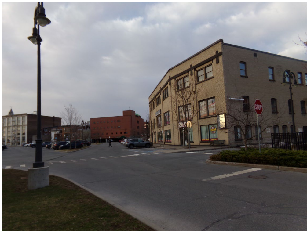
Site Conditions on March 20, 2025
