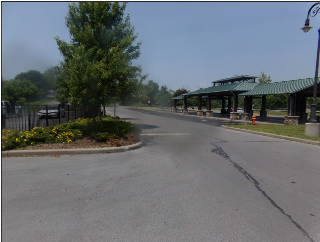
Site Conditions on June 12, 2025
