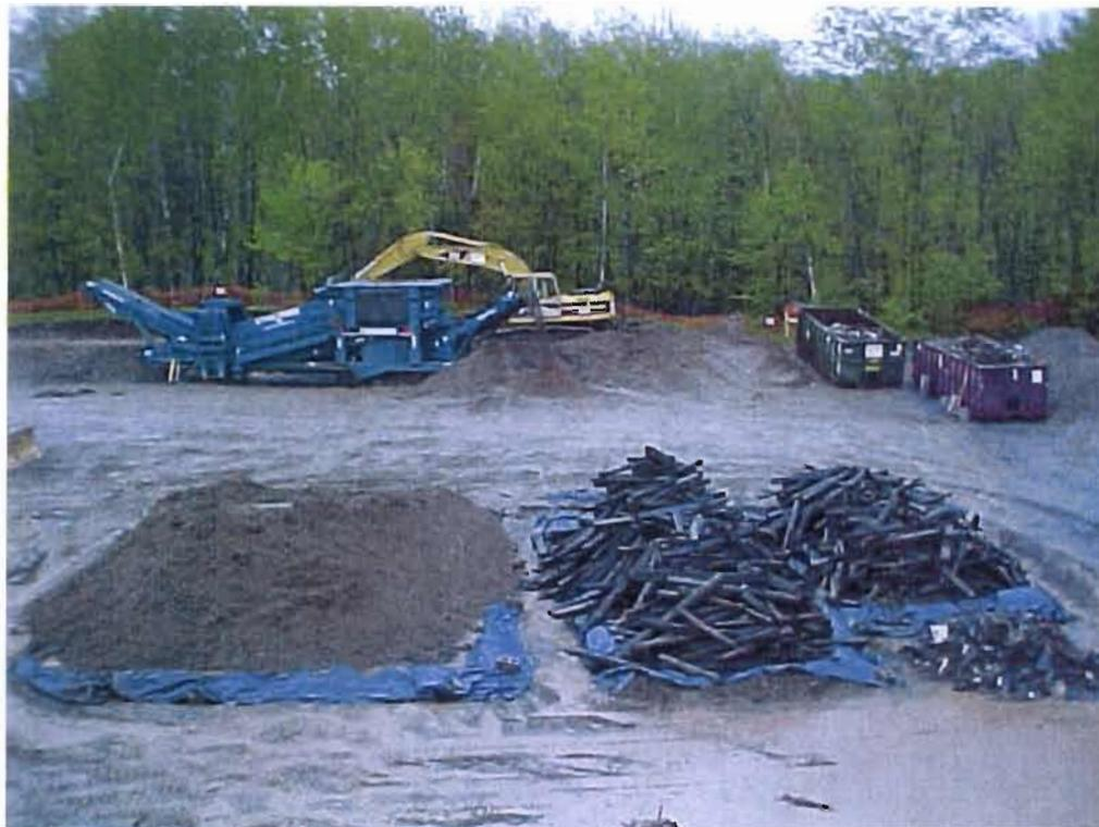
Excavation, power screening, soil stockpiles and wood stockpiles.
