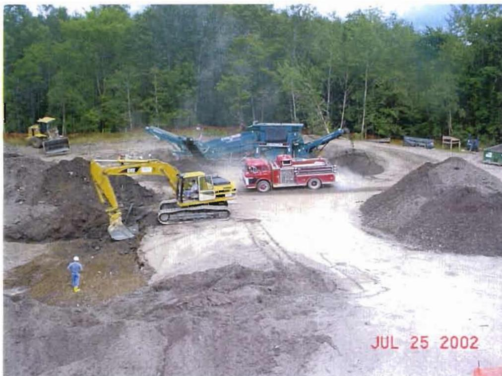
Excavation, power screening, stockpiling. Fire truck used for dust control.
