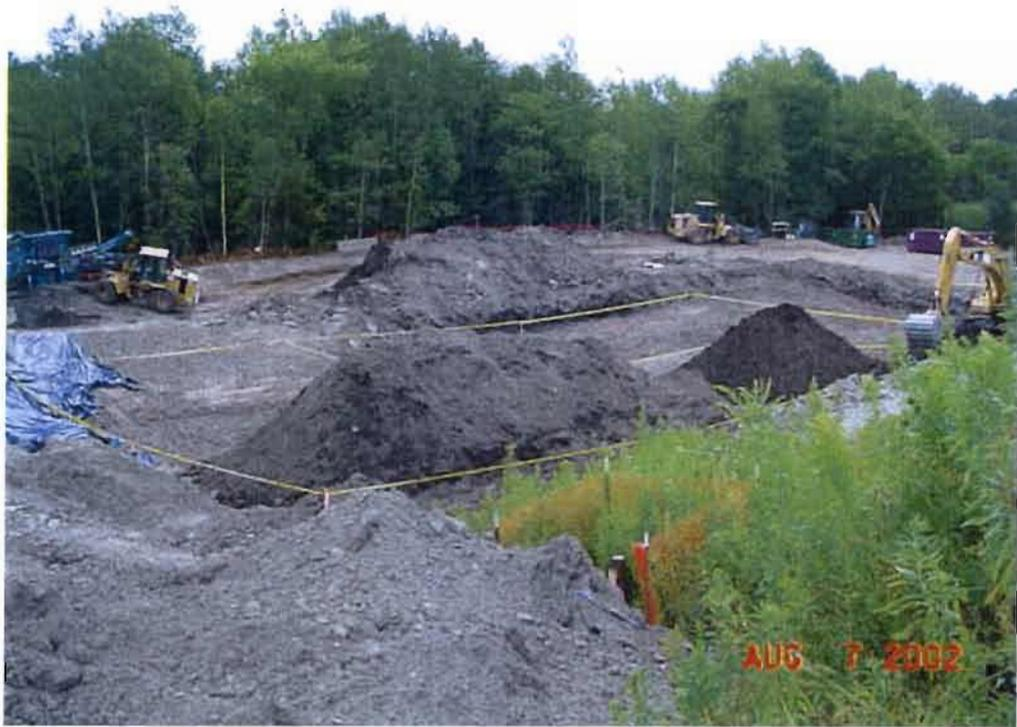
Clean soil obtained from screening, prior to use as backfill. Note poly to demarcate landfill 1.
