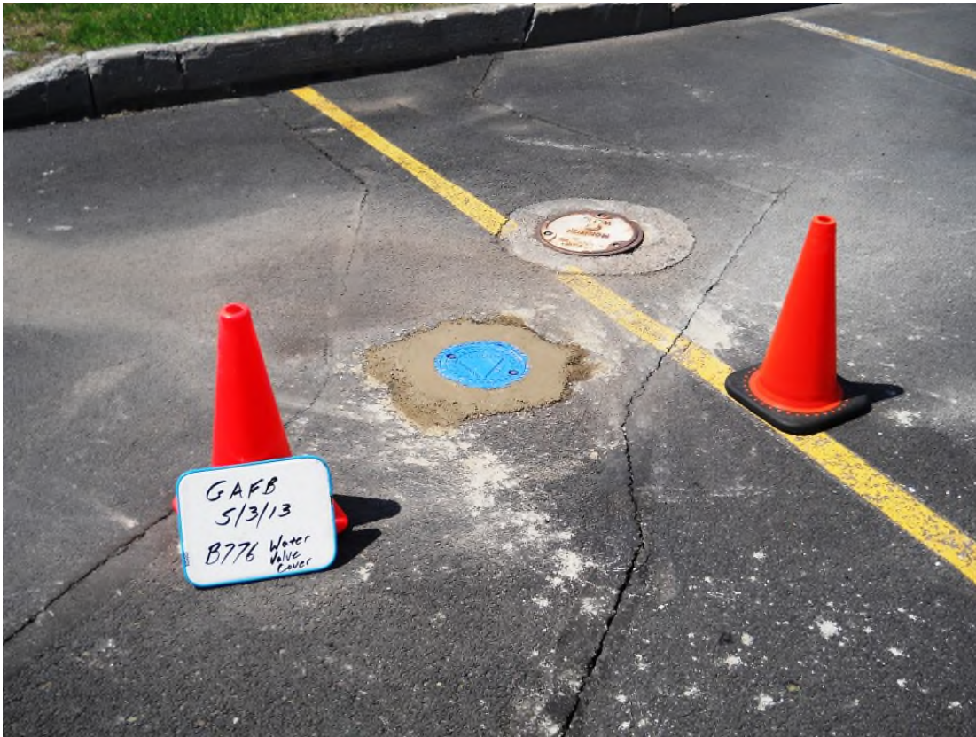
Bldg. 775 Water Cover replaced
