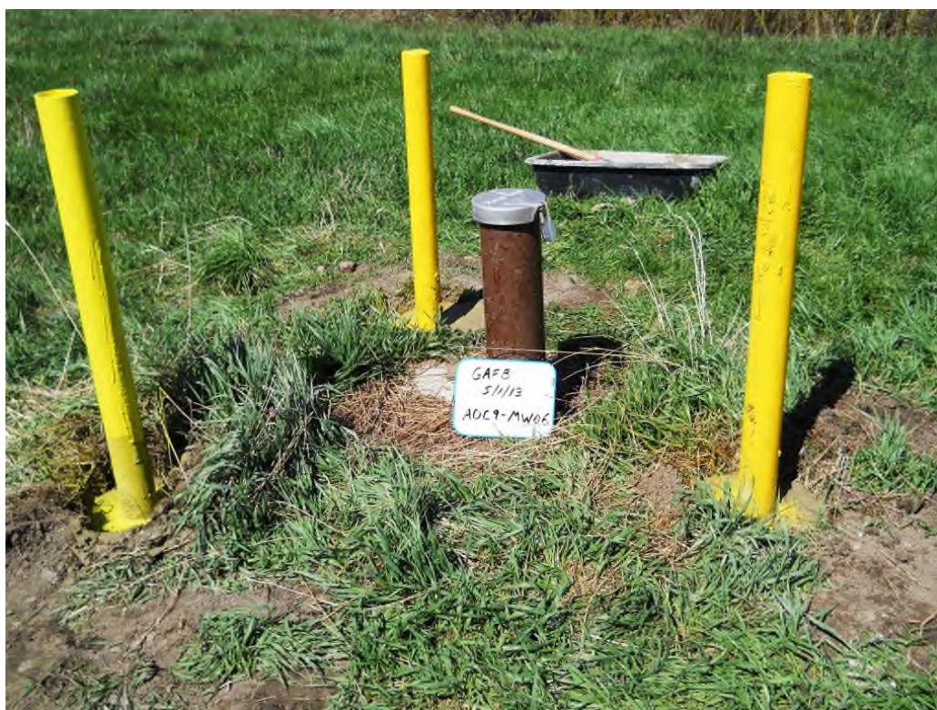
GAFB AOC9 MW-06 Before and after maintenance items
