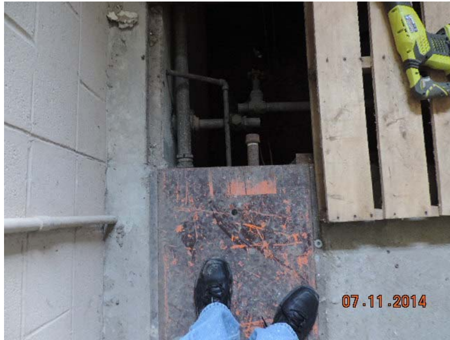
View of B817 sump and line breach to facilitate smoke test.
