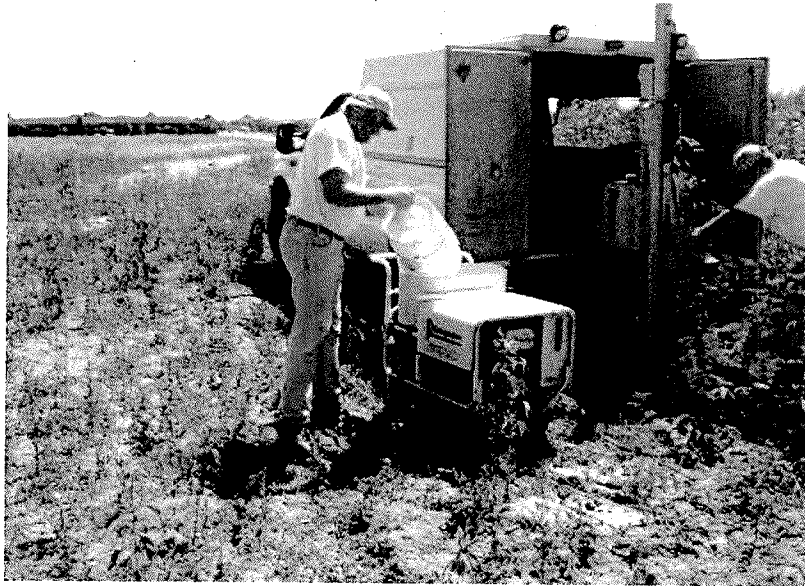
Figure 3: PERMEOX Injection Set Up
