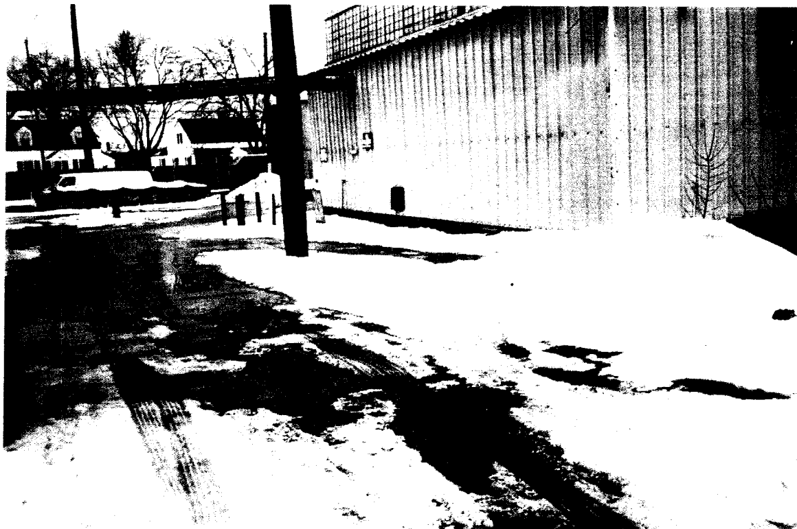
LOOKING WEST AT AREA #2 - PRIOR TO REMEDIATION
