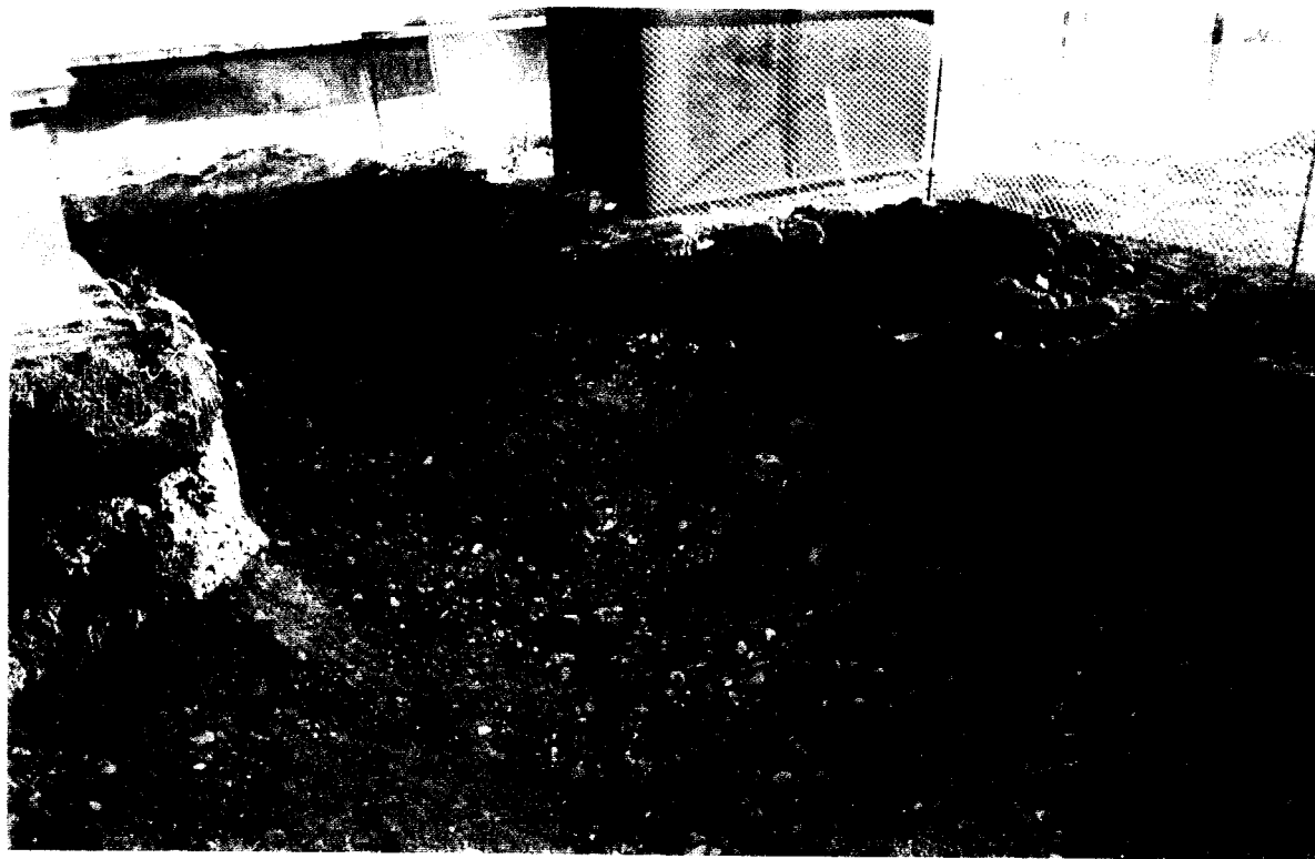
LOOKING NORTH AT EXCAVATION OF AREA #3
