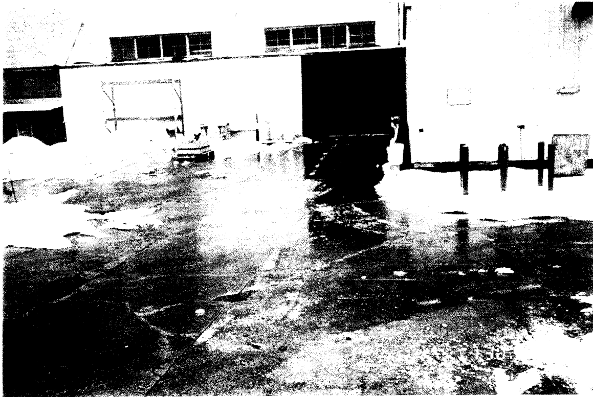
LOOKING NORTH AT AREA #1 - PRIOR TO REMEDIATION
