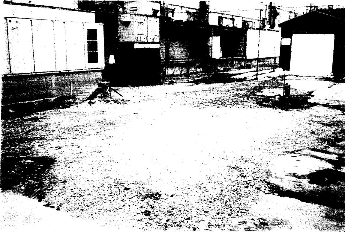
BACKFILLED AREA #2 AND AREA #3 - LOOKING NORTHEAST
