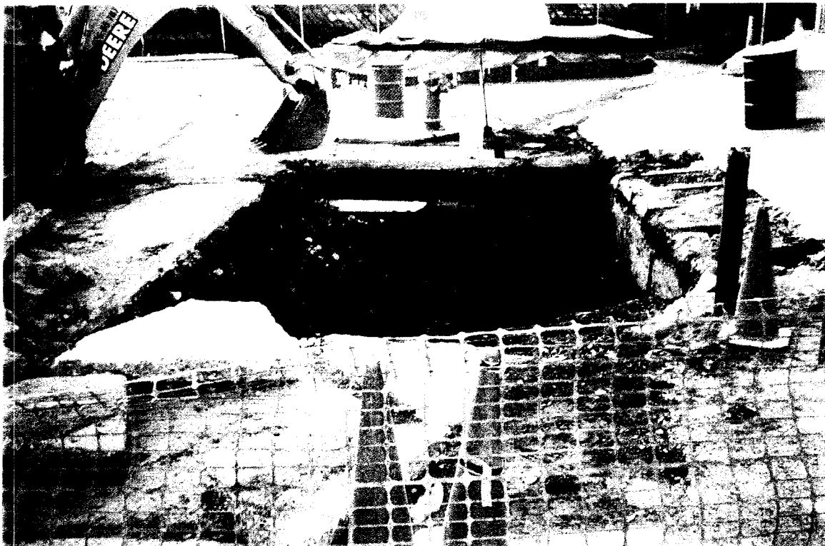
LOOKING WEST AT EXCAVATION OF AREA #1
