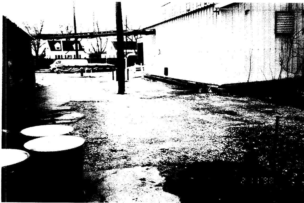
BACKFILLED AREA #2 - LOOKING WEST
