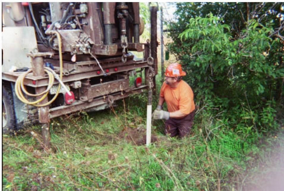
Modification and Decommissioning of Monitoring Wells Looking north from Former Test Building location on 9/12/05
