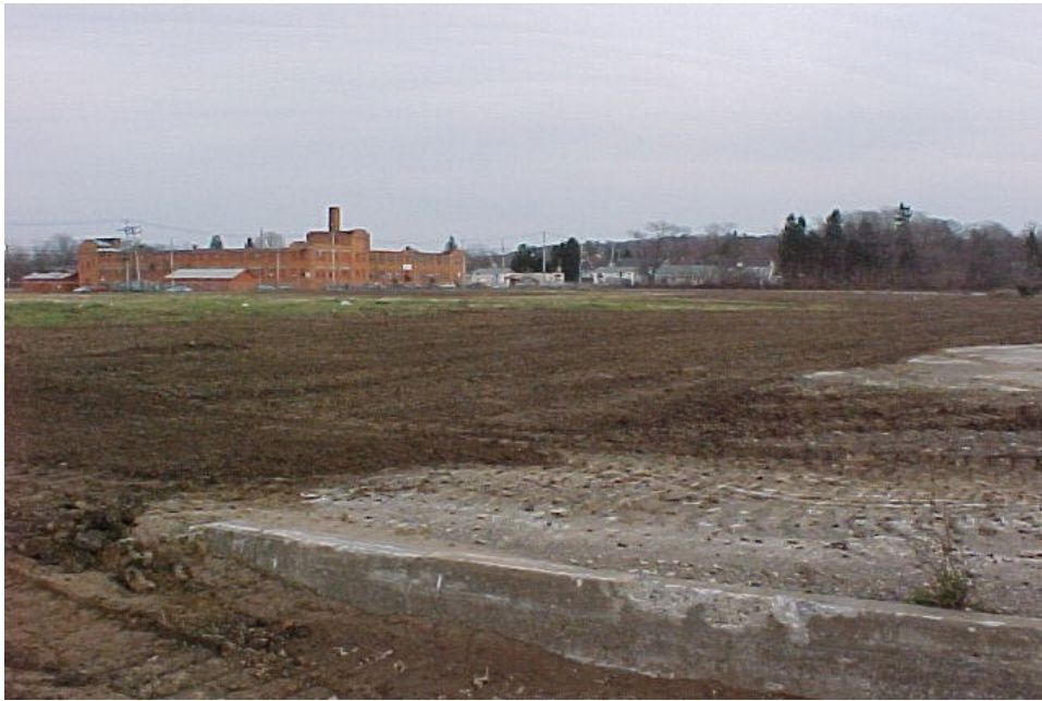
Barrier Layer Construction Activities Completed Looking northeast from Parking Lot No. 2 on 11/21/05
