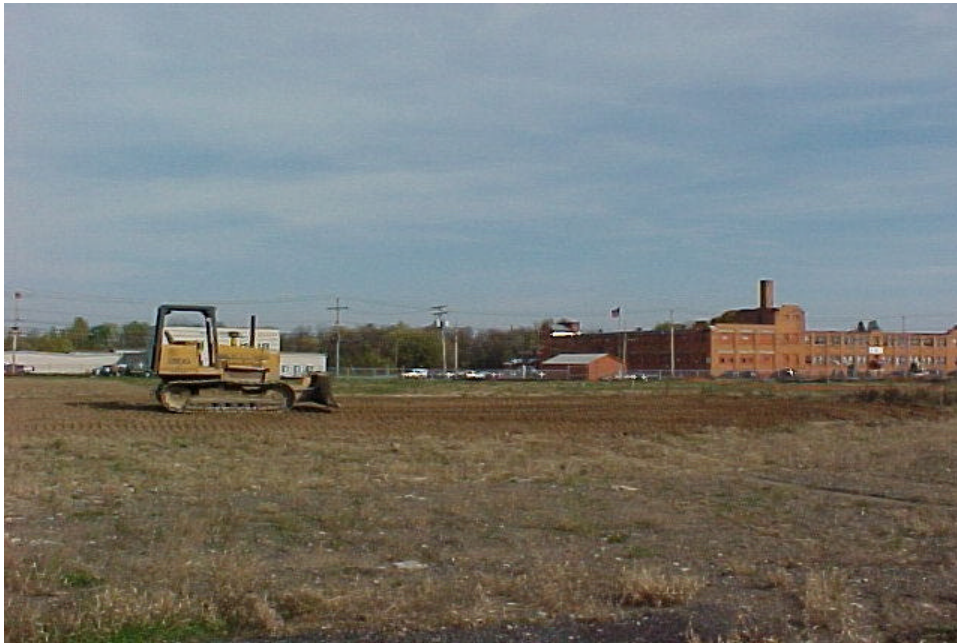
Placement of 9-Inch Minimum-Thickness Run-of-Bank Gravel Layer Looking north from Parking Lot No. 2 on 11/1/05
