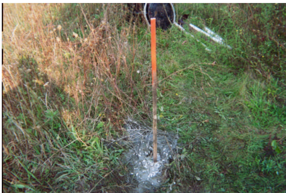
Modification and Decommissioning of Monitoring Wells Looking north from Former Test Building location on 9/13/05
