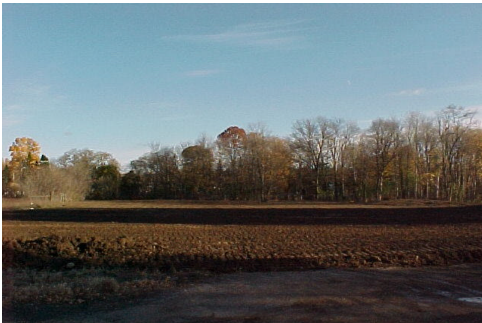
Barrier Layer Construction Activities Completed Looking east from Parking Lot No. 2 on 11/8/05
