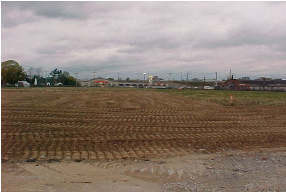
Placement of 9-Inch Minimum-Thickness Run-of-Bank Gravel Layer Looking west from Parking Lot No. 1 on 11/1/05
