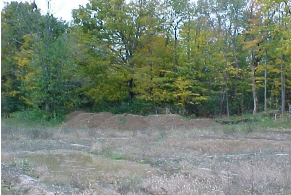
Placement/Grading/Compaction of Run-of-Bank Gravel to Fill Depressions Looking east from Parking Lot No. 2 on 10/26/05
