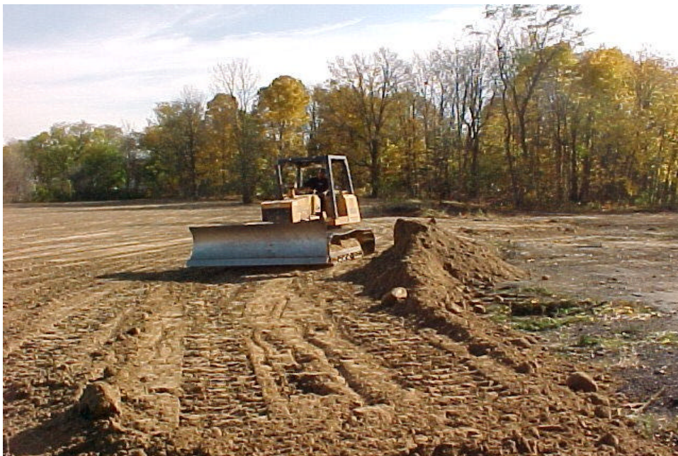
Placement of 9-Inch Minimum-Thickness Run-of-Bank Gravel Layer Looking east from Parking Lot No. 2 on 11/3/05
