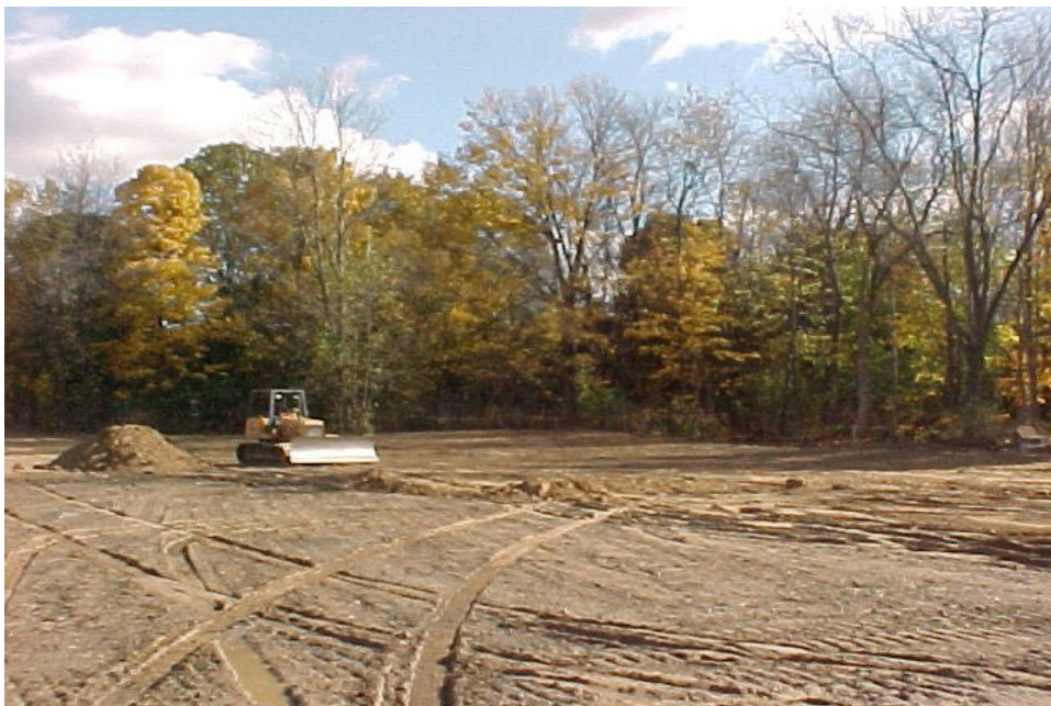
Placement of 9-Inch Minimum-Thickness Run-of-Bank Gravel Layer Looking east from Parking Lot No. 2 on 11/2/05
