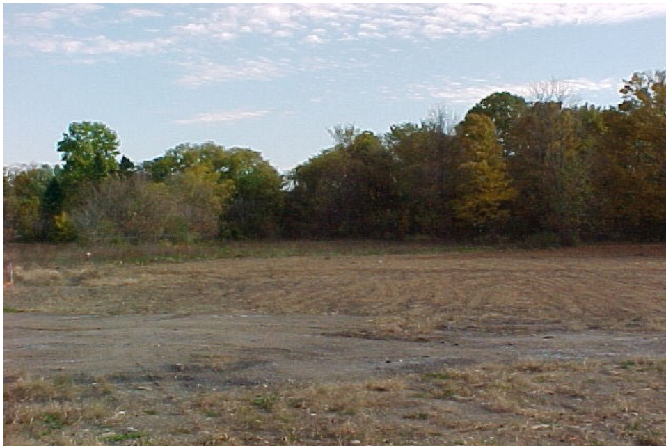
Placement/Grading/Compaction of Run-of-Bank Gravel to Fill Depressions Looking east from Parking Lot No. 2 on 10/31/05
