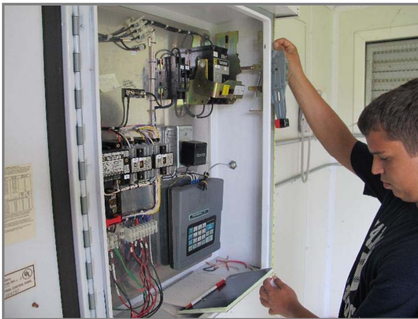
Frank measured the panel enclosure to be 25" wide, 30" tall and 8" deep. The panel contents will all be changed. We will replace the relays with a PLC.
