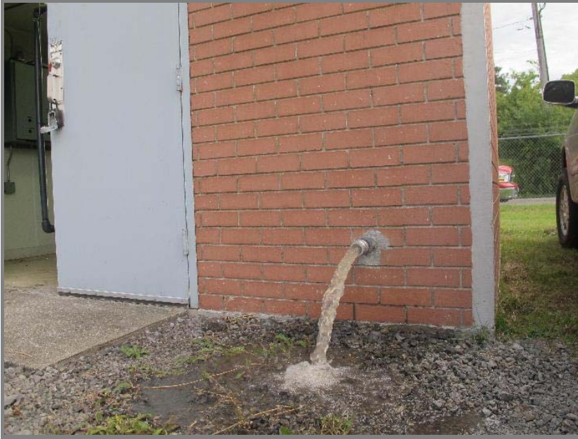
Photo, August 23 - 25, 2011, panel wiring work
