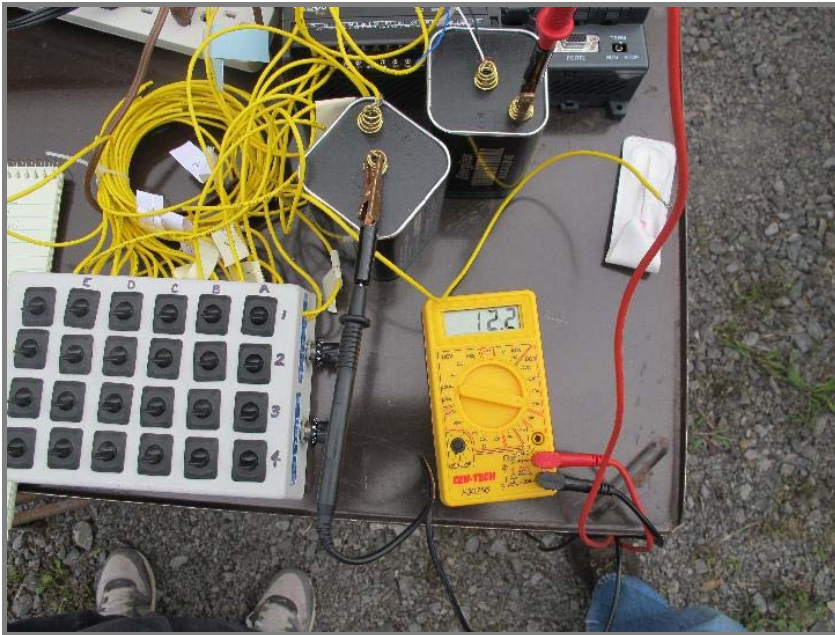
Photo, August 23 - 25, 2011, panel wiring work
