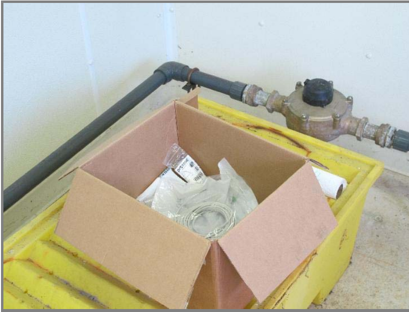
Photo, August 23 - 25, 2011, panel wiring work
