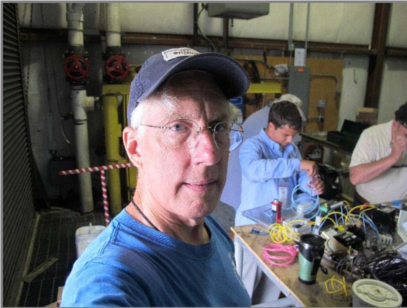
Photo, August 23 - 25, 2011, panel wiring work
