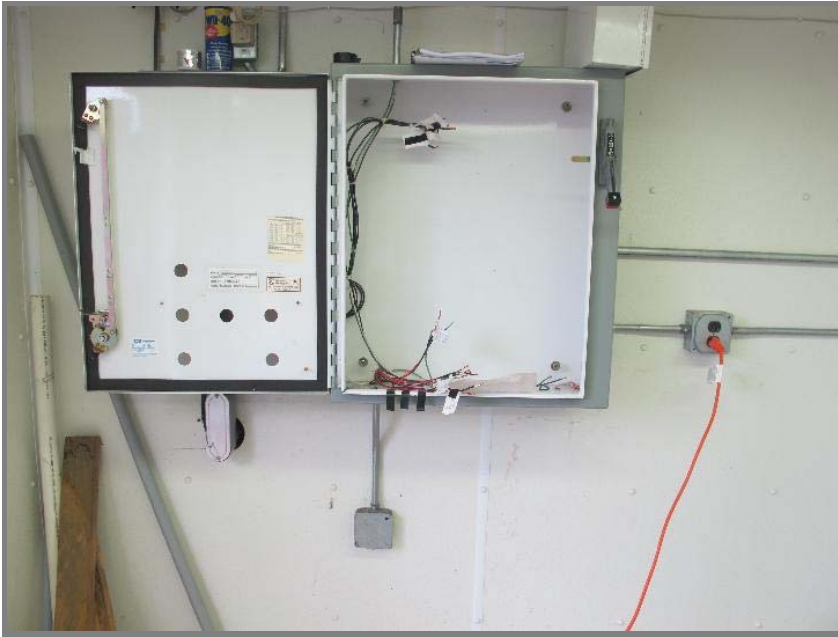
Photo, August 23 - 25, 2011, panel wiring work
