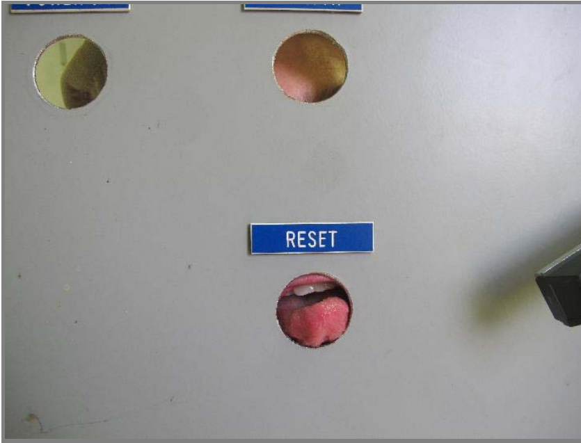
Photo, August 23 - 25, 2011, panel wiring work
