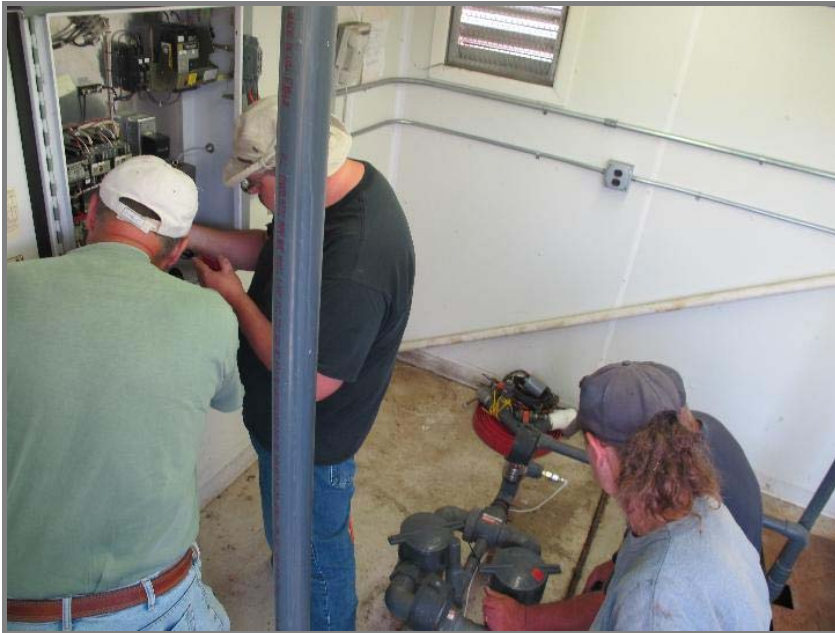
Photo, August 23 - 25, 2011, panel wiring work
