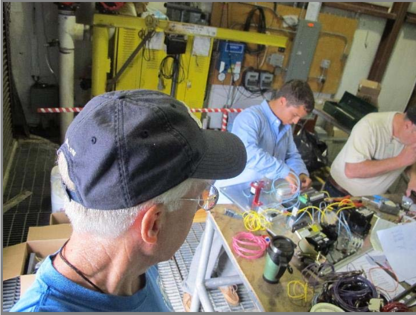
Photo, August 23 - 25, 2011, panel wiring work
