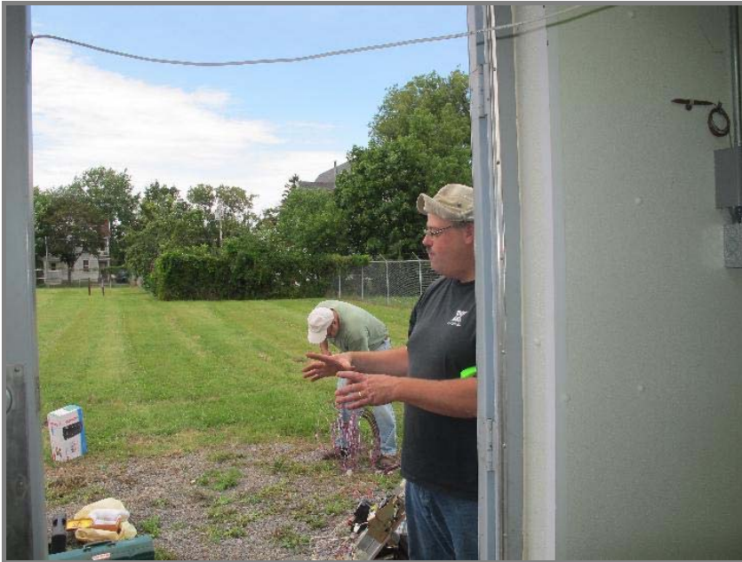
Photo, August 23 - 25, 2011, panel wiring work
