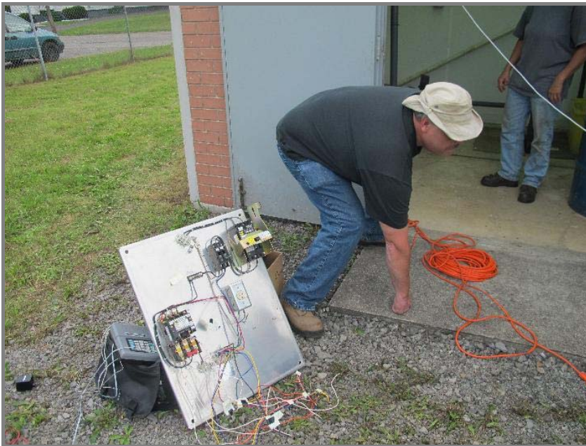
Photo, August 23 - 25, 2011, panel wiring work
