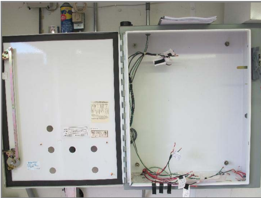
Photo, August 23 - 25, 2011, panel wiring work
