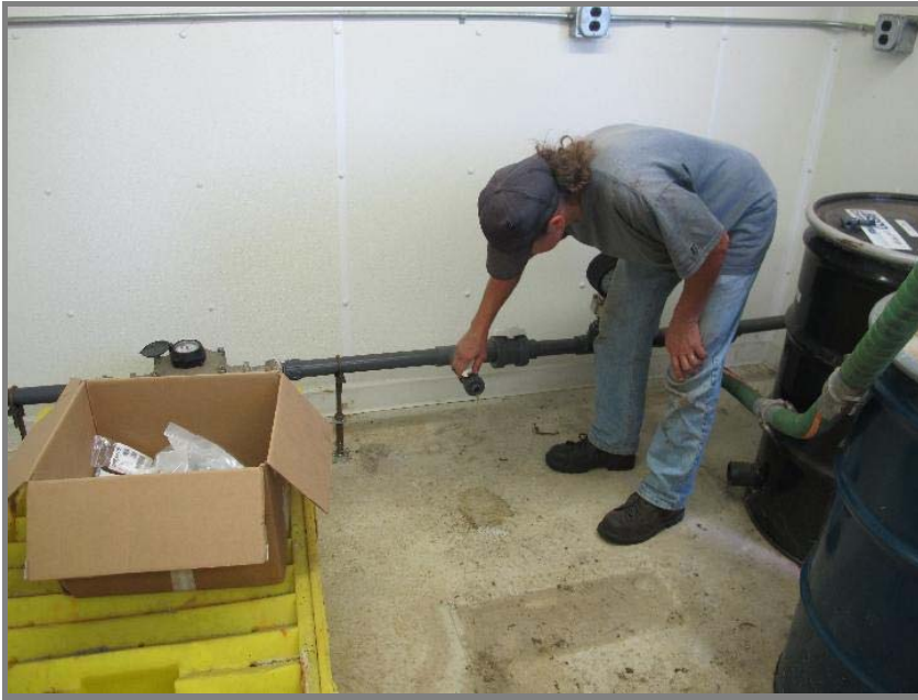
Photo, August 23 - 25, 2011, panel wiring work
