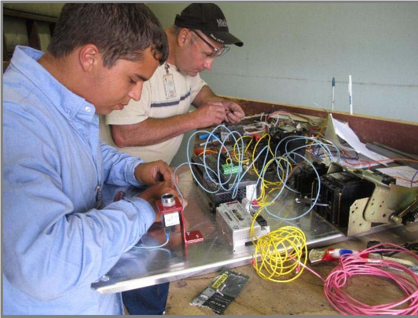
Photo, August 23 - 25, 2011, panel wiring work
