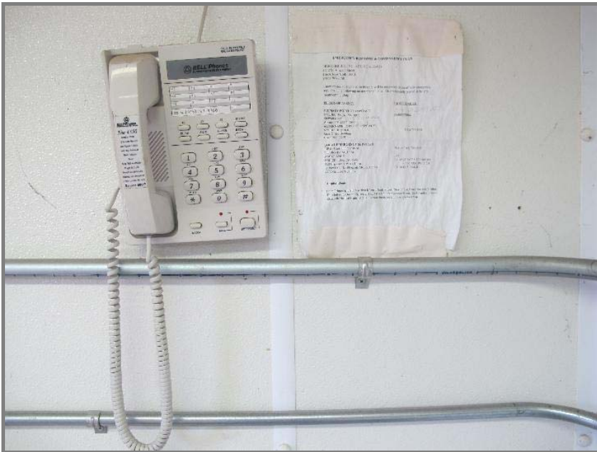
Photo, August 23 - 25, 2011, panel wiring work
