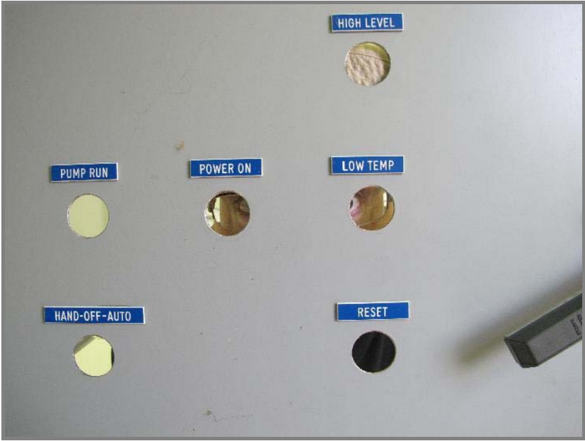
Photo, August 23 - 25, 2011, panel wiring work
