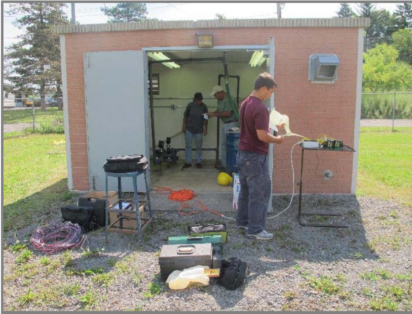
Photo, August 23 - 25, 2011, panel wiring work
