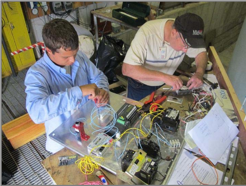
Photo, August 23 - 25, 2011, panel wiring work
