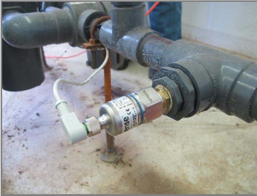
Photo, August 23 - 25, 2011, panel wiring work
