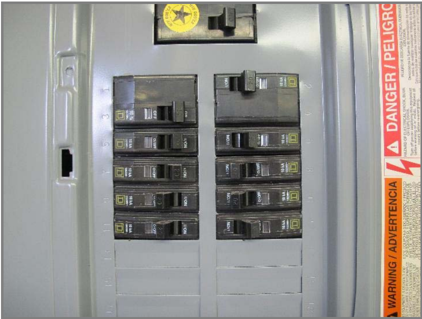
Photo, August 23 - 25, 2011, panel wiring work
