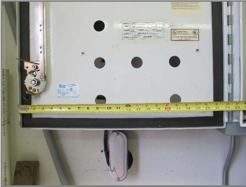
Photo, August 23 - 25, 2011, panel wiring work
