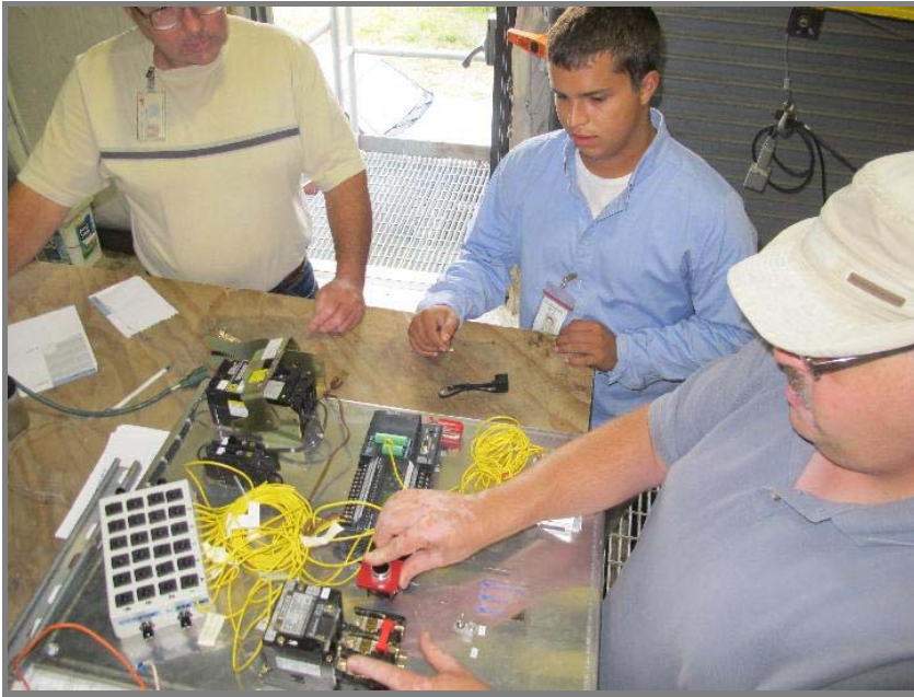
Photo, August 23 - 25, 2011, panel wiring work
