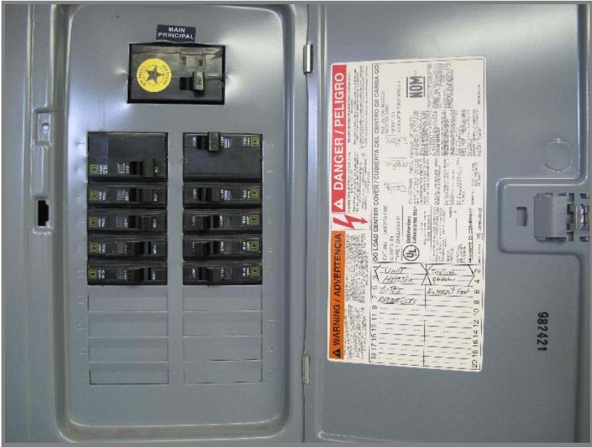
Photo, August 23 - 25, 2011, panel wiring work
