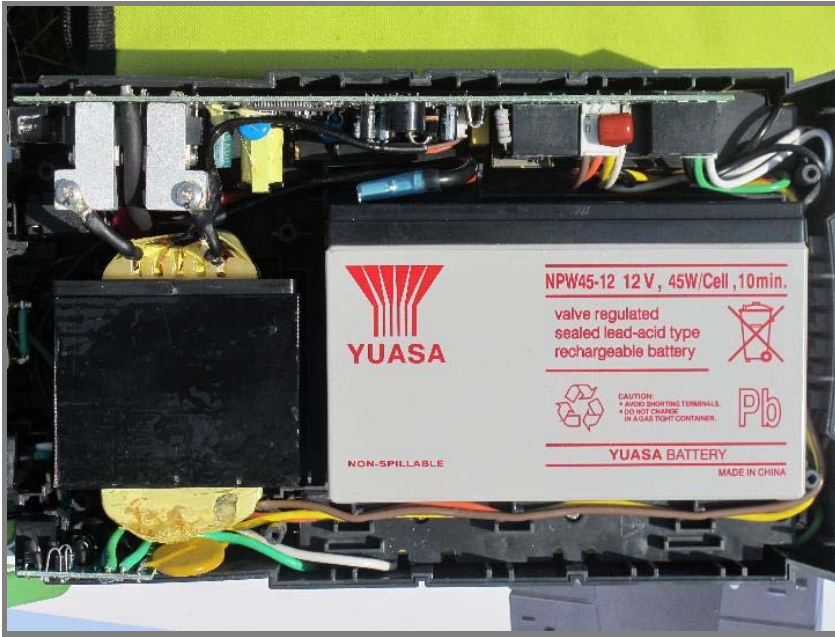
Photo, August 23 - 25, 2011, panel wiring work
