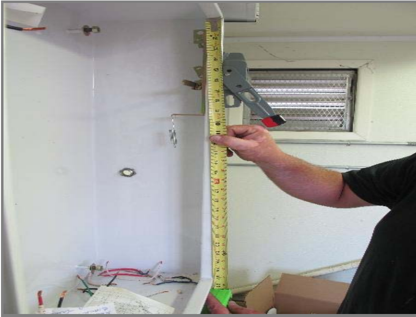
Photo, August 23 - 25, 2011, panel wiring work
