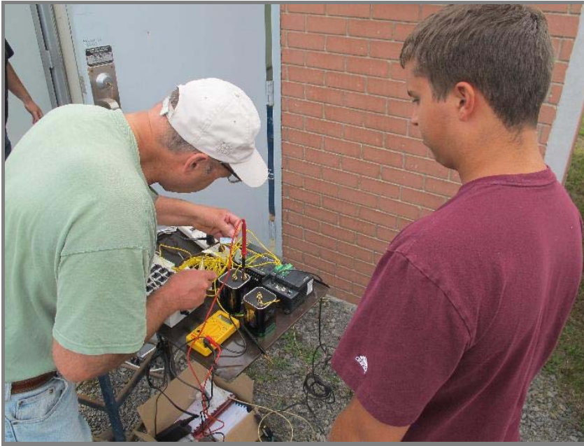
Photo, August 23 - 25, 2011, panel wiring work
