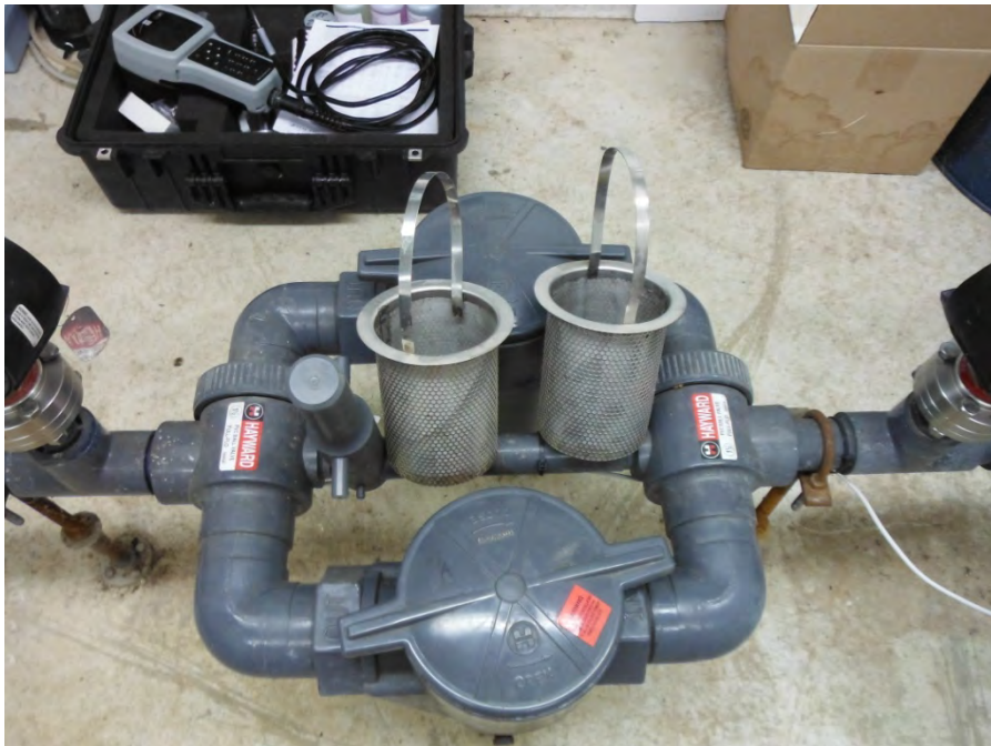
Photo 6: Basket strainers from the Treatment system
