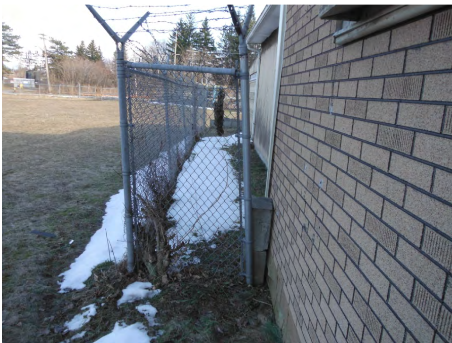
Photo 20: Loose fence post against building and southern perimeter of site (repair pending)
