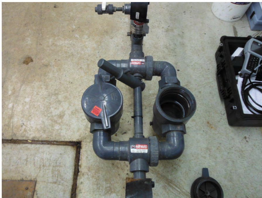
Photo 7: View of holders for the basket strainers
