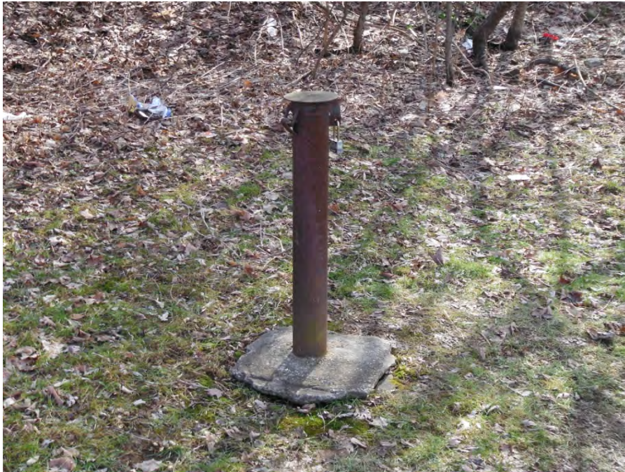
Photo 5: Monitoring Well P-108 slight heaving of concrete pad (view 2)
