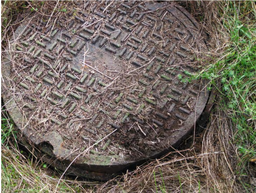
9. Cracked iron collar at MH-13
