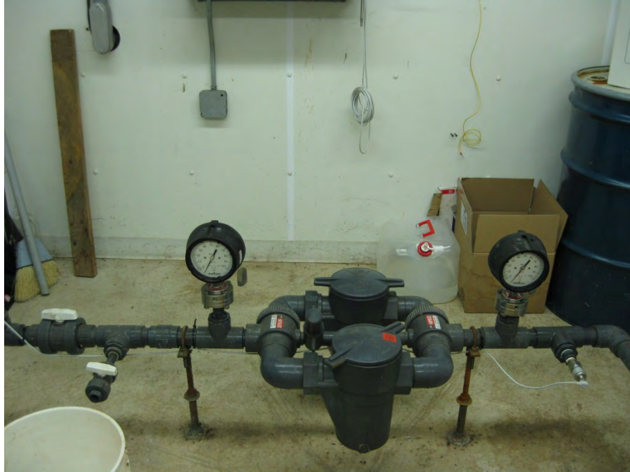
Photo 3 – System piping; pressure sensor next to gauge at right, sample port is next to gauge on left, basket strainers in the center. Looking northeast inside treatment building
