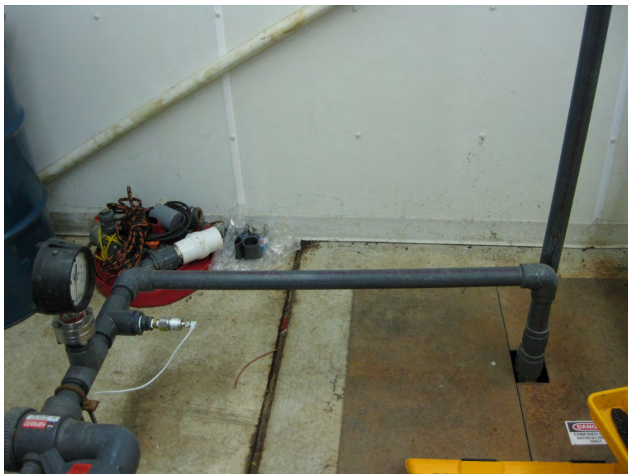
Photo 2 – Start of system piping (influent) Looking southeast inside treatment building
