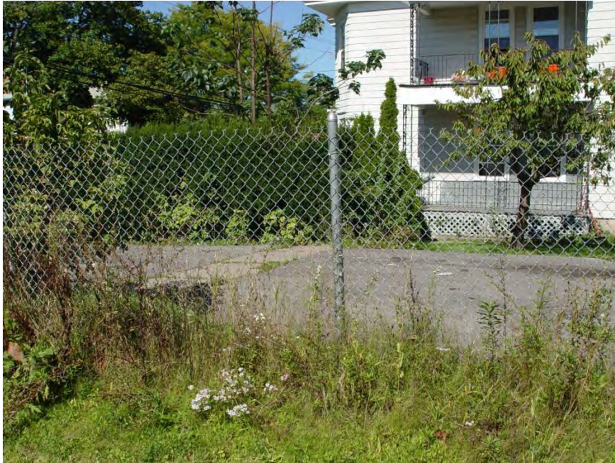
Photo 11: Missing top rail and barbed wire - northwest
