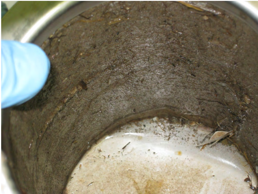
Photo 19 – Close up of basket strainer removed from housing; fine silts and some organic debris visible.
