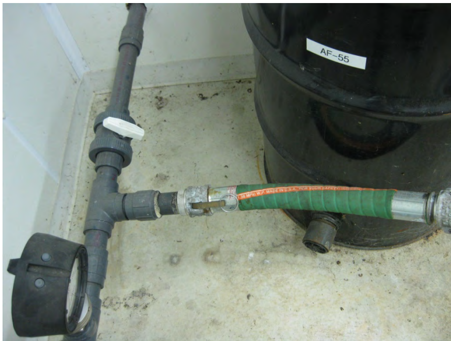
Photo 9 – System piping, flex hose connection back to hard pipe
