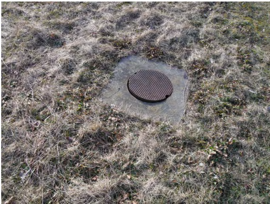
Photo 14: Slightly heaved cleanout cap near P-106S/D
