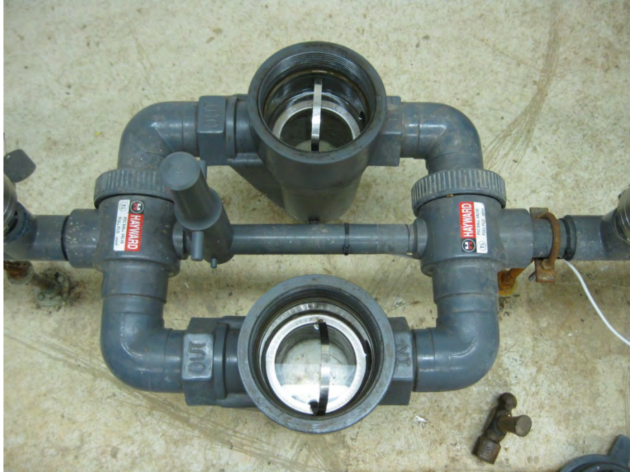
Photo 18 – looking down on basket strainers, covers off; treatment building
