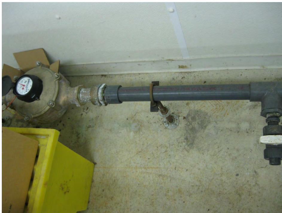
Photo 11 – System piping, left is totalizer and at the right a sample port
