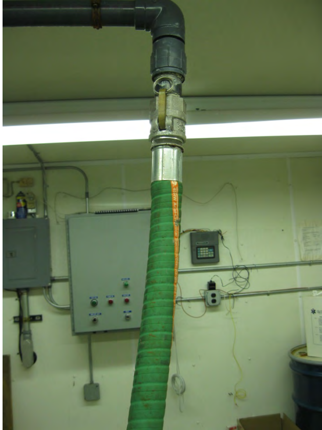
Photo 7 – System piping, showing connection from hard Pipe to flex hose; looking north inside treatment building
