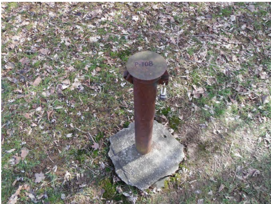
Photo 4: Monitoring Well P-108 slight heaving of concrete pad (view 1)
