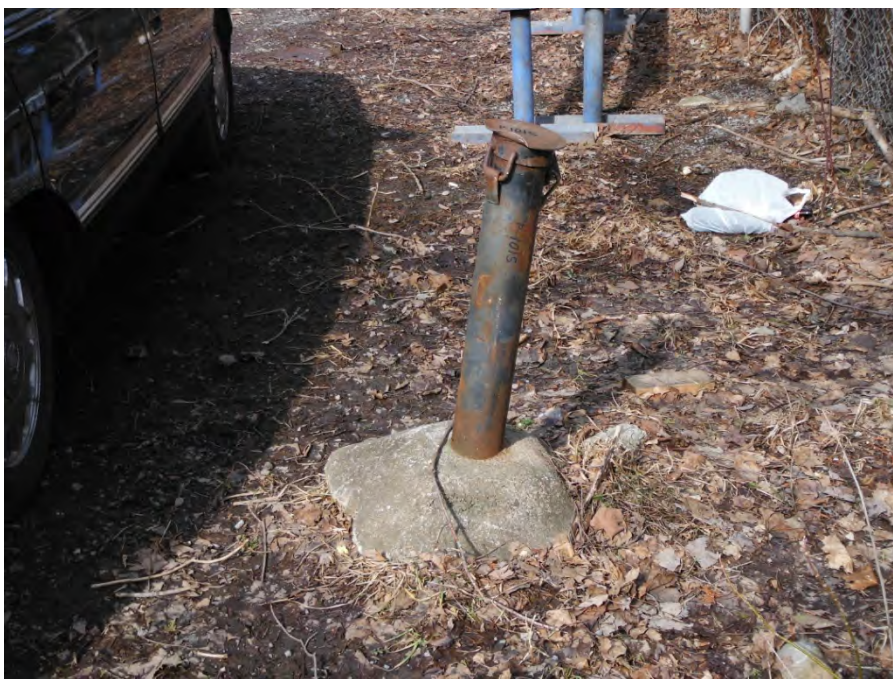
Photo 1: Monitoring Well P101S damage view
