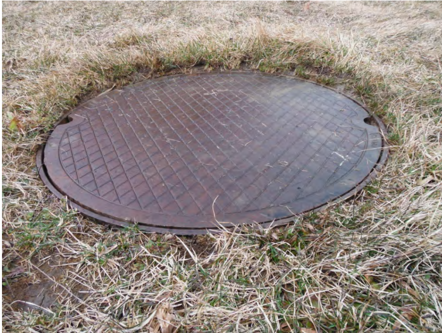
Photo 25: Collection manhole cover
