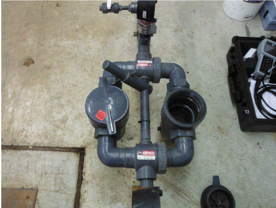
Photo 7: View of holders for the basket strainers
